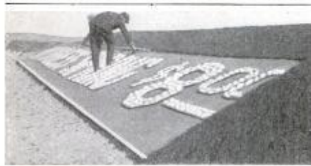
Large Sign of Concrete and Clamshells: These Materials were Selected for the Purpose of Reducing the Upkeep Cost of the Sign
