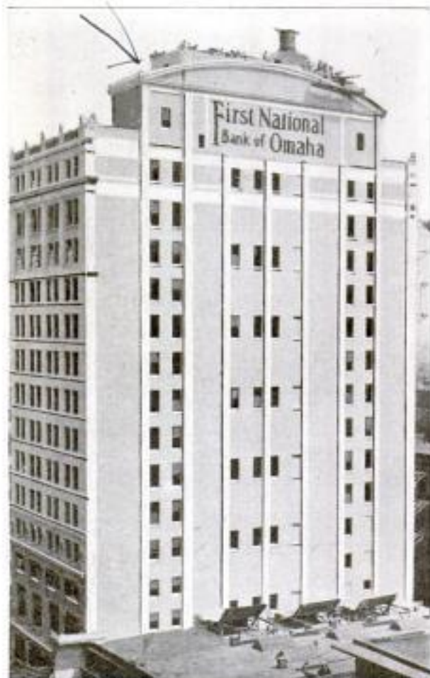
A Conspicuous Sign Which is Made of Terra Cotta: It Measures 14 by 44 Feet and Stands 200 Feet above the Street
