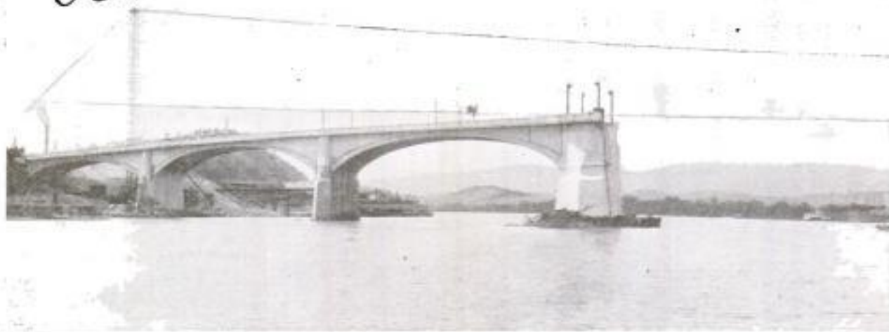
Chattanooga's New 2,500-Foot Reinforced-Concrete Bridge, across the Tennessee River, Which Bascule Span of
