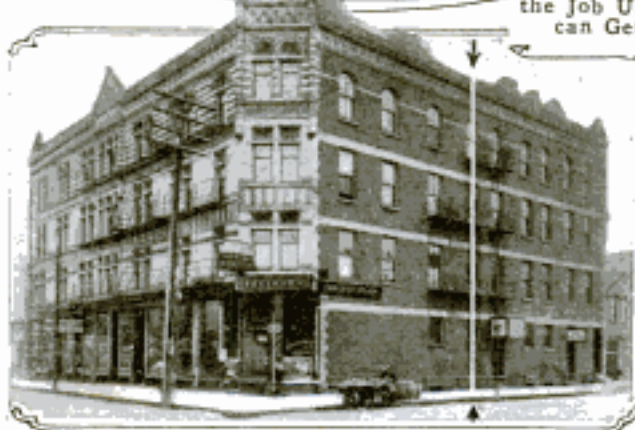
The White Line on the Building at the Left Indicates the Shave It Underwent. This Was a Substantial Four-Story Structure. There Was Not Room to Move It Back, So Part of the Building had to be Sacrificed
