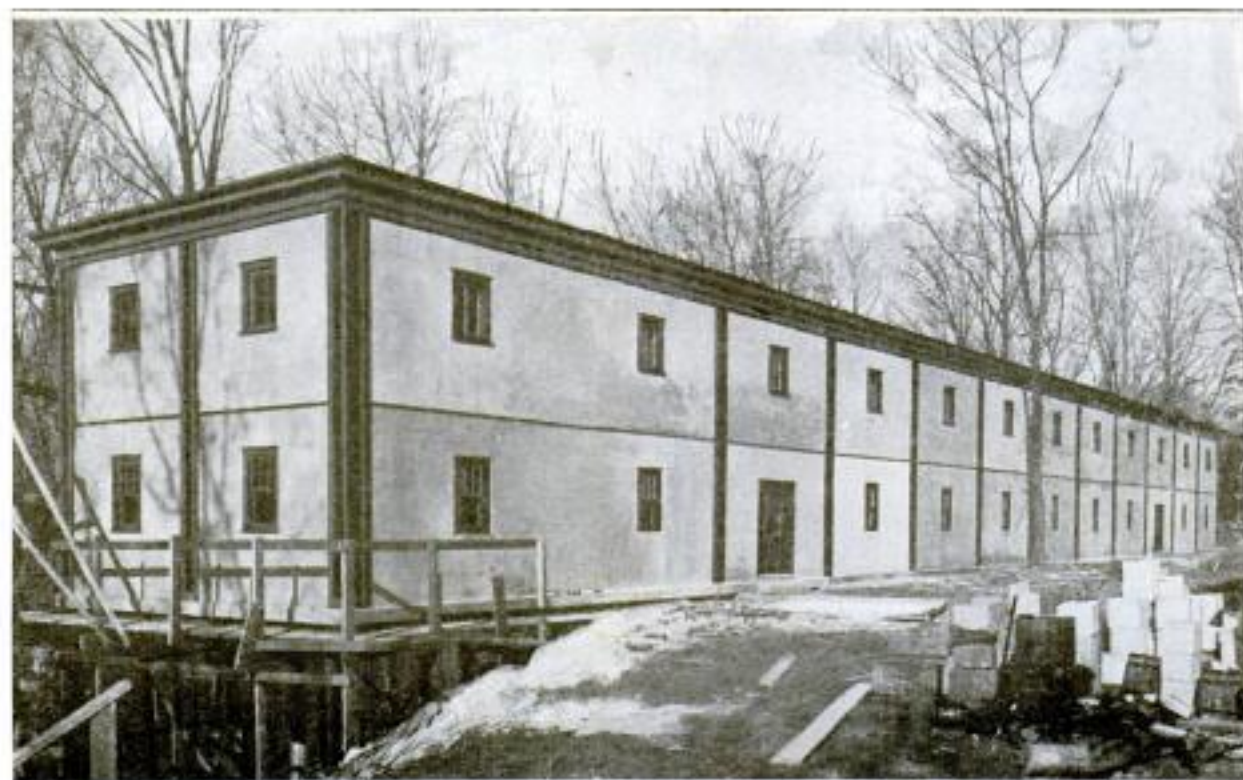
A Structure Having 56 Stucco Panels, No Two of Which Are Exactly Alike. Built for the Purpose of Testing Various Kinds of Stucco and the Bases to Which It is Applied
