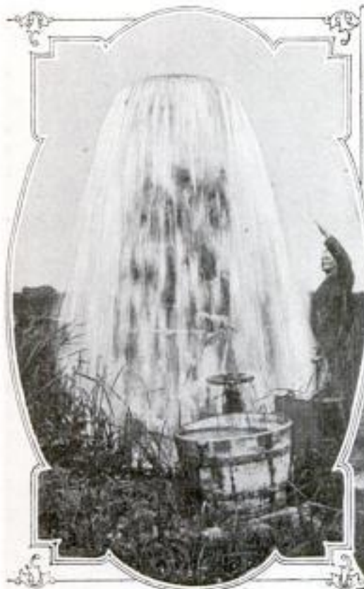
Several Wells Which Barely Bubbled Before, Flowed Like This After the Water Was Spread
