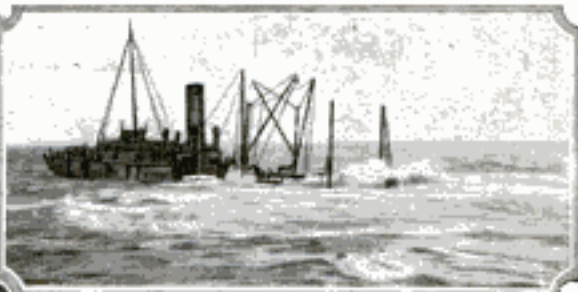
Storm Waves, Washing over the Wreck, Repeatedly Spoiled the Work of the Salvors and Drove Them Away
