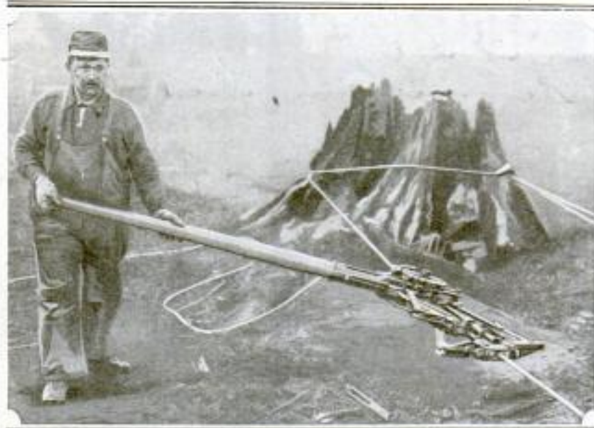
The Device Attached to Block Cable, Which is Anchored to Stump at Right. Stump to be Pulled Not Shown in Picture
