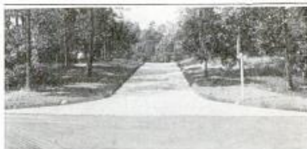
Newly Laid Concrete Paving in a Residence District in Cedar Rapids, Iowa, Which Slopes toward the Center and Requires No Curb
