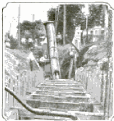
Above: View Showing a Section of the Main being Lowered into the End of the Trench. Left: Crane Lifting a Section Weighing Four and One-Half Tons
