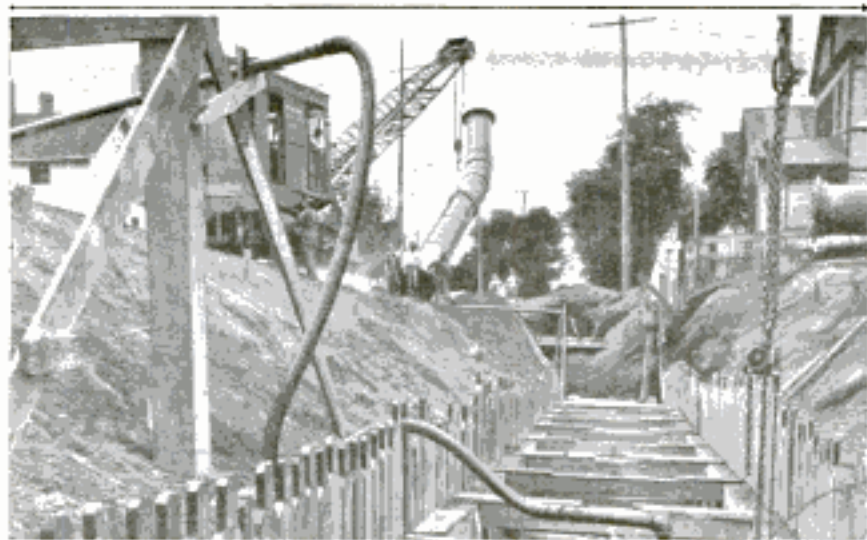
Above: View Showing a Section of the Main being Lowered into the End of the Trench. Left: Crane Lifting a Section Weighing Four and One-Half Tons
