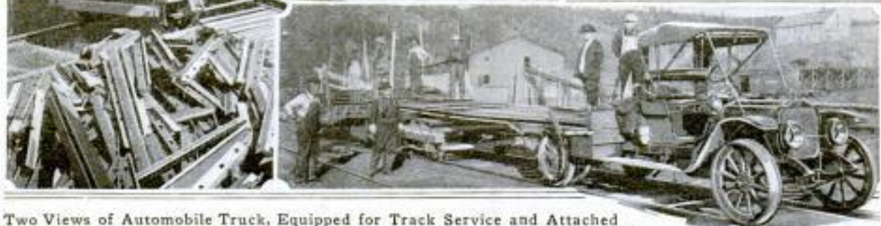
Two Views of Automobile Truck, Equipped for Track Service and Attached to a Trailer: The Outfit was Used to Salvage the Rails on an Abandoned Railway Line and Traveled 108 Miles a Day, Its Loads Being 12 Tons Each
