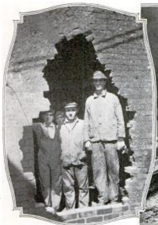
The View on the Left Shows a Big Hole Broken in a Brick Wall by a Section of the Shattered Flywheel. On the Right Is the Interior of the Engine Room after the Accident. The Shaft Which Drove the 30-Ton Wheel is Shown Wound with Wire
