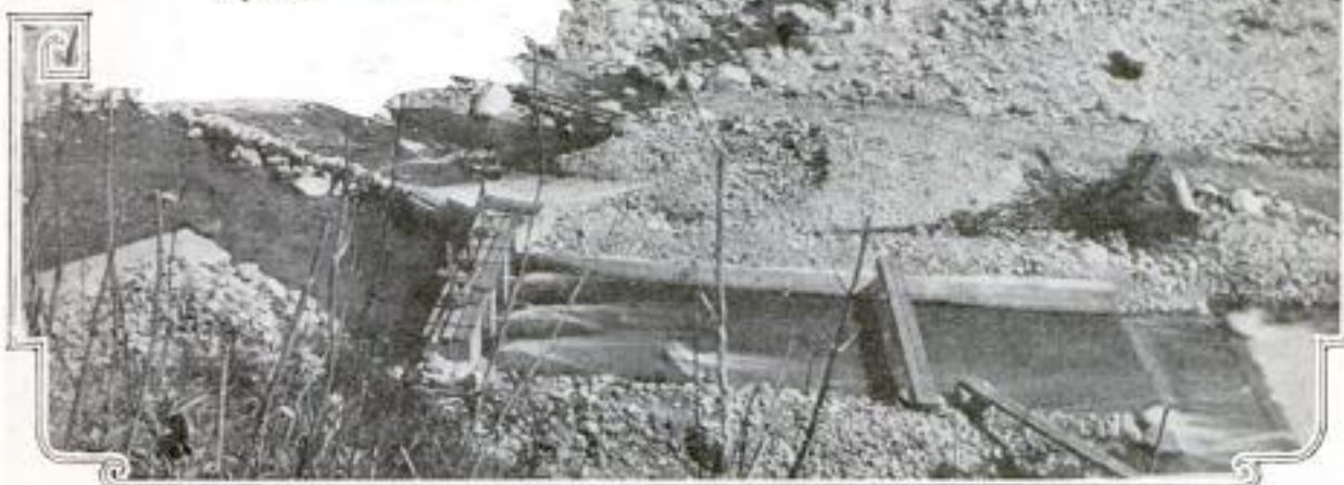
A View of San Antonio Creek Bed, Which is Almost Dry, with Dam in Foreground, Which Diverts Flood Water to the Right. This Rocky Soil is Well Adapted to Absorbing the Water
