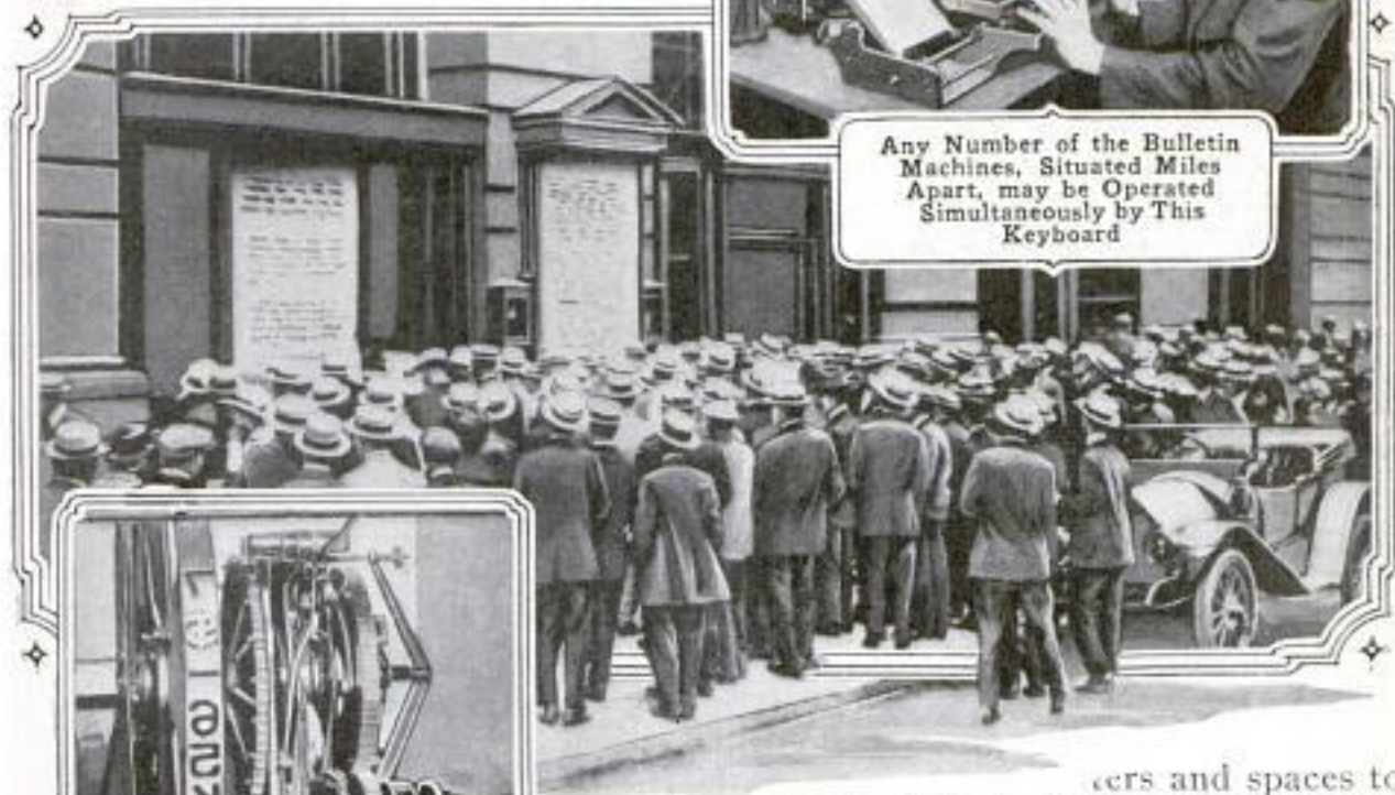
Above: Crowds Blocking Sidewalk before Office of a Philadelphia Newspaper Where the Electric Bulletin-Board System is Installed. Left: The Type Wheel and Operating Mechanism of Apparatus
