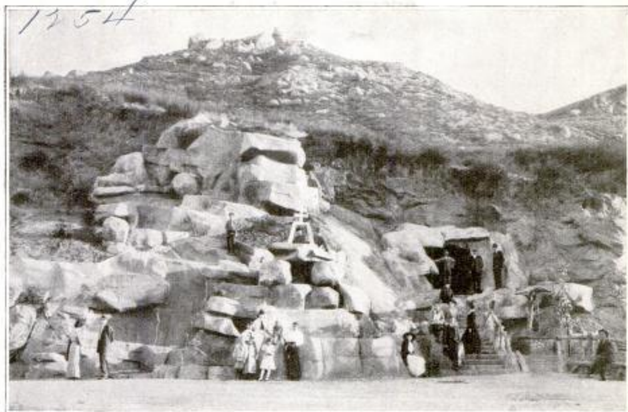
Waterfall and Drinking Fountain of Natural Appearance Built of Concrete
