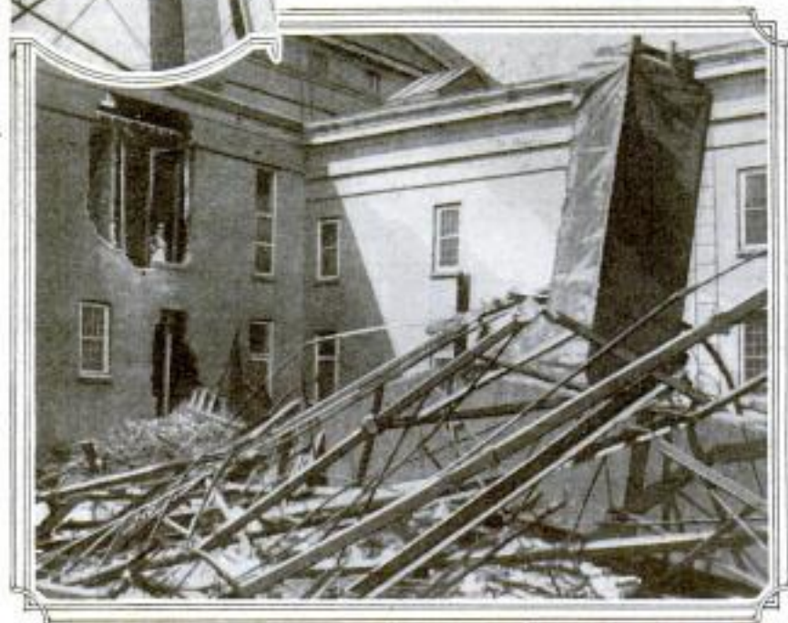
At the Top the Tank is Shown as It Appeared When Ablaze. The Photograph Below was Taken After the Tower had Collapsed, and Pictures Its Debris and the Damage Done by It
