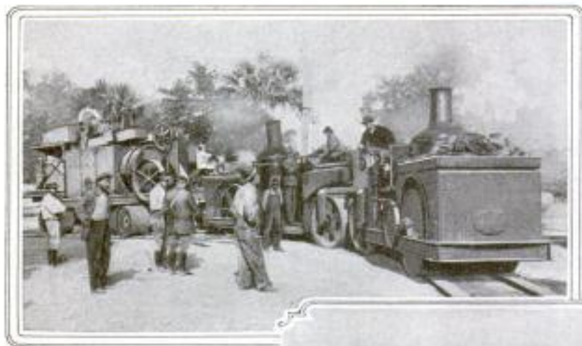
The Road is Given a Clay Base When Possible and Surfaced with a Special Mixture of Asphalt and Sand, Applied Hot and Rolled
