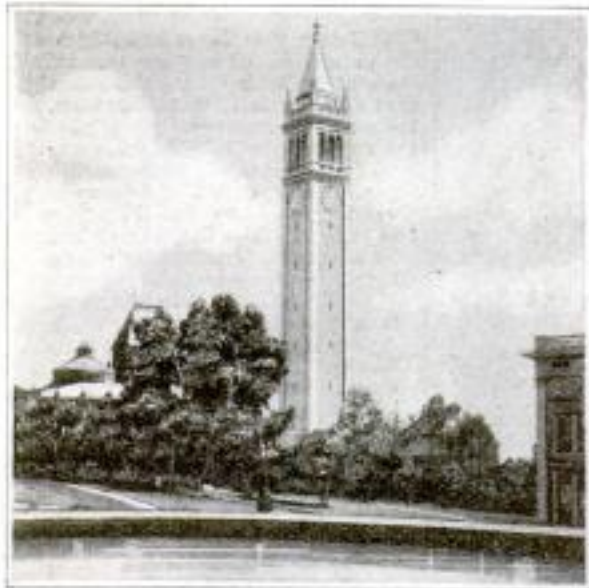
Three-Hundred-Foot Campanile on University of California Campus Built to Resist Earthquakes
