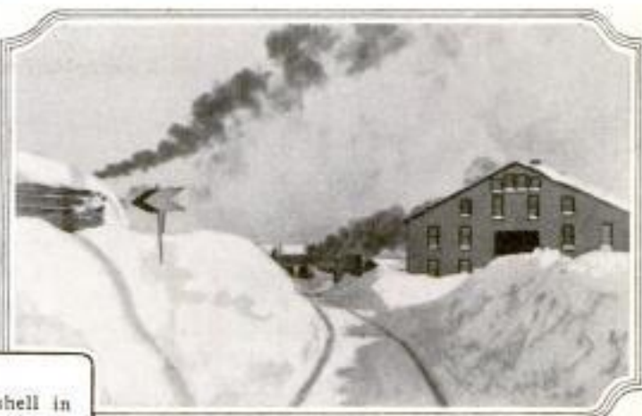
Clamshells were Used in Cutting This Path through Snowdrifts in Northern Michigan
