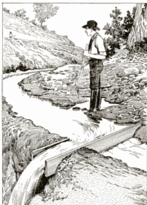
Spillways in Irrigation and Mining Ditches on Hilly Ground Prevent Washouts
