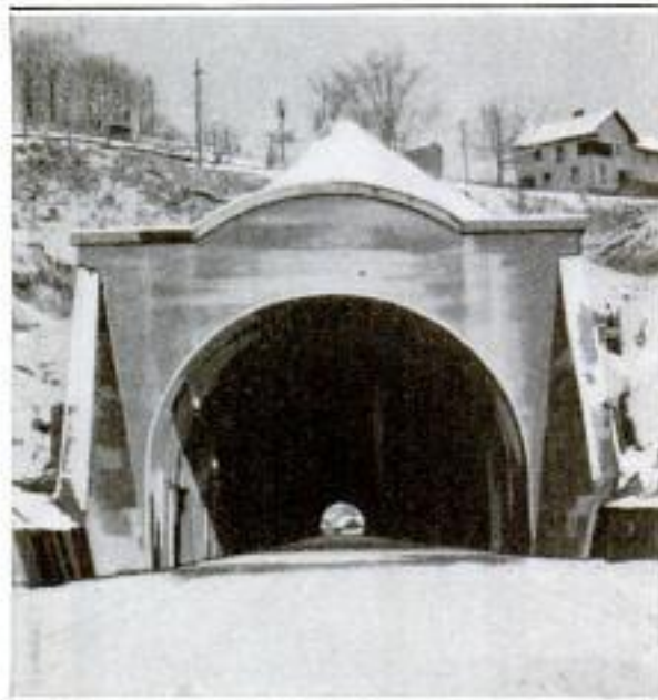
A Highway Tunnel, 933 Feet Long, Which Pierces Historic Missionary Ridge, Three Miles from Chattanooga, Tennessee
