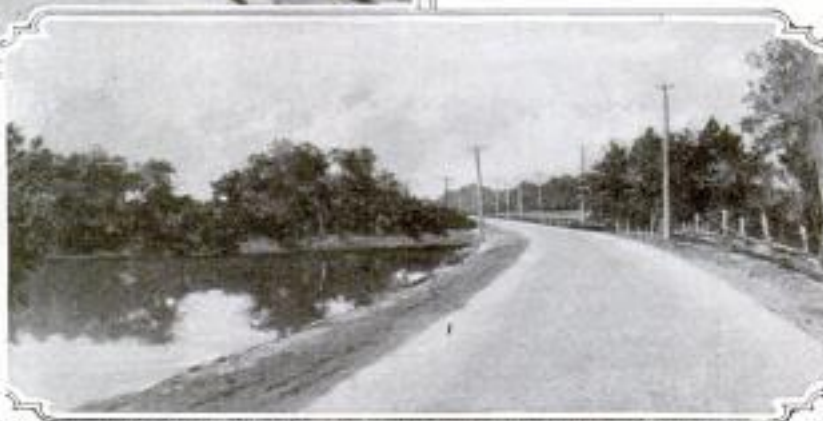
Stretch of Sand-Asphalt Turnpike Extending through Rural District in Florida. This Type of Highway Presents a Good Appearance, but the Length of Its Life Is Yet to be Determined
