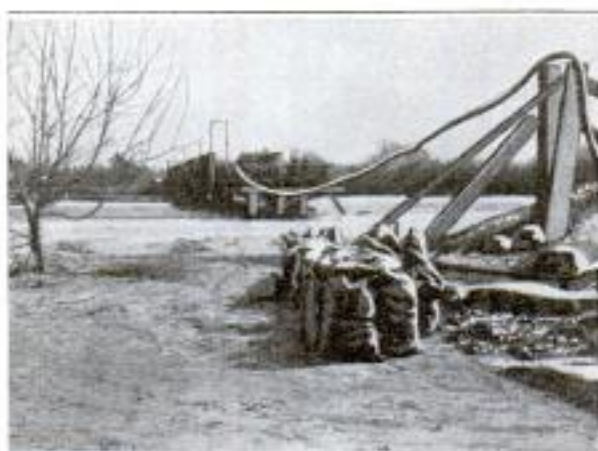
Fire Hose being Used to Bring Gas across a River After the Floods had Carried Away Part of the Bridge and Gas Main
