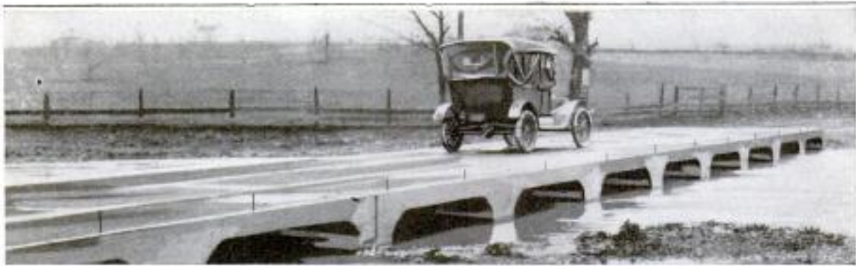
This Concrete Bridge, Which Is so Low as to Require No Approaches, Is 100 Feet Long and 16 Feet Wide, and Cost $750
