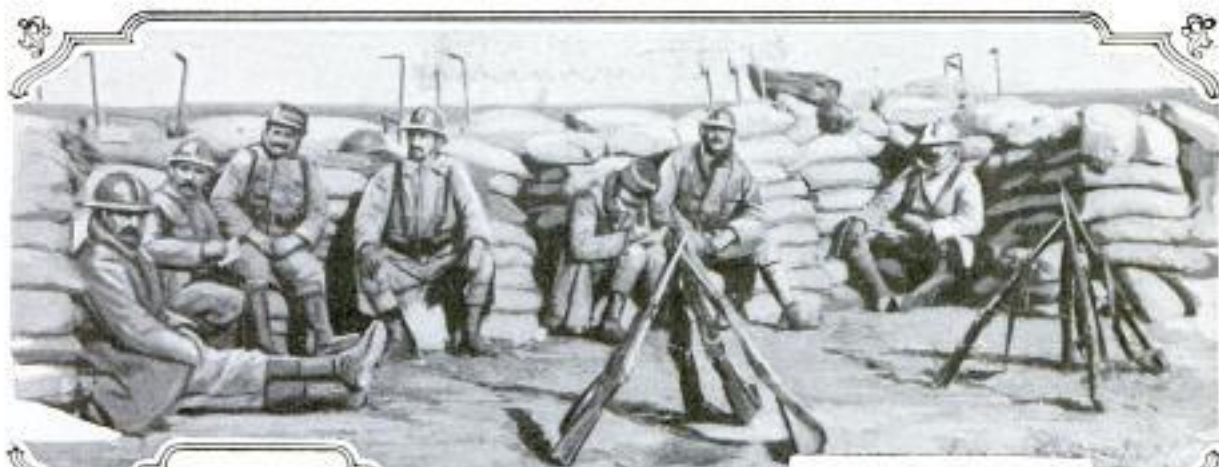
French Troops Intrenched Outside of Saloniki. The Steel Rods Visible above the Parapet are Used to Hold the Bags in Place
