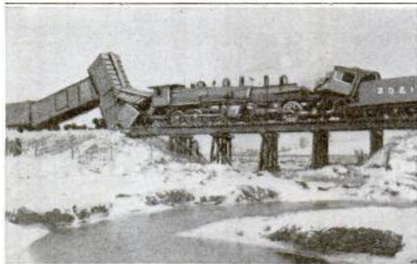
Two Engines as They Appeared Immediately After They had Collided near the Center of a Small Bridge: The Freight Train was Backing onto a Siding to Make Way for the Other, a Fast Milk Train
