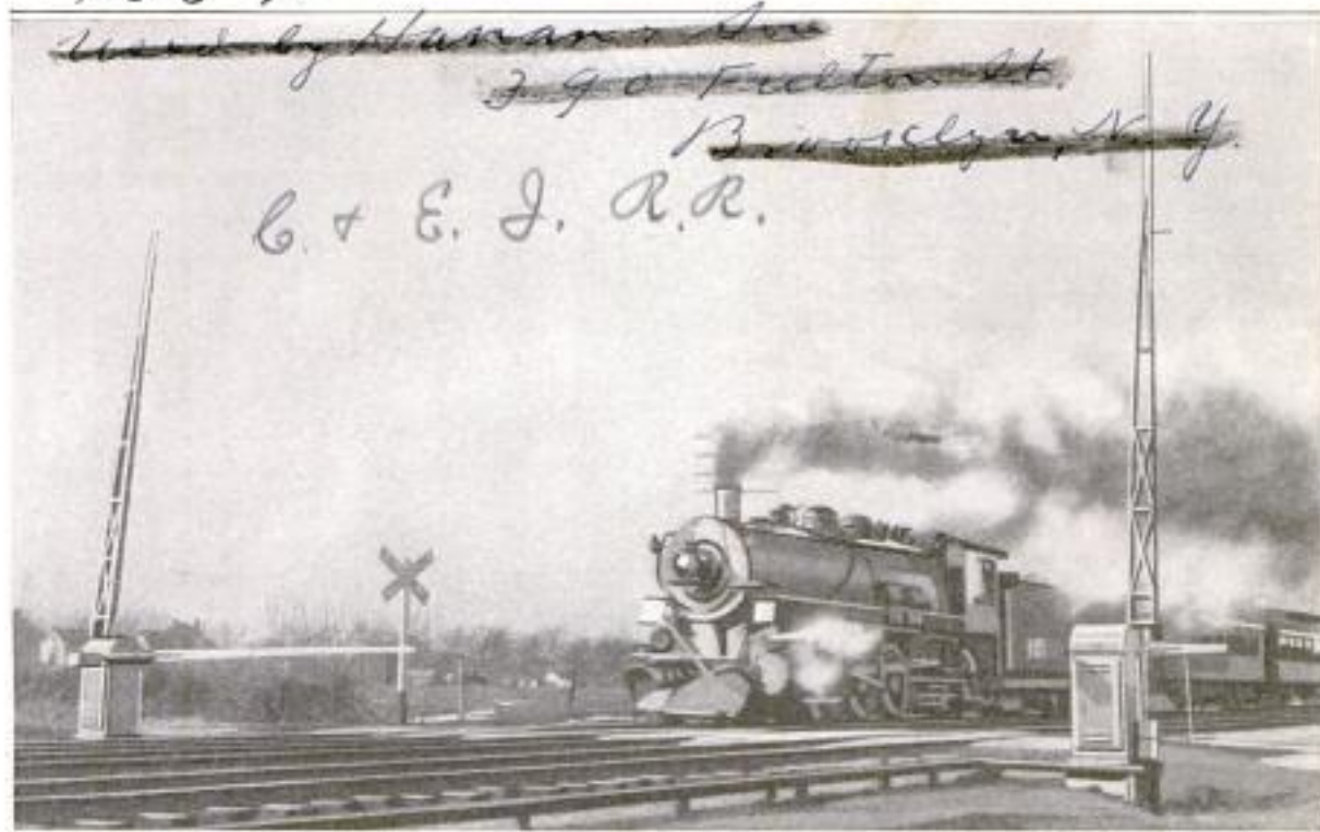
These Automatic Gates are Designed to Guard Users of the Crossing against Switching Operations and against Approaching Trains or Trains Passing in Opposite Directions
