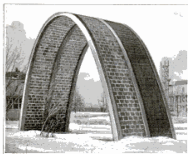
Section of Experimental Arched Roof Made of Clay Blocks
