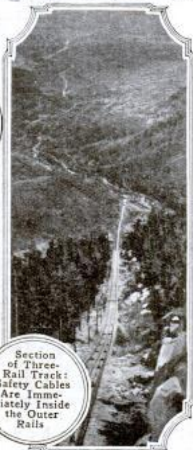
The Line Is Little More than a Mile Long but Makes a Rise of 2,600 Feet
