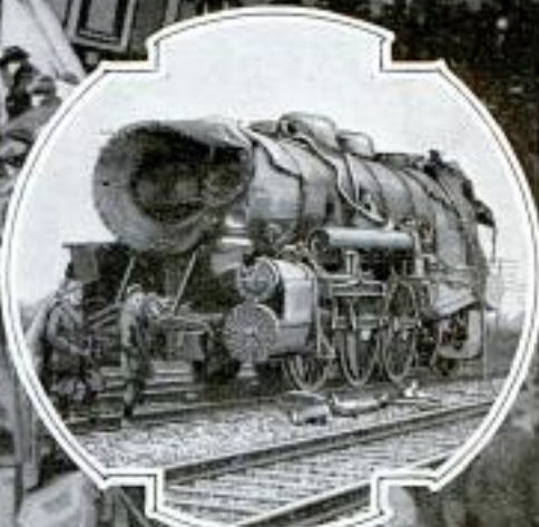
The Tragedy Occurred When the Second Section of a Two-Part Train Smashed into the Rear of the First, Pushing Some of the Wreckage across Another Track in Path of Twentieth-Century Limited, the Engine of Which is Shown Above
