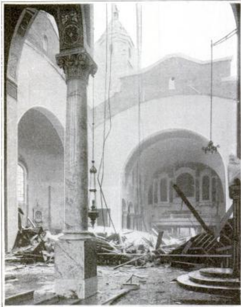
Interior of St. James Cathedral at Seattle After Dome had Collapsed under the Weight of Wet Snow
