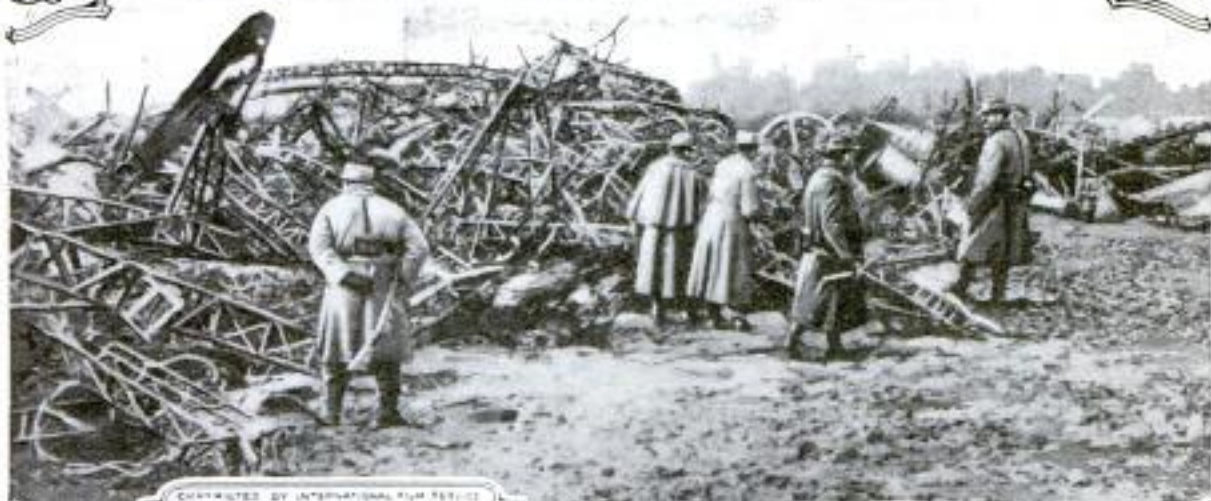
CONTRIBUTED BY INTERNATIONAL FILM SERVICE Wreckage of Zeppelin "L 77," Which was Recently Brought Down near Brabant-le-Roi by an Incendiary Shell
