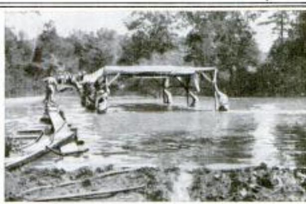
Carrying a Shelter across a River to a Point Where the Workers are Concentrated
