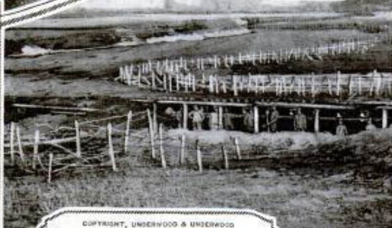
Network of Entanglements Protecting Austrian Position in Swamp, Where It Was Necessary to Build the Trenches on Top of the Ground
