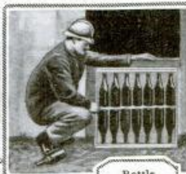
Bottle Window Used in French Dugouts Resists Concussion of Big Shells
