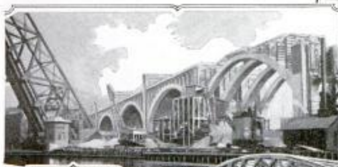
From Structure in Foreground It may be Seen That Each Span Is in Reality a Quadruple Arch
