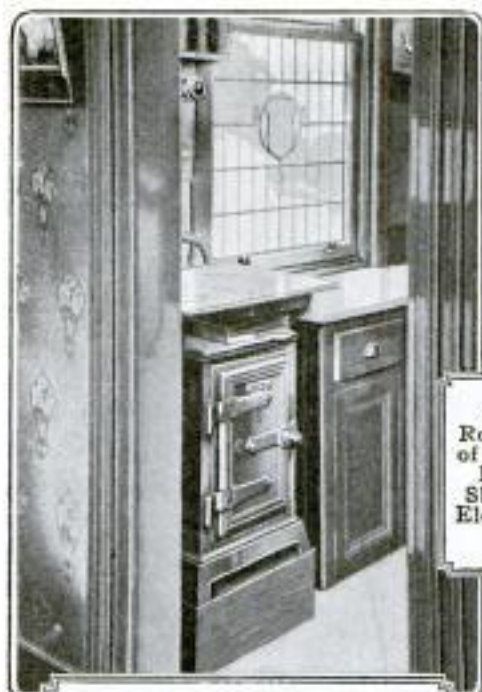
The Compact Electric Kitchen Range with Double Heat-Retaining Walls, Used in One of the "Electric" Bungalows
