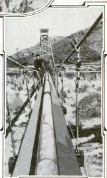
A Near View of the Pipe Line and a Suspension Bridge Which Carries It over a River Bed
