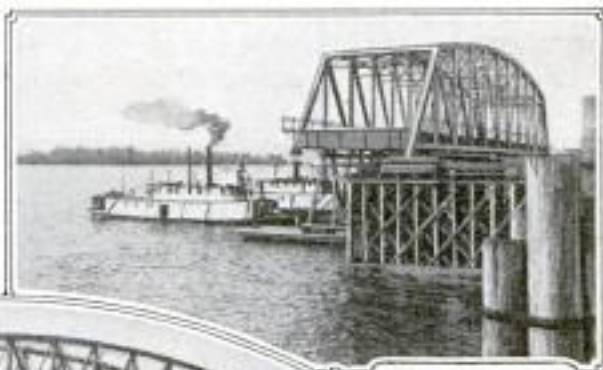
One of the Spans, being Drawn by Two Tugs, Leaving the Special Docks Where Each Span was Constructed
