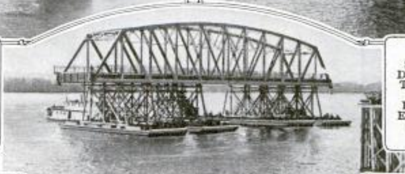
Floating a Section of the Interstate Bridge on the Columbia River
