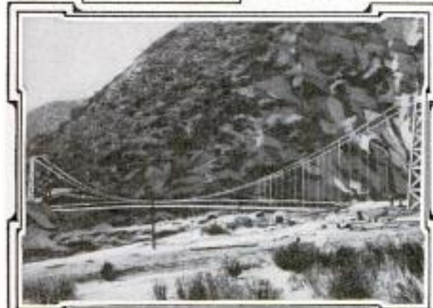
A Suspension Bridge, 500 Feet Long, Built for the Pipe Line in a Region Where Bridges Are Few
