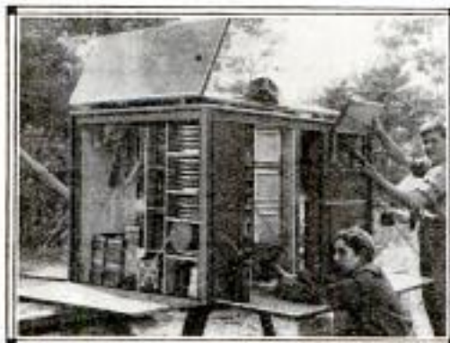
The Portable Kitchen Outfit Opened, Exposing the Various Compartments Arranged So as to Be Convenient: Above, Stove and Cooking Compartments; Below, Pantry Compartment and Space for Utensils
