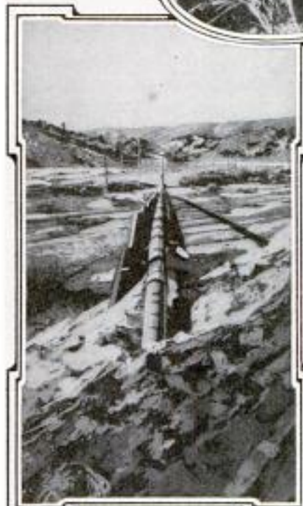
The Pipe Line Projecting from a Hillside and Extending across the Desert, Supported in Part by Framework
