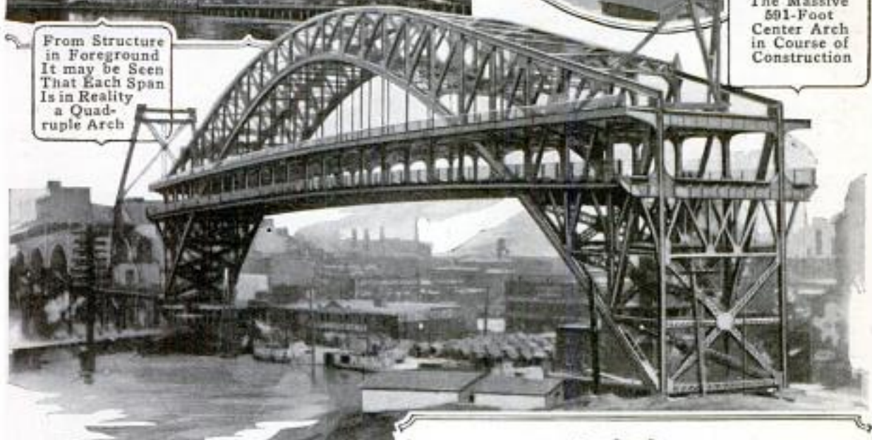
Great Steel Arch After It had been Completed and the Two Decks Suspended from It
