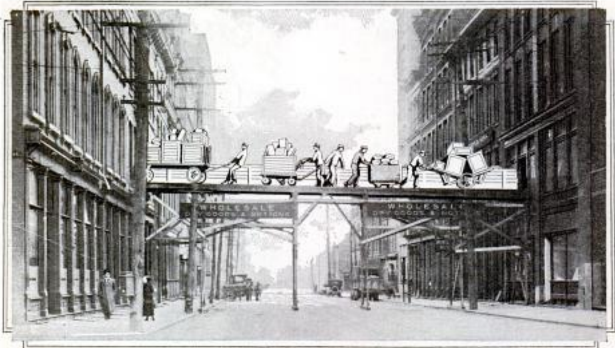
The Stock of Goods was Moved across the Street from One Building into the Other on Trucks Operated on the Temporary Bridge
