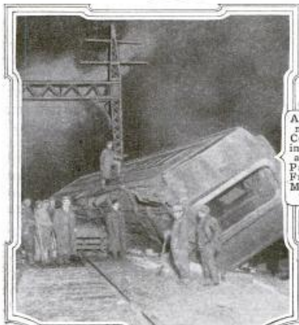
Except for the Overhead Signal Structure, the Car in Foreground would have Followed Others down 50-Foot Embankment
