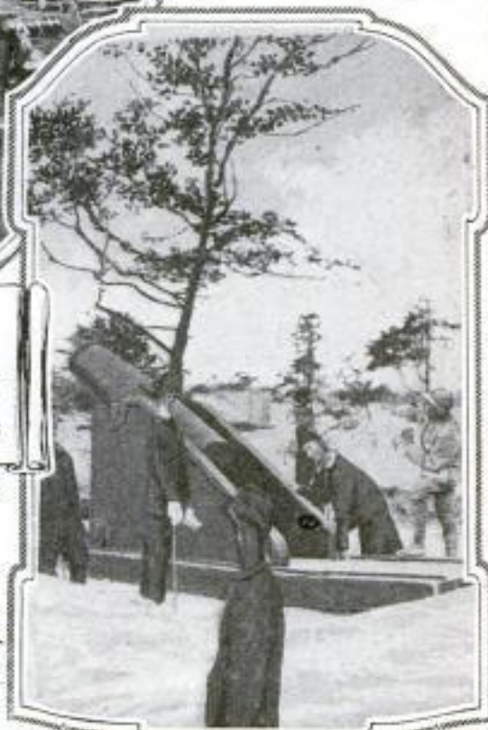
Wooden Mortar and Dummy Artillery- men Divert Airmen from Real Battery: By Pulling Cords Distant Soldier Moves Figures and Causes Smoke to Issue from Gun on Approach of Scout
