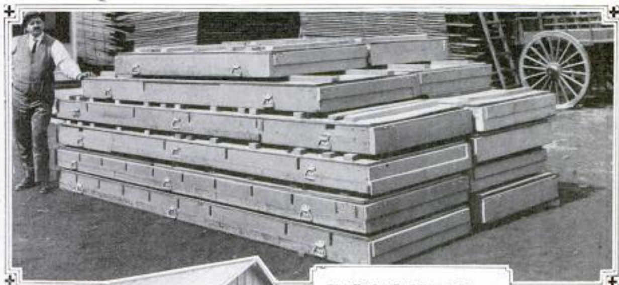
The Entire Building is Shown Here Crated so That It can be Transported on a Motor Truck
