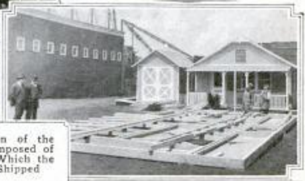
The Hospital in Process of being Erected, Showing the Manner in Which the Panels and Framework Fit Together
