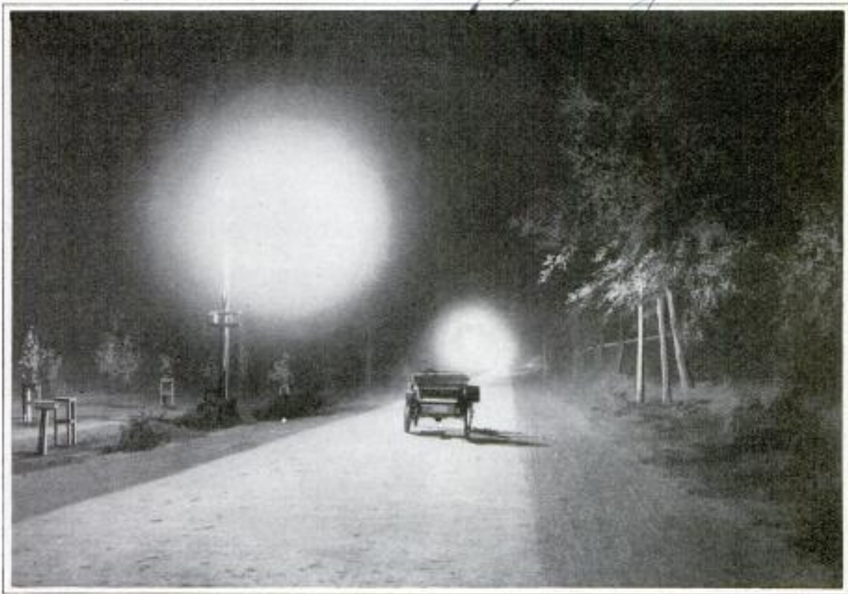
Section of California State Highway between Chico and Red Bluff Which is Well Lighted by Luminous Arcs
