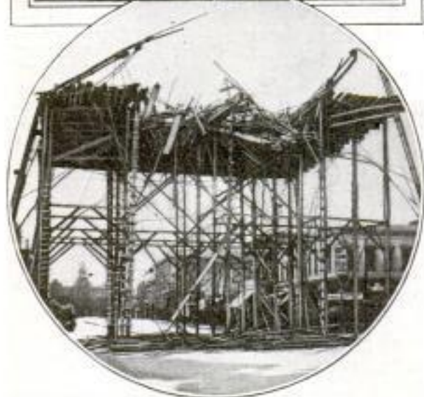
Above: San Jose's Steel Tower, 265 Feet High, As It Appeared at Night Before It was Destroyed. Below: Wreckage of the Tower After a 57-Mile Gale Swept the City
