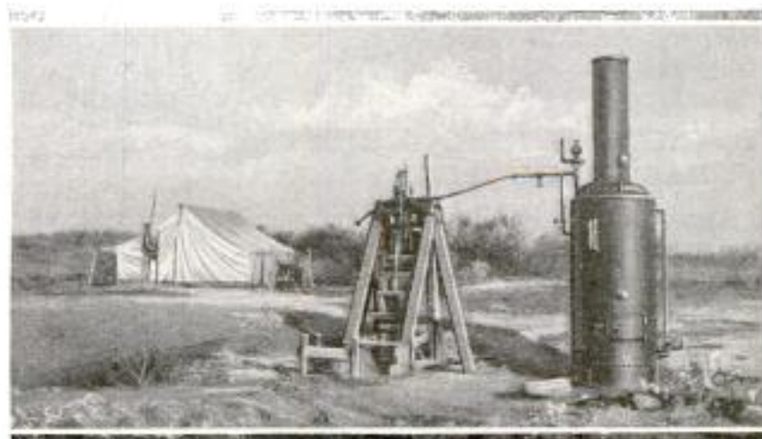
Curious Stamping Mill Which Paid Large Dividends: Old Boiler and an Air Drill Used to Crush Gold-Bearing Ore
