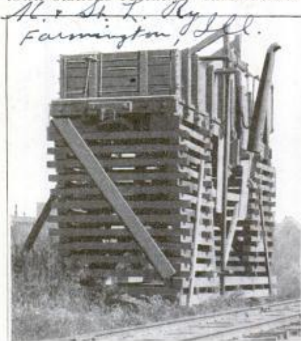
Coal Car has been Made to Serve as a Water Tank on an Illinois Railroad
