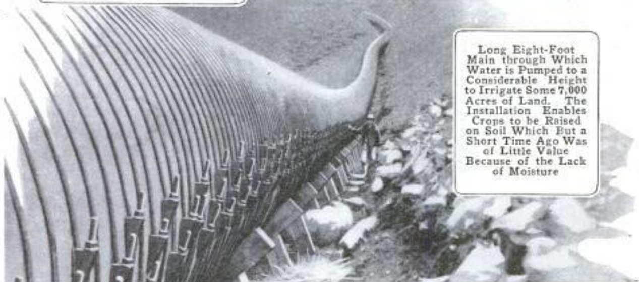
Station at Indian Cove, Idaho, Where Water is Raised 250 Feet to Irrigate Hillsides Now under Cultivation
