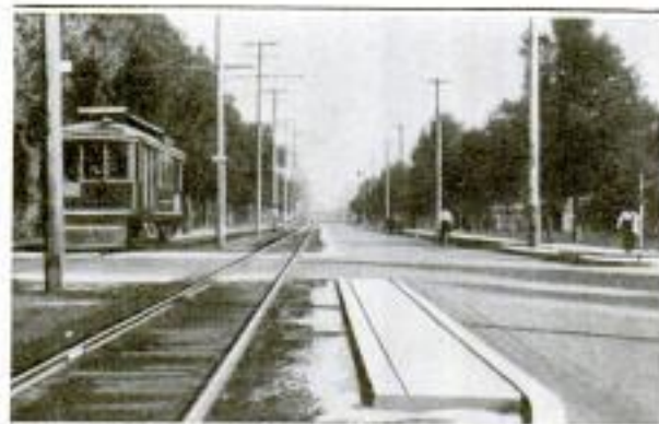
Concrete Waiting Platforms Protect Street-Railway Patrons from Passing Vehicle Traffic
