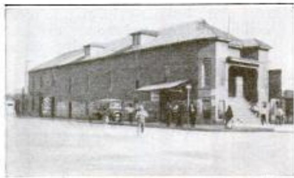
Mexicans Use One Building for Church, Saloon, and Billiard Parlor
