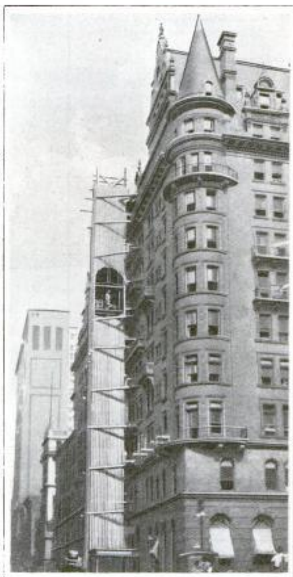
Freight Elevator on Outside of Hotel during the latter's Renovation
