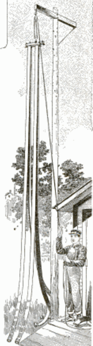
Hoist for Draining Lengths of Hose Used in a Small Fire Station
