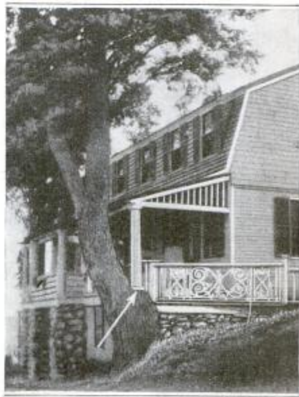
With a Shelf Cut in One Side, This Ancient Elm was Made to Serve as the Corner Foundation of the Porch
