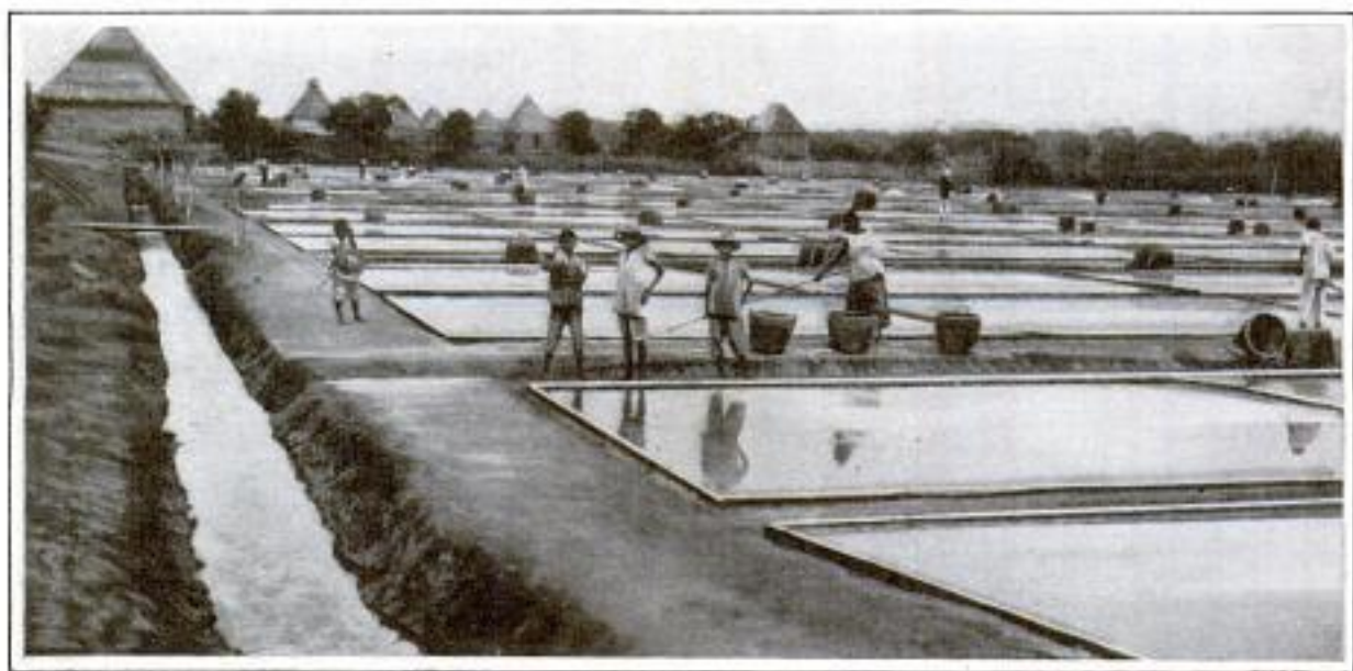
Evaporating Ocean Water to Recover Salt in the Province of Cavite
