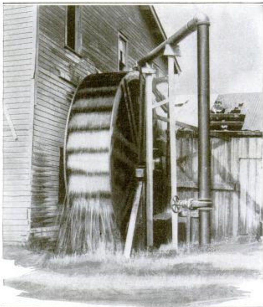
Aged Water Wheel Supplies Southern Woodworking Plant with Power
