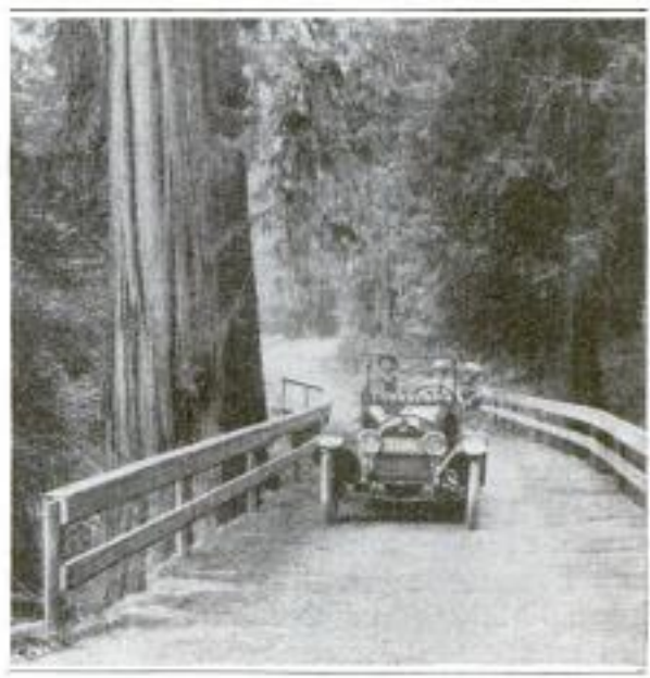
In Order to Avoid Felling This Cedar the Bridge was Built around It
