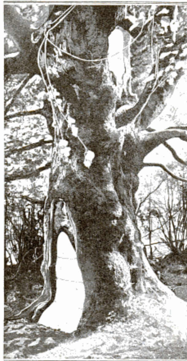
Oregon Tree Requires Concrete Column 41 Feet High as Interior Filling
