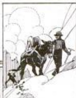
Extending Telephone Line to 9,000-Foot Level
