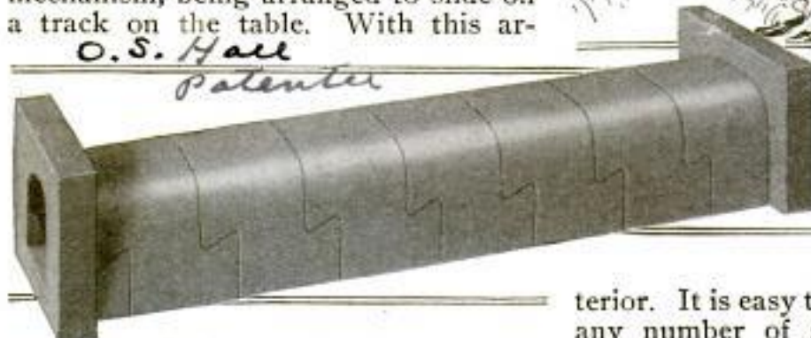
The Ends of This Culvert, as Well as the Intermediate Sections, Have Interlocking Joints
