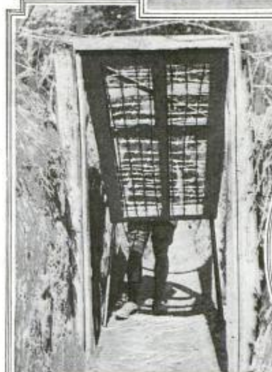
French Trench Equipped with Barbed-Wire Doors Placed 100 Yards Apart. If the Enemy Gets into the Trench the Doors are Locked to Impede Progress
