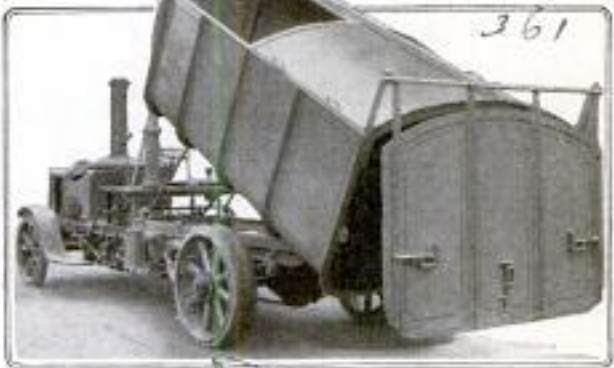
Two Views of Self-Dumping Steam Truck. Recently Brought Out in England, Which Uses Coke as Fuel
