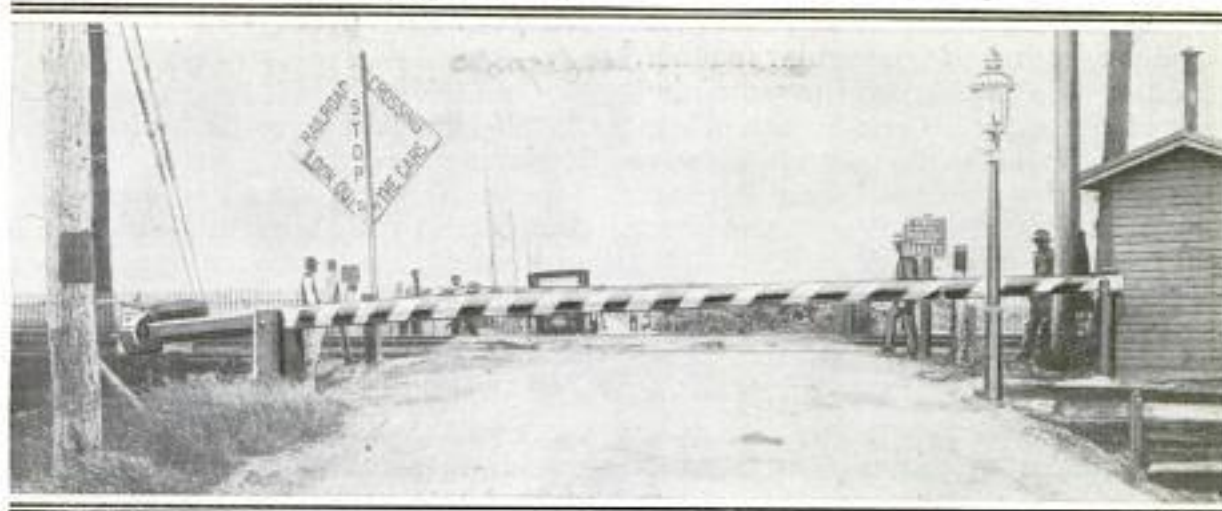
The Arms Are Strong Enough to Stop a Motor Car if Its Driver Fails to See the Danger Warning
