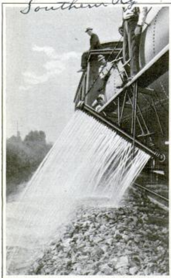
How the Chemical is Applied to the Roadbed for Killing Weeds and Other Vegetation
