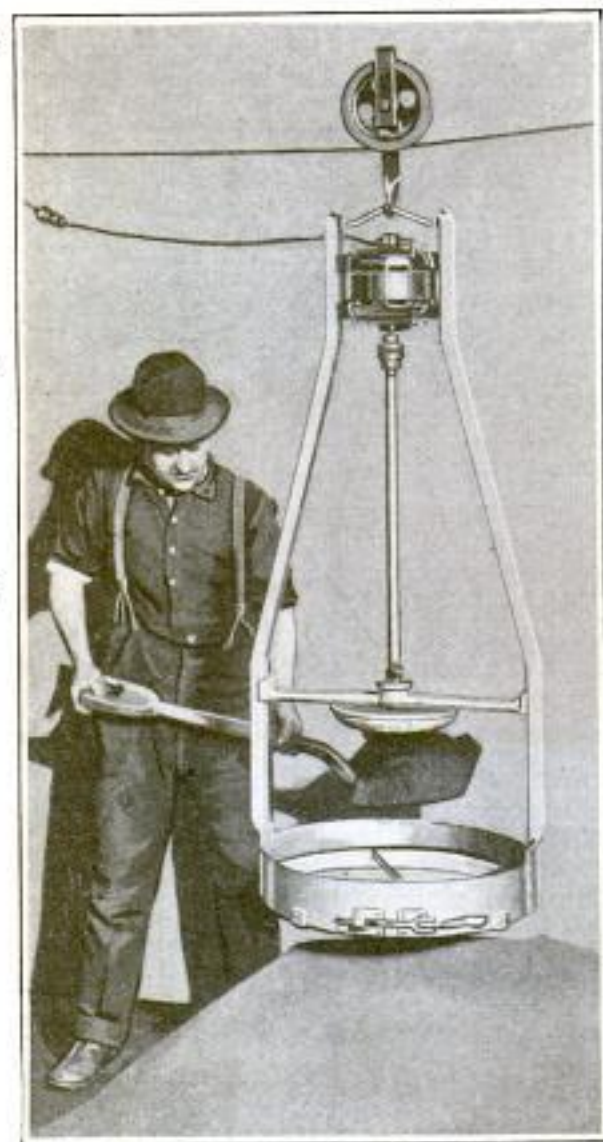
This Electric Sand Sifter is Suspended upon a Trolley and may be Moved Anywhere about a Plant
