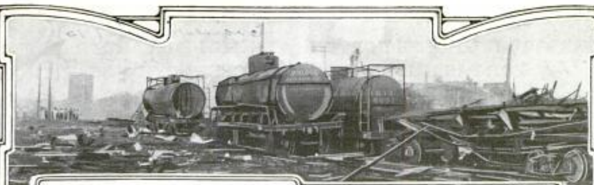
Section of the Railway Yards at Ardmore, Oklahoma, Where the Explosion of a Tank Car Recently Occurred, Wrecking a Large Part of the Town's Business District and Killing Many Citizens. Immediately Below is Shown the Railroad Station, Which was Practically Demolished. Blazing Gasoline was Spouted in Every Direction, Kindling Several Fires and Adding to the Horror
