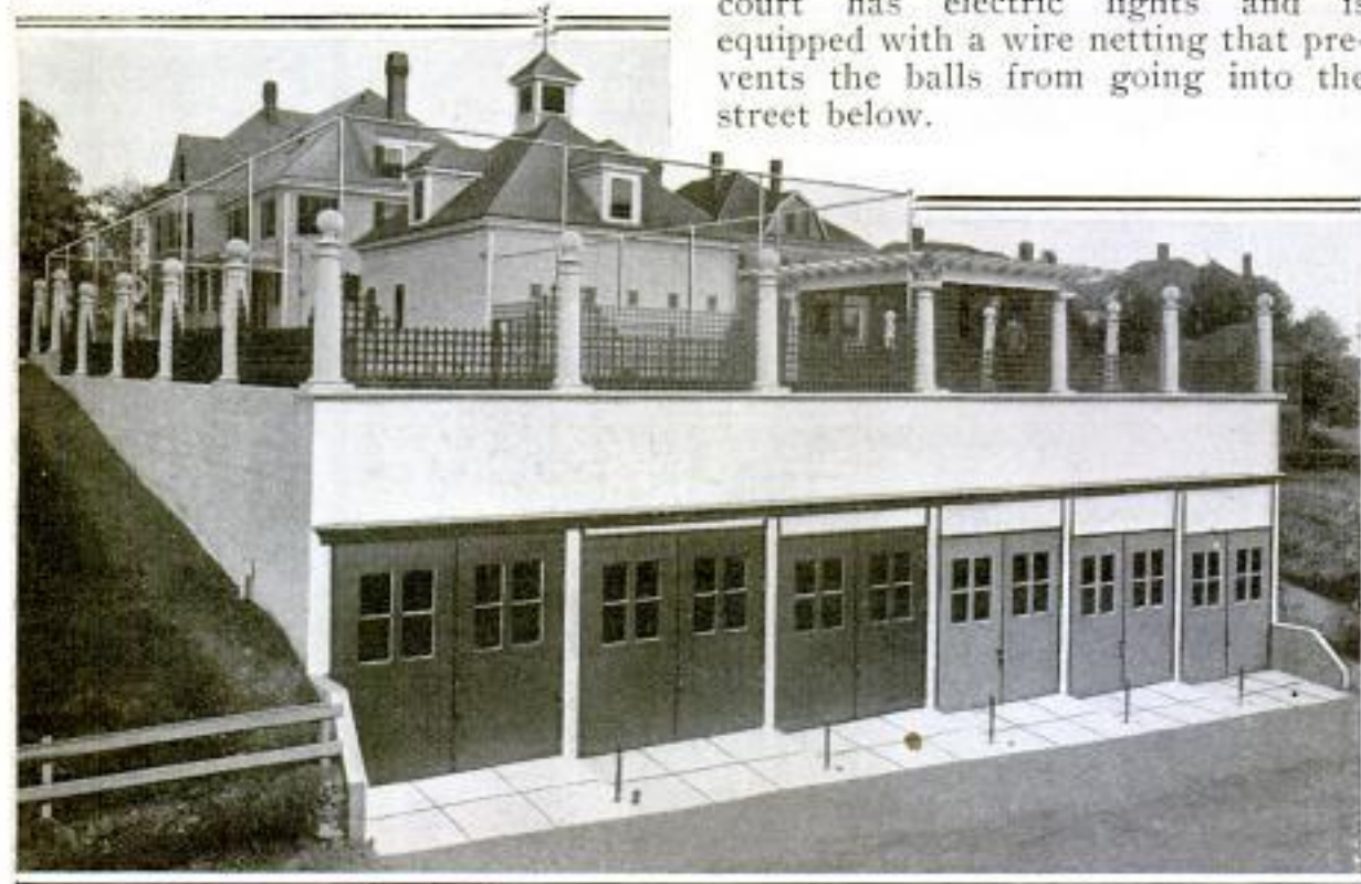
The Novel Features of This Garage Are a Garden and a Tennis Court Located on the Roof
