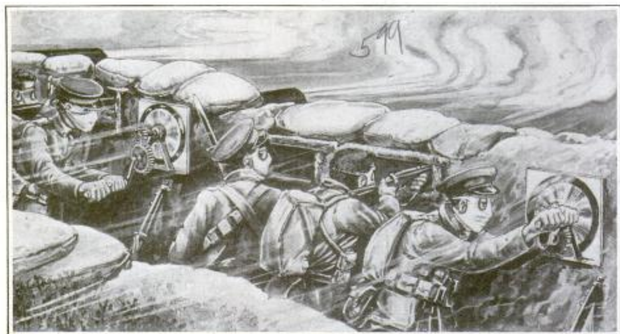
Rotary Blowers, Operated by Hand, Installed in an Advance Trench to Lift the Clouds of Deadly Gases Used by the Germans. This Plan has Recently been Proposed by the British
