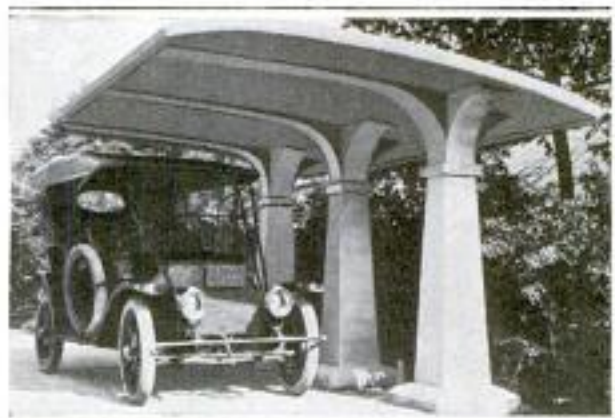
The Canopy Is of Rigid Construction and Requires No Counterweight to Balance the Roof
