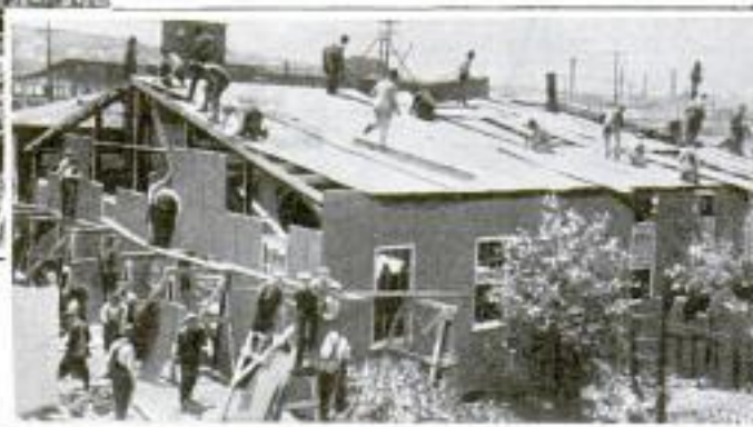
Here the Building is Shown as It Appeared Exactly Four Hours Later, When 32 Men Were at Work
