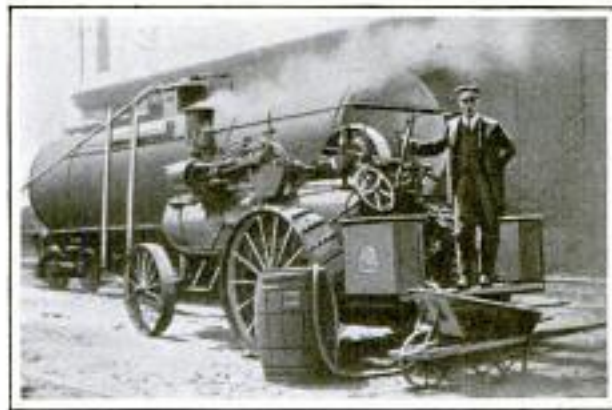
Traction Engine Used for Warming Crude Oil That had been Stiffened by the Cold
