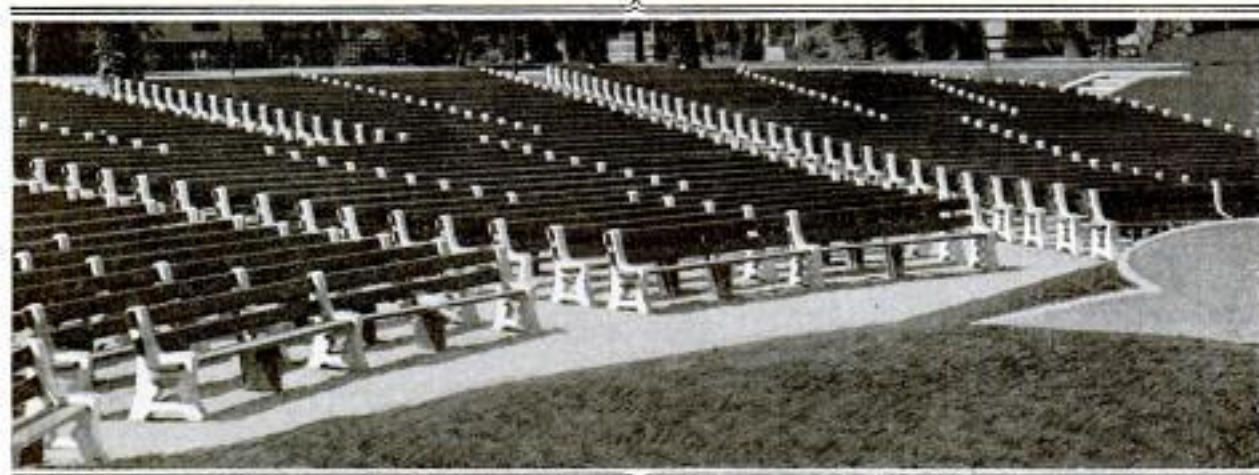
The Ground was Excavated to Allow the Floor to Slope Gradually from the Street Level to the Middle of the Park, Where the Band Stand has been Erected
