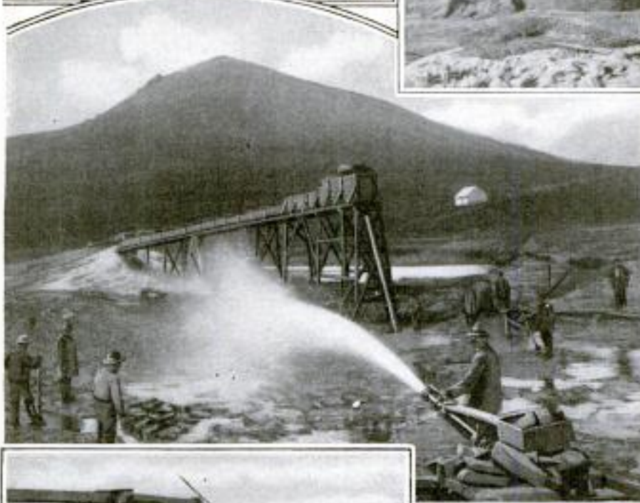
Using Hydraulic Giant for Stripping the Earth from Mineral Deposits at a Mine in Canada: This Machine Throws a Five-Inch Jet under a Pressure of 200 Pounds to the Square Inch
