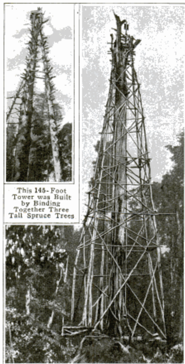
The Top of This Lone Tree Supported a Platform on Which the Geodesists' Instruments were Mounted While Carrying a Survey through a Forest
