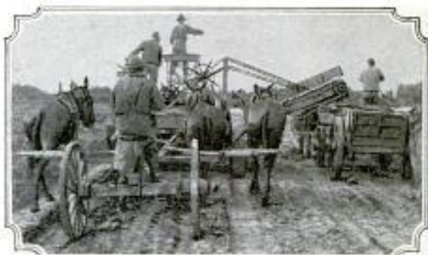
As the Grader Proceeds, the Sod and Dirt is Conveyed into Wagons Driven at the Right
