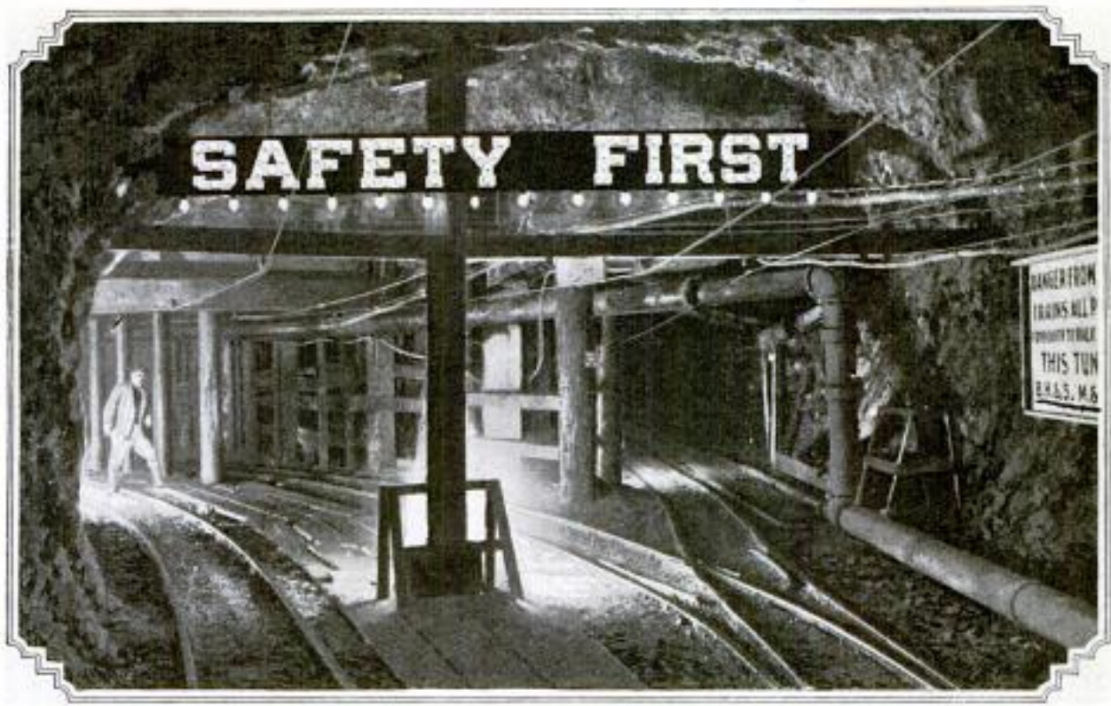
Electric "Safety-First" Sign Erected in One of the Tunnels of an Idaho Gold Mine
