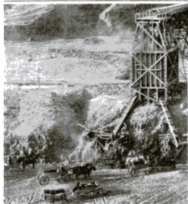
Belt Conveyor, 925 Feet Long, Used for Delivering Earth to the Truckee-Carson Dam Site
