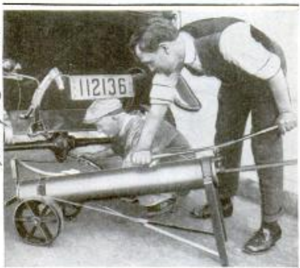
Forcing Grease from the Gun into the Differential Housing of a Motor Car
