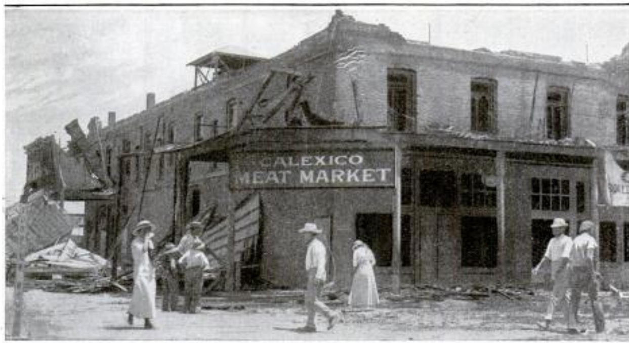
Calxico, a Border Town in Southern California, Suffered Seriously. This Shows a Partly Destroyed Building Which Fared No Worse than Many Others
