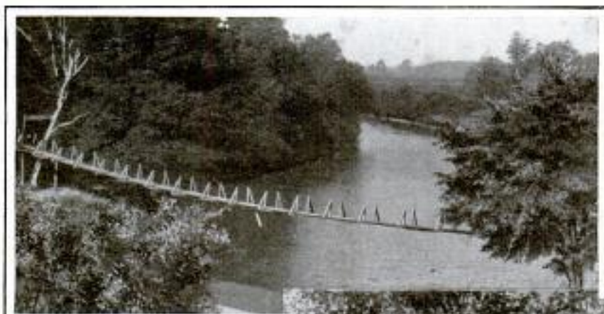
The Planking is Supported on Top of Two Parallel Steel Cables
