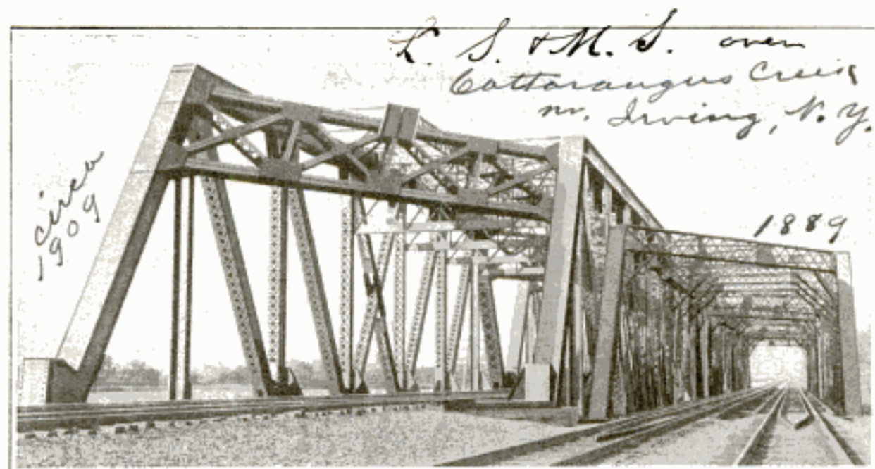
8608 Two Bridges of Different Periods Which Illustrate the Advance Which has been Made in Railway-Bridge Construction
