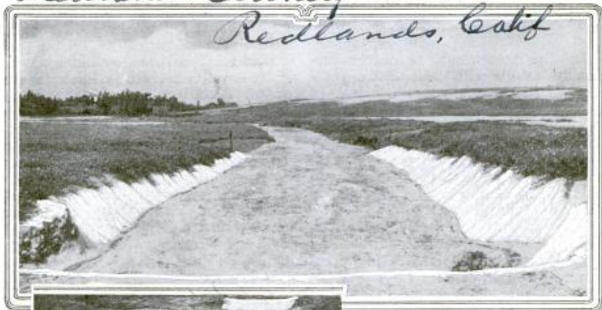
The Banks of the Cuts are Reinforced with Cement, to Preserve Golf-Links Hazards
