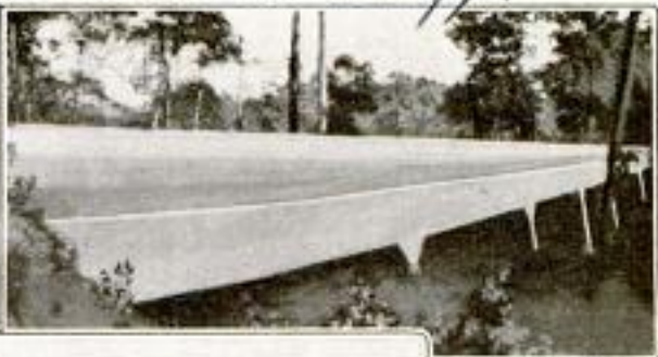
At Left, the Filter Beds in Operation: The Liquefied Sewage is Sprayed over the Beds, under Which Air is Introduced by the Ventilating Funnels
