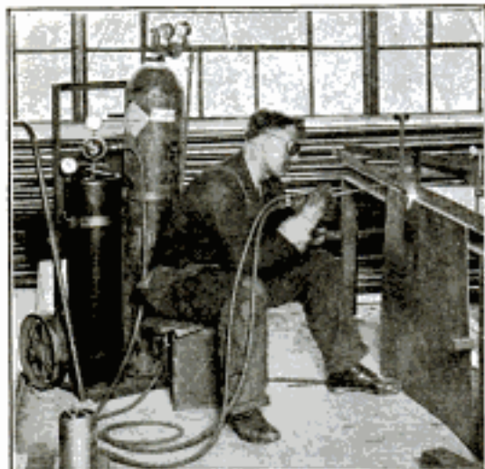
Manufacturing gas tight rectangular tanks from sheet steel by oxy-acetylene welding. These tanks are part of the large acetylene purifying apparatus used at the various charging plants of The Prest-O-Lite Co., Inc., in its extensive acetylene service system.
