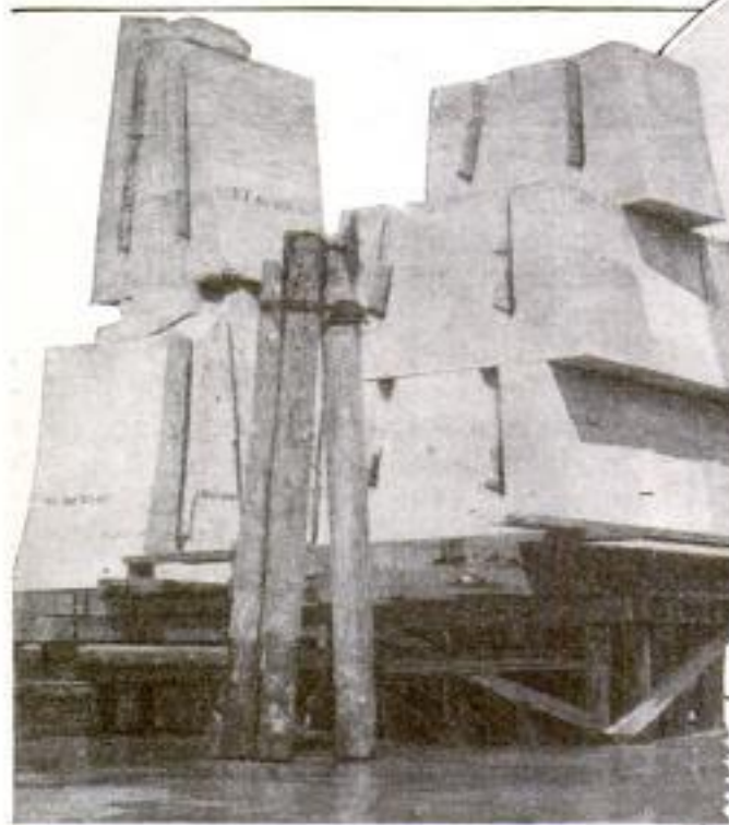
These Concrete Blocks, Weighing 240 Tons in All, were Loaded on Successive Sections of the New 1,000-Foot Piers in New York Harbor to Test the Bearing Power of the Pile Foundations
