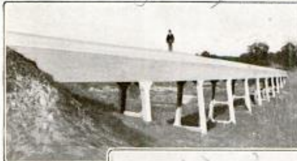
In the Pictures Above Two Views are Given of the Concrete Aqueduct, 276 Feet Long, That Forms Part of the Sewage Disposal System at Atlanta, Ga.
