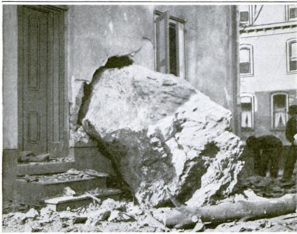
Two-Ton Rock Hurlled against Dwelling House by a Heavy Blasting Charge: Part of This Rock Went through the House, Taking the Breakfast Table with It
