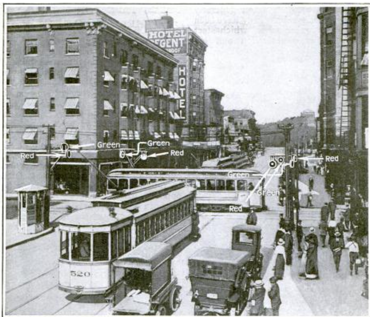
With This Crossing-Signal System, Installed at Cleveland, Ohio, the Traffic is Controlled Entirely by the Red and Green Lights; the Crossing Officer is Stationed in the Booth at the Left
