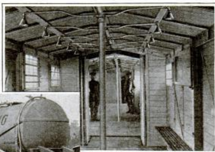
Shower Facilities in Cars Intended for Privates. The Officers' Compartments are Provided with Tubs and Dressing Rooms
