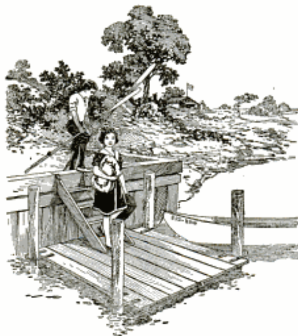
The Floating Platform Makes an Excellent Landing Place for Small Boats in Tidewaters
