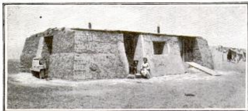
This Sod House, Built in 1914, is Located in a Timberless Section of Montana, 40 Miles from the Nearest Railroad
