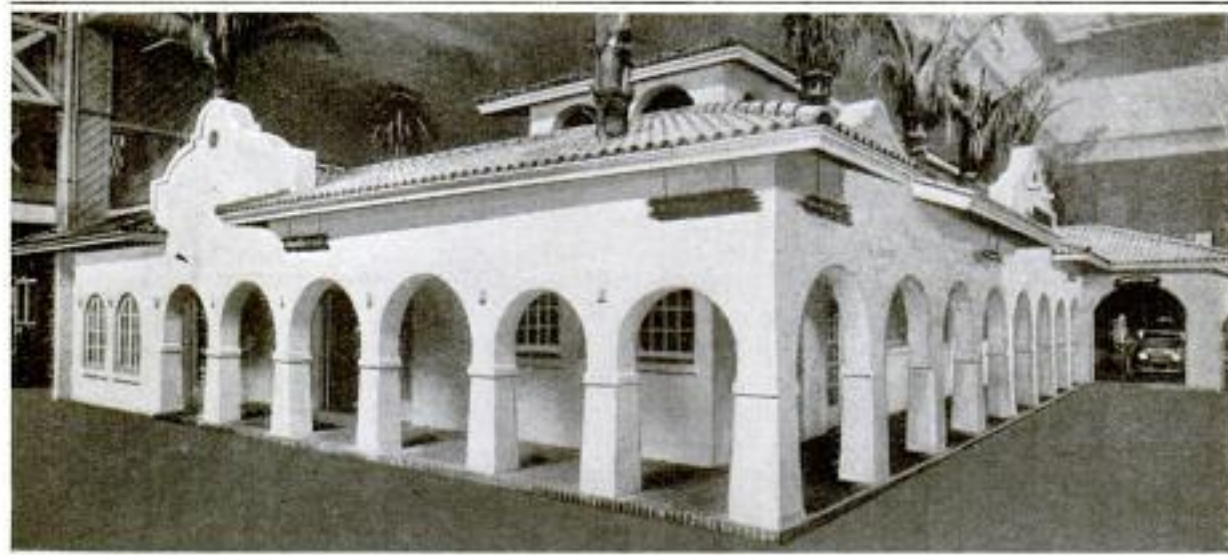
In This Bungalow Electricity is Made to Perform Practically All Domestic and Personal Services. The Meals are Cooked, the House Cleaned, the Rooms Heated and the Air Freshened by Pushing a Button
