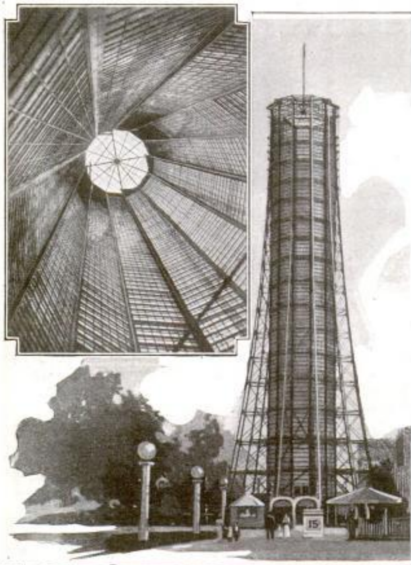
Remarkable Glass and Steel Tower in Which, without Cables or Plungers, a Large Elevator is Raised on a Cushion of Air to a Height of More than 200 Feet
