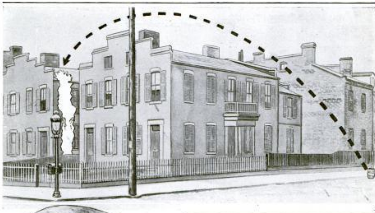
Iron Cover Plate Blown from a Sewer Manhole through an Adjacent House: The Barrel Marks the Position of the Sewer Vent, While the Dotted Line Indicates the Course Taken by the Heavy Cap
