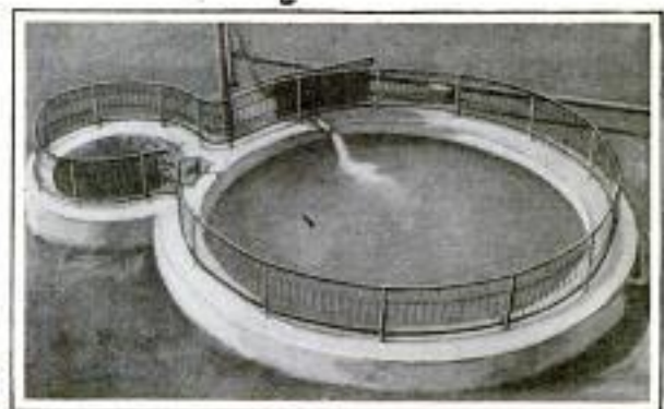
The Flow from Artesian Well is Increased 100,000 Gallons a Day by the Centrifugal Pump Located in the Housing at the Edge of the Reservoir
