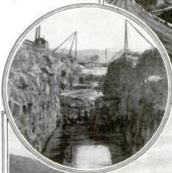
Excavation for Tandem Lock Completed and Ready for the Concrete
