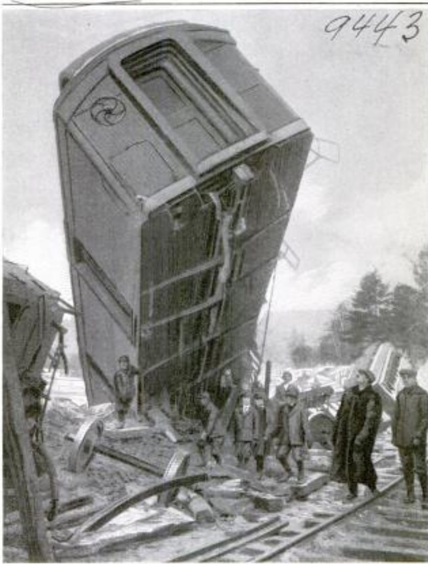
Unusual Position of the Baggage Car Following a Train Wreck in New Hampshire
