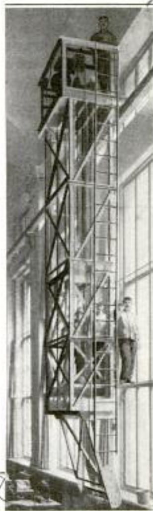
The Picture at the Top Shows the Traveling Crane with Electric Lift, Used in Cleaning Windows; Arched Crane for Cleaning Skylight Shown at Left
