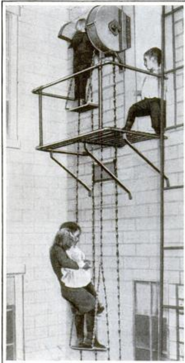
Consisting of an Endless-Chain Ladder, This Fire Escape Requires Only the Power Derived from the Weight of a Passenger to Operate It
