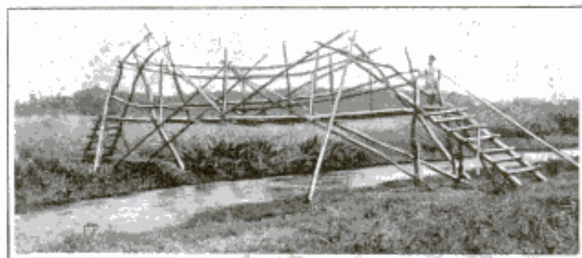
Philippine Bridge Made of Bamboo with Cantilever Principle
