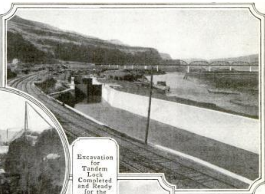
Canal and Railways Paralleling The Dalles
