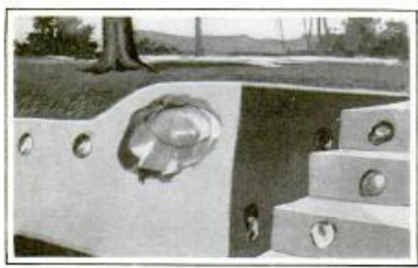
Novel and Attractive Effect Produced by Imbedding Shells in a Concrete Garden Wall
