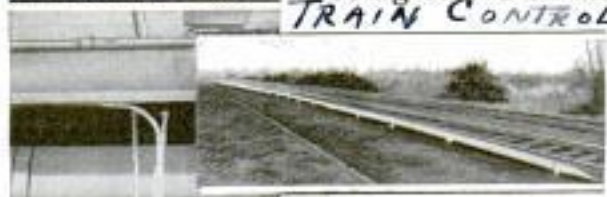
How the Ramp and Contact Shoe are Arranged in a New Automatic Train Stop
