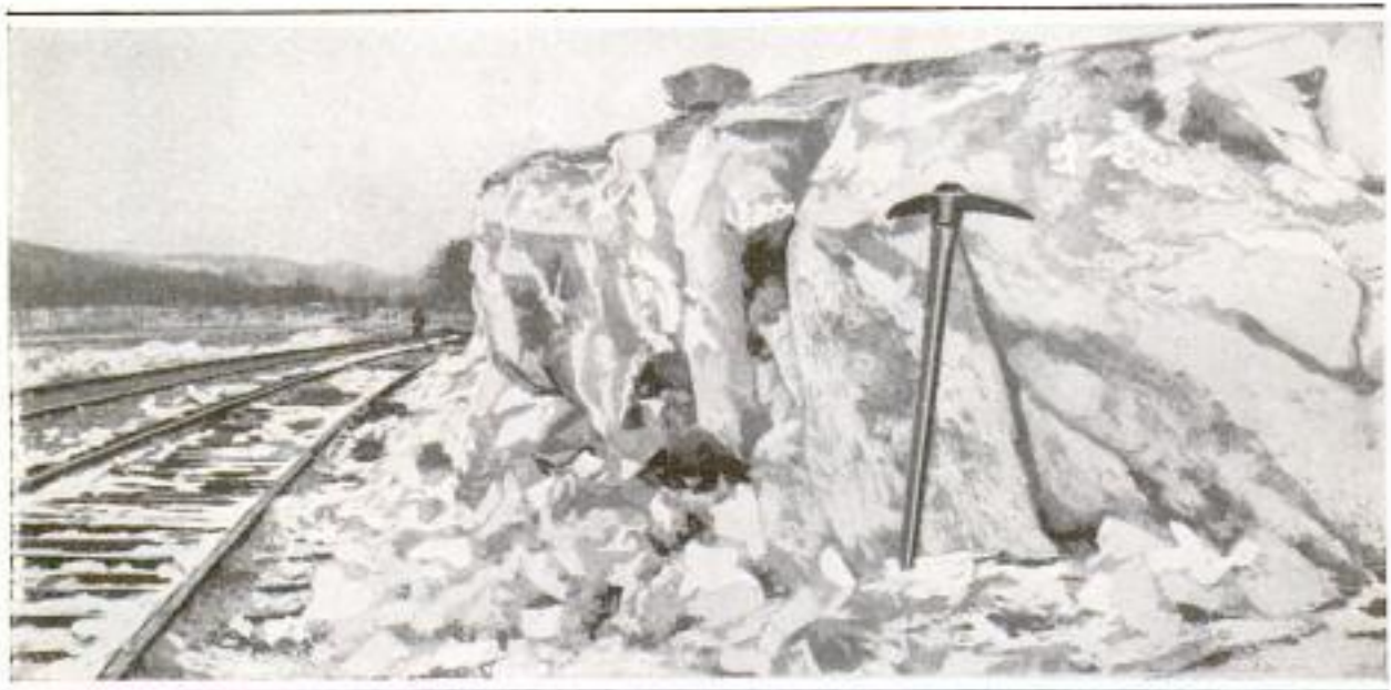
This Shows the East-Bound and Middle Track Cleared of the Ice. The Third Track is Hidden beneath the Ice Embankment
