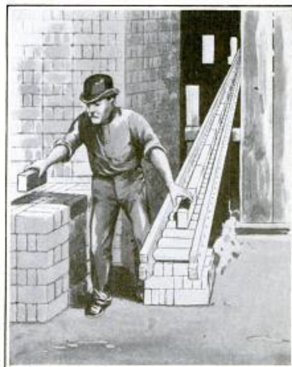
Handling Bricks on a Building Site with the New Conveyor
