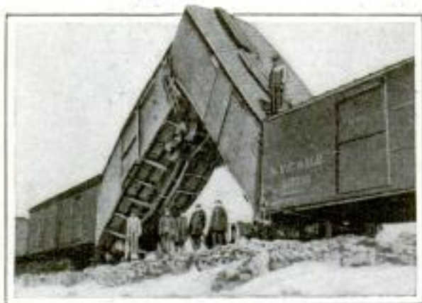
Two Cars in the Middle of a Long Freight Train Buckled When a Head-On Collision Occurred
