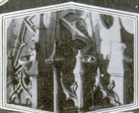
Above is shown a cluster of projectors hidden in the ornamentations on a side of one of the Tourelles. While at the right is the Woolworth Building as it now appears at night when its tower is illuminated.
