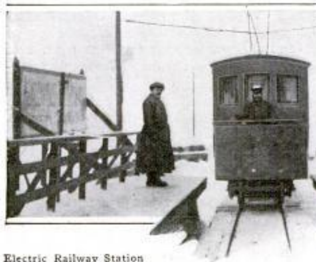
Electric Railway Station on the Ice of the River Neva in Petrograd, Russia; This Railway is Built on the Ice Each Year and is Kept in Service throughout the Winter
