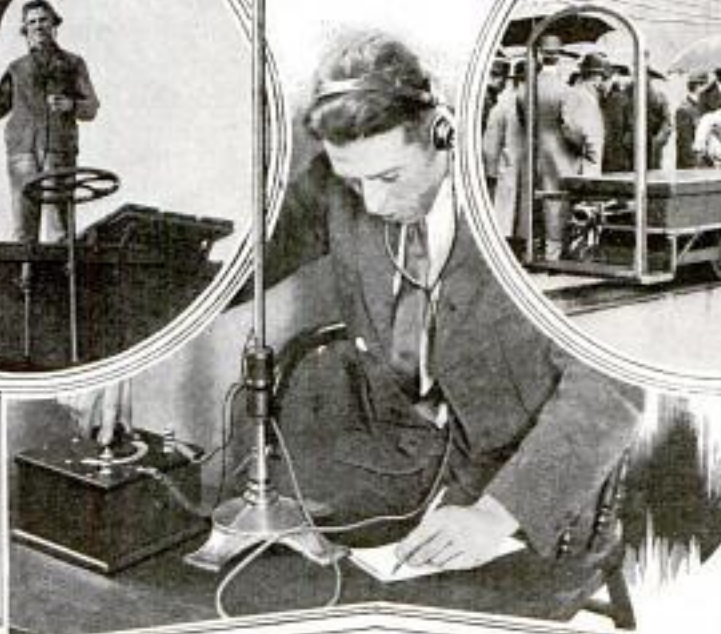
With the Ribs of the Umbrella Acting as Antennae, This Brakeman is Receiving a Wireless Message from a Station Located Several Hundred Feet Away
