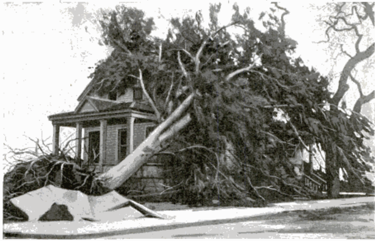
This Large Tree was Uprooted during a Storm and Hurled against the House, Partly Wrecking It
