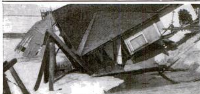
Wreckage of the Board Walk on the Bulkhead which Gave Away, Allowing the Breakers to Sweep the Beach
