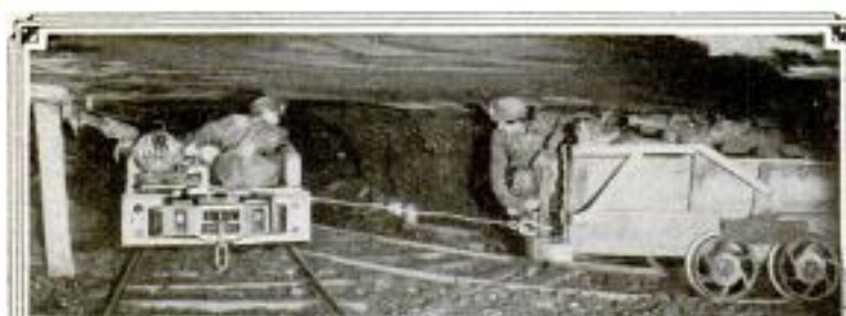
Using the Drum and Cable to Haul Loaded Car Out of a Room
