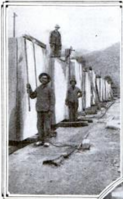
Marble Blocks being Cut into Uniform Sizes by Means of a Wire Saw Which Passes through the Entire Line of Stone
