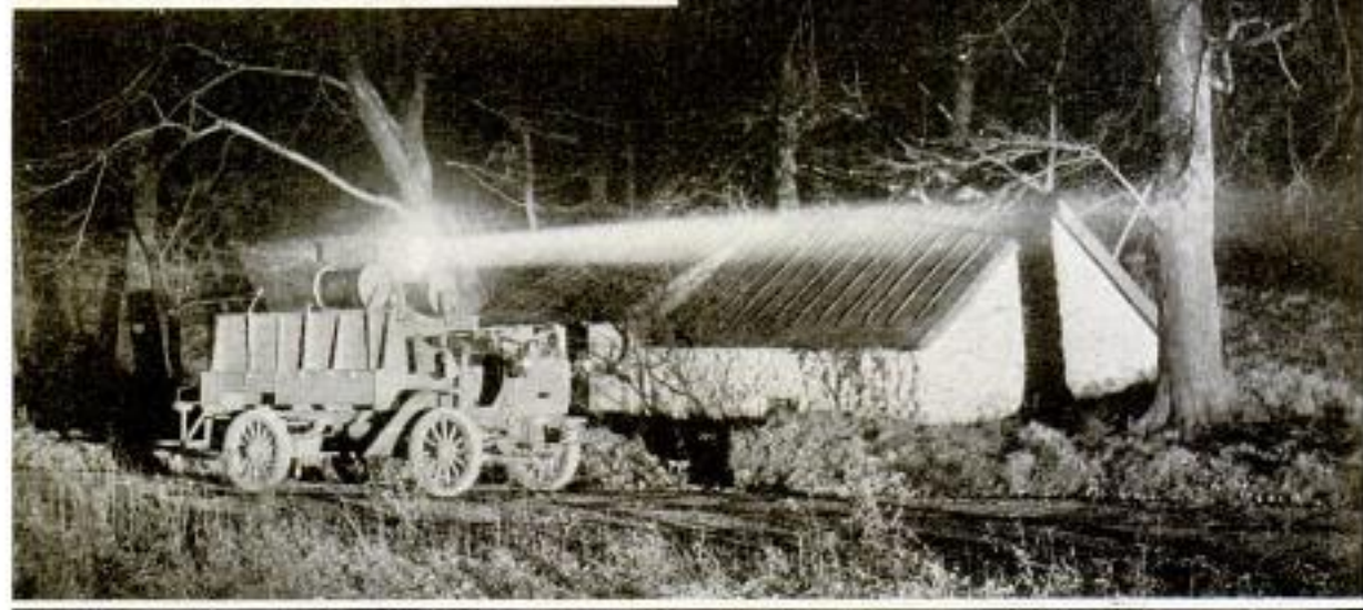
This Military Searchlight Battery was Employed Recently at Philadelphia When It Became Necessary to Repair Electric-Light Lines at Night
