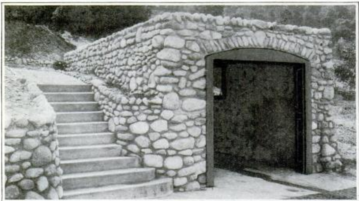
This Attractive Garage is Built of Cobblestones Picked Up about the Owner's Suburban Place
