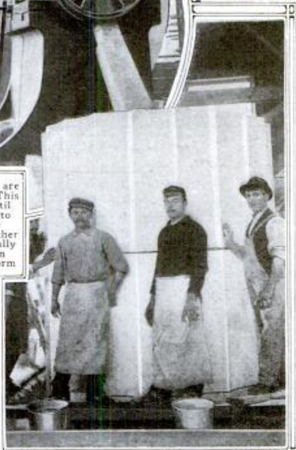
This Shows the Last Stage in the Work. The Two Drums Shown Here are being Polished and Fitted
