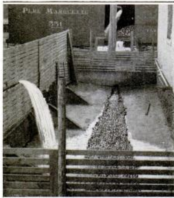
Apples are Washed Out of the Car by a Stream Thrown from a Hose, and Float Down a Channel to Conveyors That Lift Them to the Cider Machines
