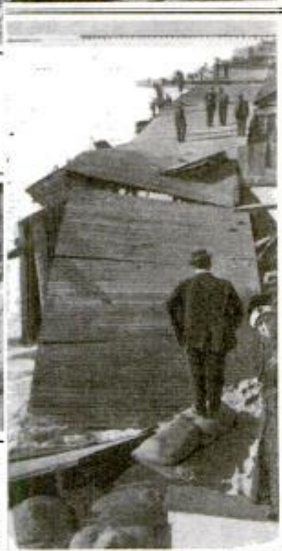
Wreckage of the Board Walk on the Bulkhead which Gave Away, Allowing the Breakers to Sweep the Beach
