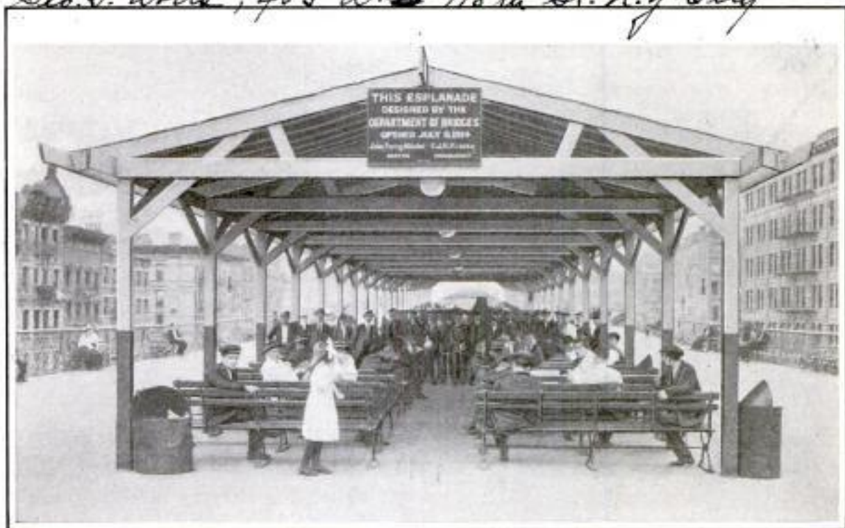
This Elevated Structure, Which Provides a Recreation Place for Several Thousands of Persons in New York's East-Side District, is Situated at the West End of the Williamsburg Bridge
