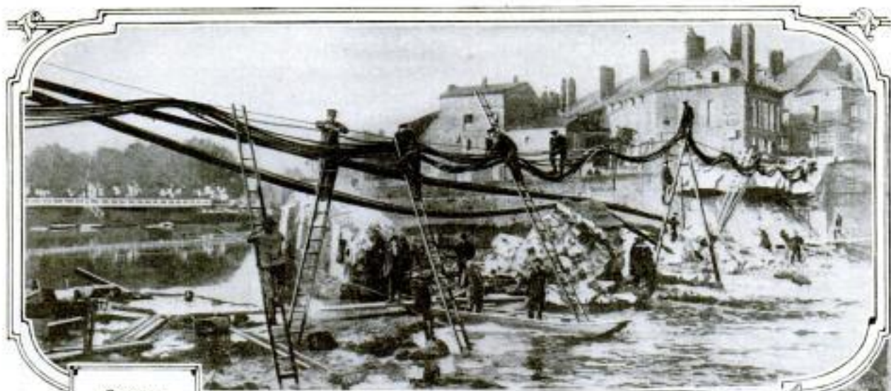
German Engineers in Belgium Repairing Telegraph Conduits
