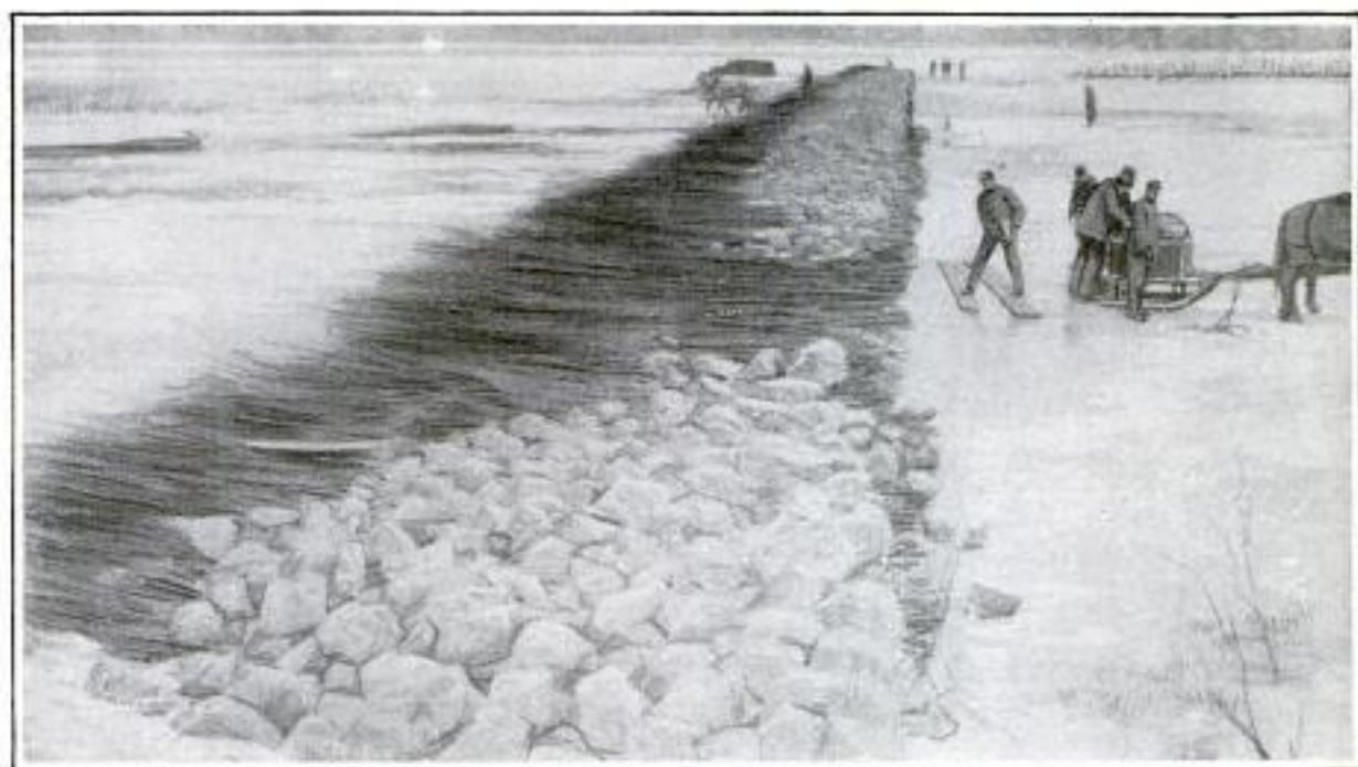
One of the Wing Dams Built on the Ice of the Upper Mississippi River in the Government's Work of Deepening the Channel
