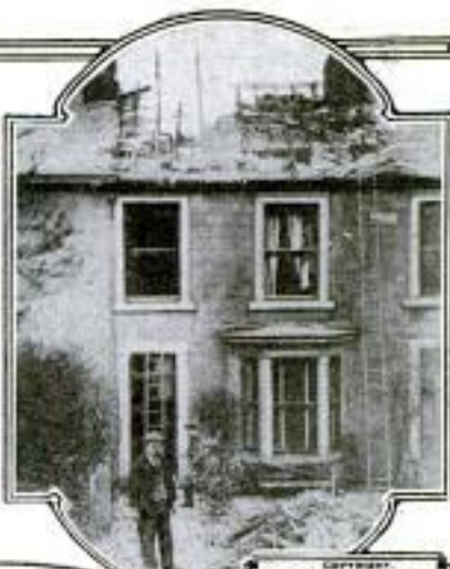
COPYRIGHT UNDERWOOD & UNDERWOOD Several Persons were Killed and Many Houses Demolished When Whitby was Fired Upon without Warning
