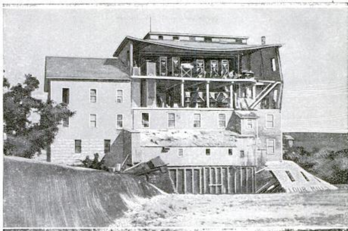
The Result of a Flour-Dust Explosion in a Nebraska Mill
