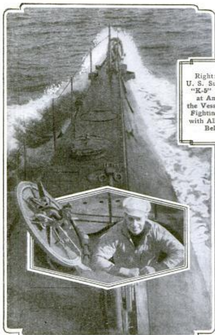
Forward Deck of the "K-5": In This Picture is Also Shown One of the Hatches That Furnish the Only Means of Entering and Leaving the Submarine
