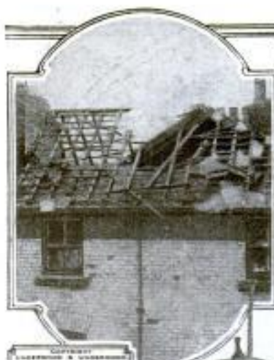
COPYRIGHT, UNDERWOOD & UNDERWOOD A Shell Striking This House Wrecked the Roof and Interior, but Did Little Damage to the Walls
