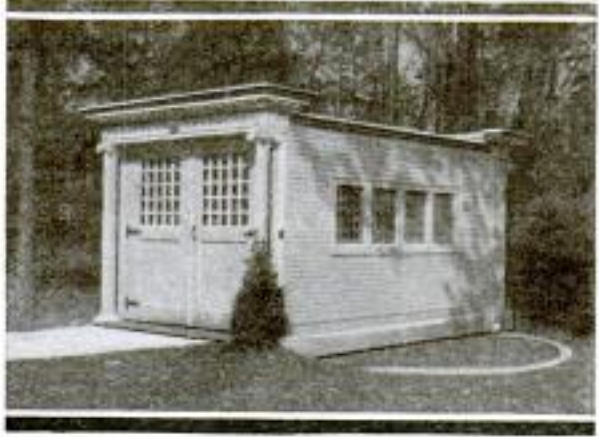
This Garage is Built So That It may be Turned End for End, Thus Eliminating the Necessity of Backing a Car Either When Entering or Leaving
