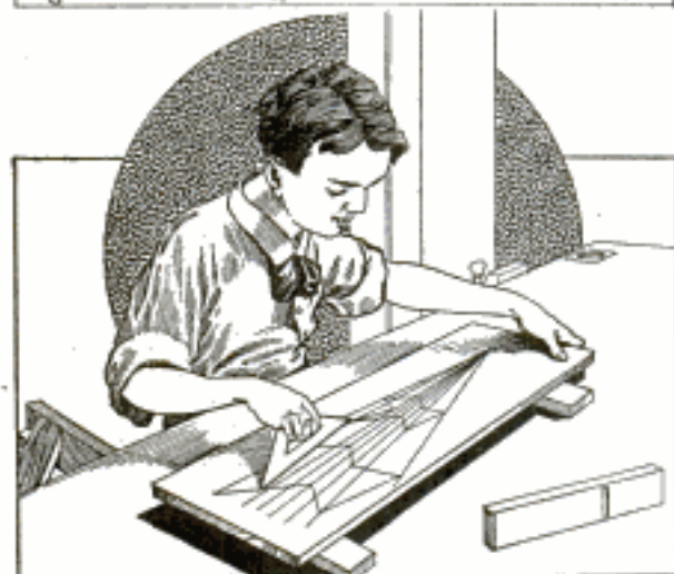
Enlarging and Reducing Plots by Radial Lines from a Common Point Located Properly
