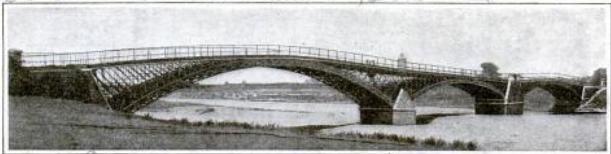
Curious Arrangement of Grades That Resulted from Building a Bridge for One Location and Then Erecting It, with Spans Transposed, on Another Site
