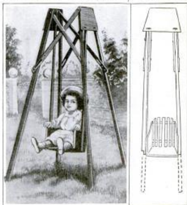
When Not in Use This Swing may be Folded Compactly and Stored in a Small Space
