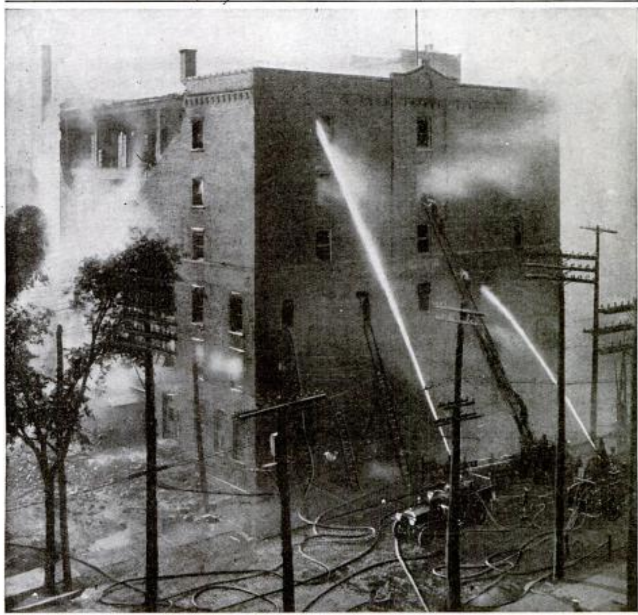
A Stubborn Fire Resulted When Several Carloads of Matches Stored in This Building were Ignited
