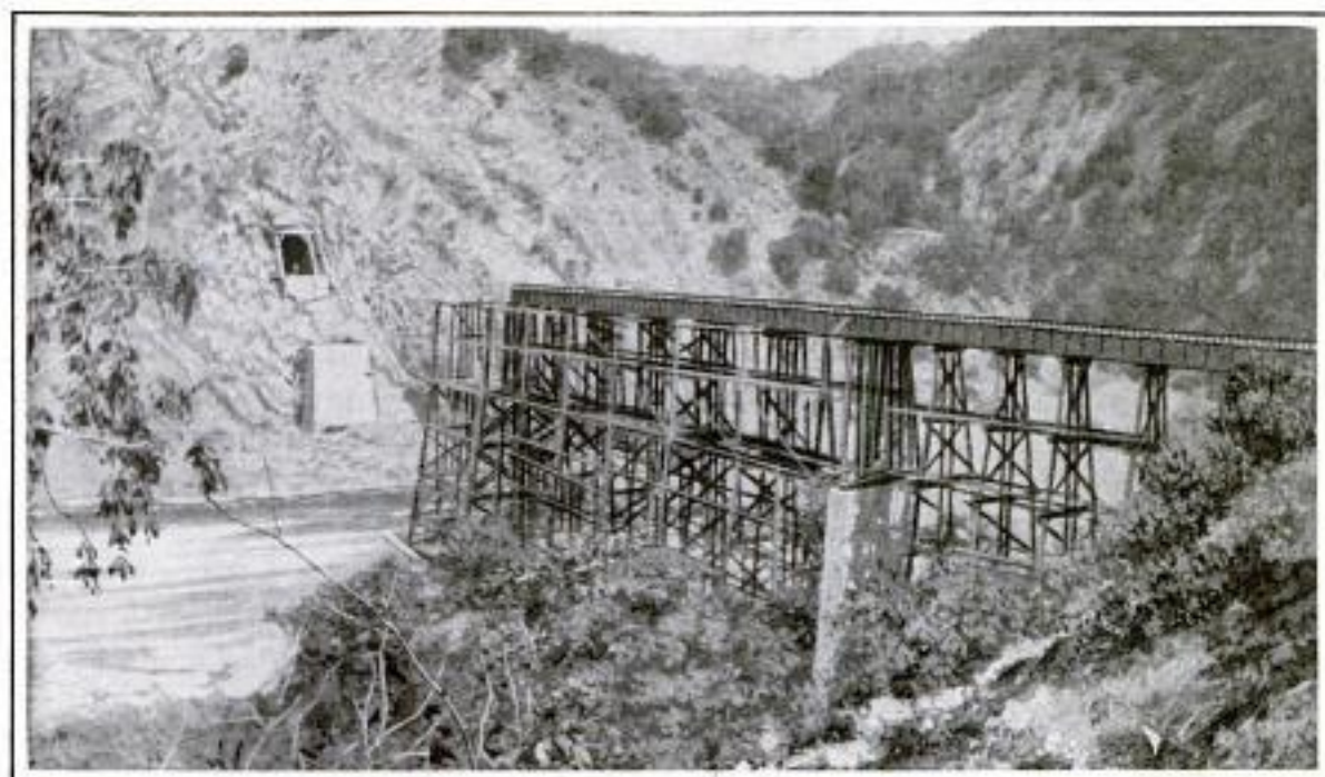
Building the Bridge to Island Mountain Tunnel: The River Takes Eight Miles to Get to the Other Side of the Mountain While the Tunnel Goes Through in 4,300 Feet
