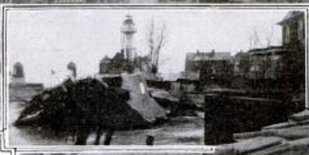
Houses along the Beach at Sea Gate, L. I., were Washed into the Sea after the Bulkheads Gave Way
