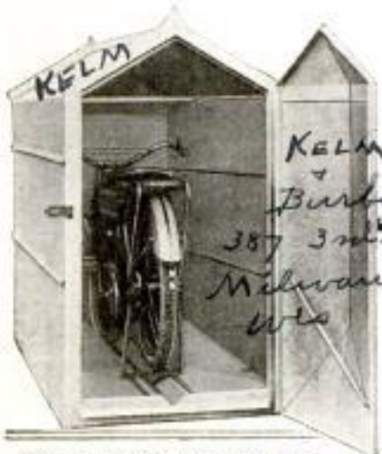
This Little Garage, Made of Galvanized Iron and Fastened Together on the Inside, Is the Last Word in Convenience for the Motorcyclist
