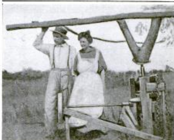
Circular Sweep Connected to a Grindstone by an Arkansas Farmer
