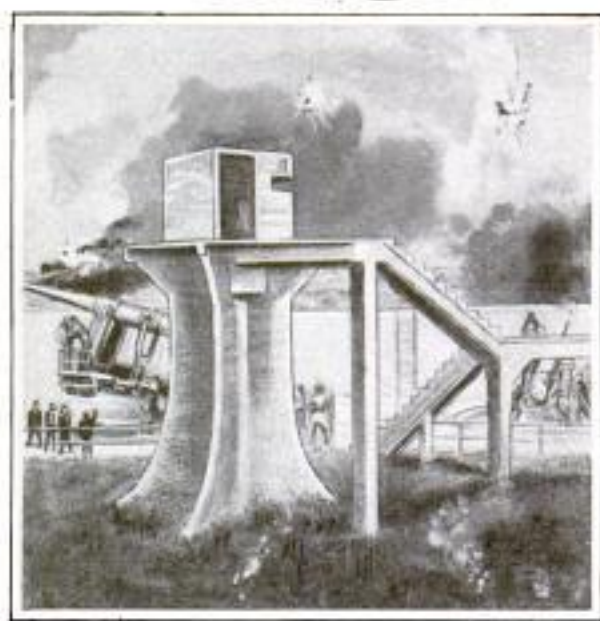
One of the New Concrete Lookout Towers for Coast Fortifications
