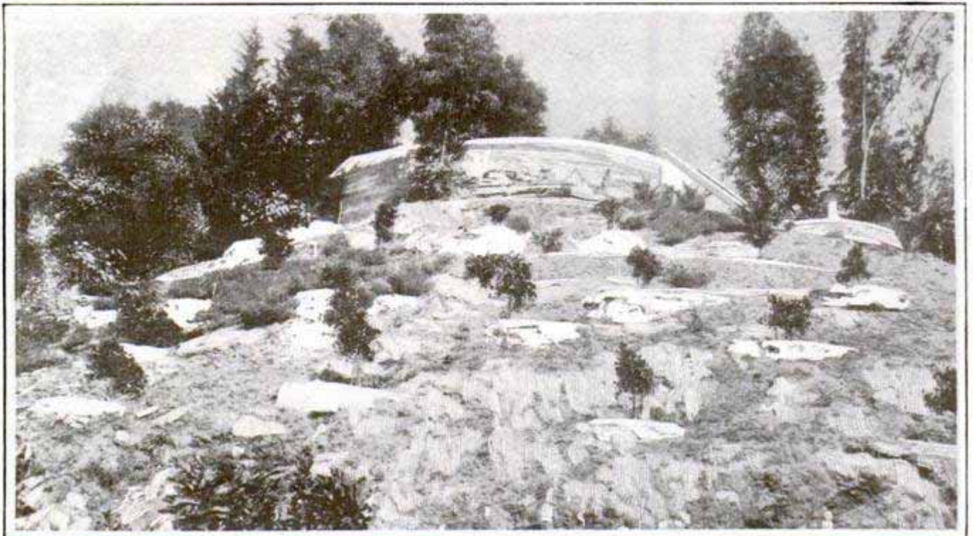
How a California Fruit Grower, by Building Semicircular Retaining Walls, Utilized a Steep Hillside for Planting Fruit Trees
