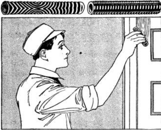
Tools Cut from Pieces of Garden Hose for Making Grains of Wood in Painted Surfaces
