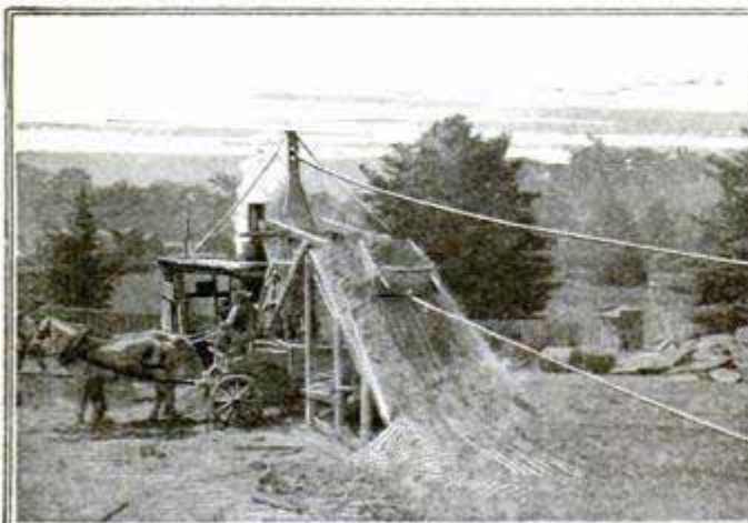
Loading Chute: The Loaded Buckets are Drawn to the Top of the Incline Where They Dump Automatically through the Chute into the Wagons
