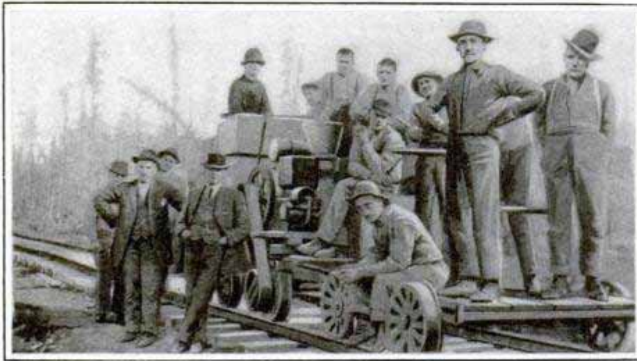
This Crude Outfit, Used on a Canadian Railway in Time of Washout, Was Capable of Making a Speed of 20 Miles an Hour
