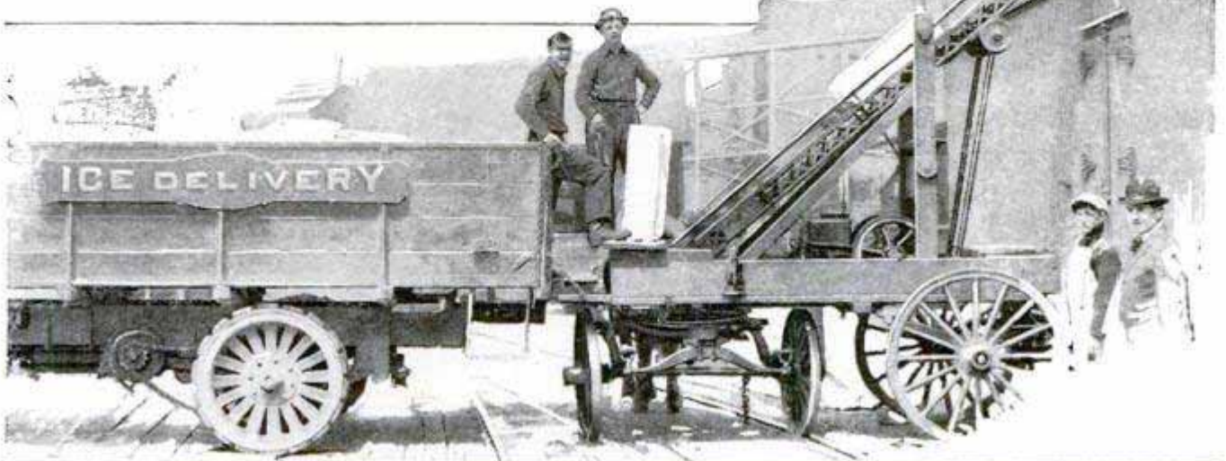
Icing Refrigerator Cars with the Aid of a Baled-Hay Loader
