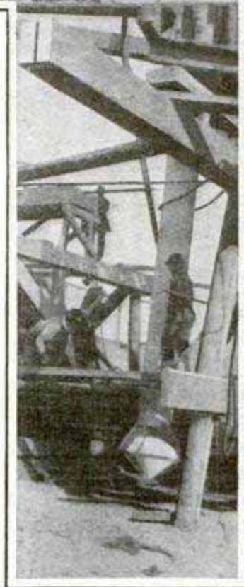
Preparing to Put a Concrete Pile in Place
