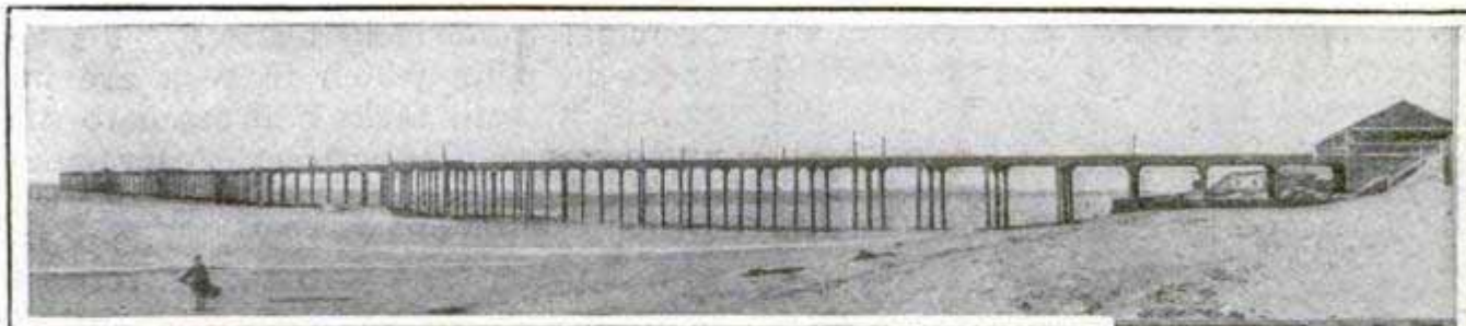
Pier after Its Completion, Showing Its Great Length and Slender Piles
