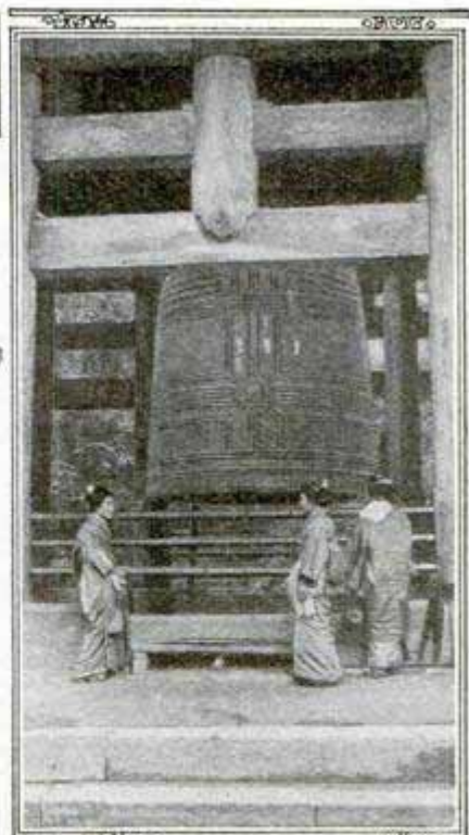
This Great Bell, at Kyoto, Japan, is Rung by Striking a Heavy Wooden Beam against Its Side
