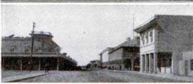
Second Stories of Business Houses in El Centro are Built Out to Shade the Sidewalks
