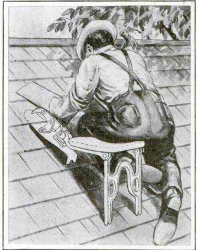
Chair Which Gives Level Seat for Roof Workers
