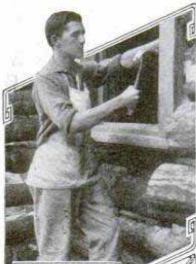
Setting a Window Frame in a Log Building
