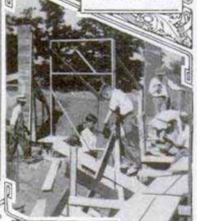
Setting the Forms for a Concrete Foundation
