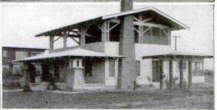
No Walls to Second Story of House
