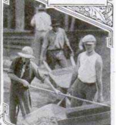
Wheeling Concrete for Foundation of a New Building
