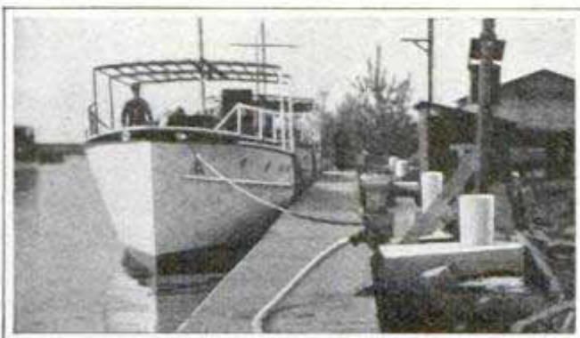
Concrete Snubbing Posts for Docking Boats
