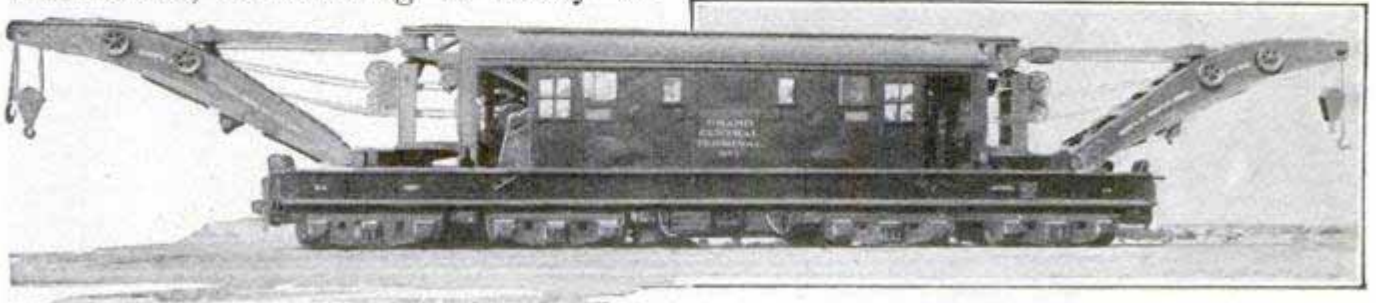
An Electric Tunnel Crane with a Speed of 25 Miles an Hour
