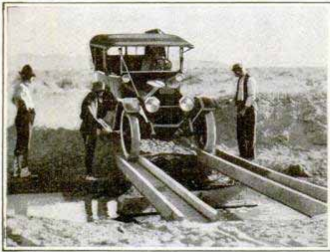
These Grooved Tracks Form a Bridge for Motorists
