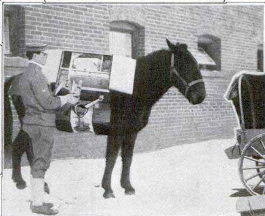
Demolition Equipment of Engineer Corps Packed for Transportation
