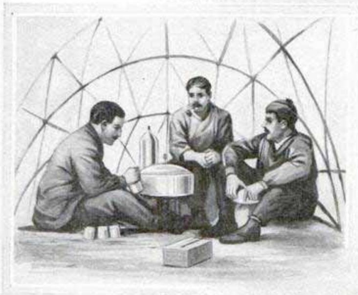
Interior of Folding Hood Tents for Antarctic Exploration: They can be Erected in the Severest Windstorm and Shelter Six Men Each, While They Weigh But 37 Pounds. Below is an Exterior View of the New Tent
