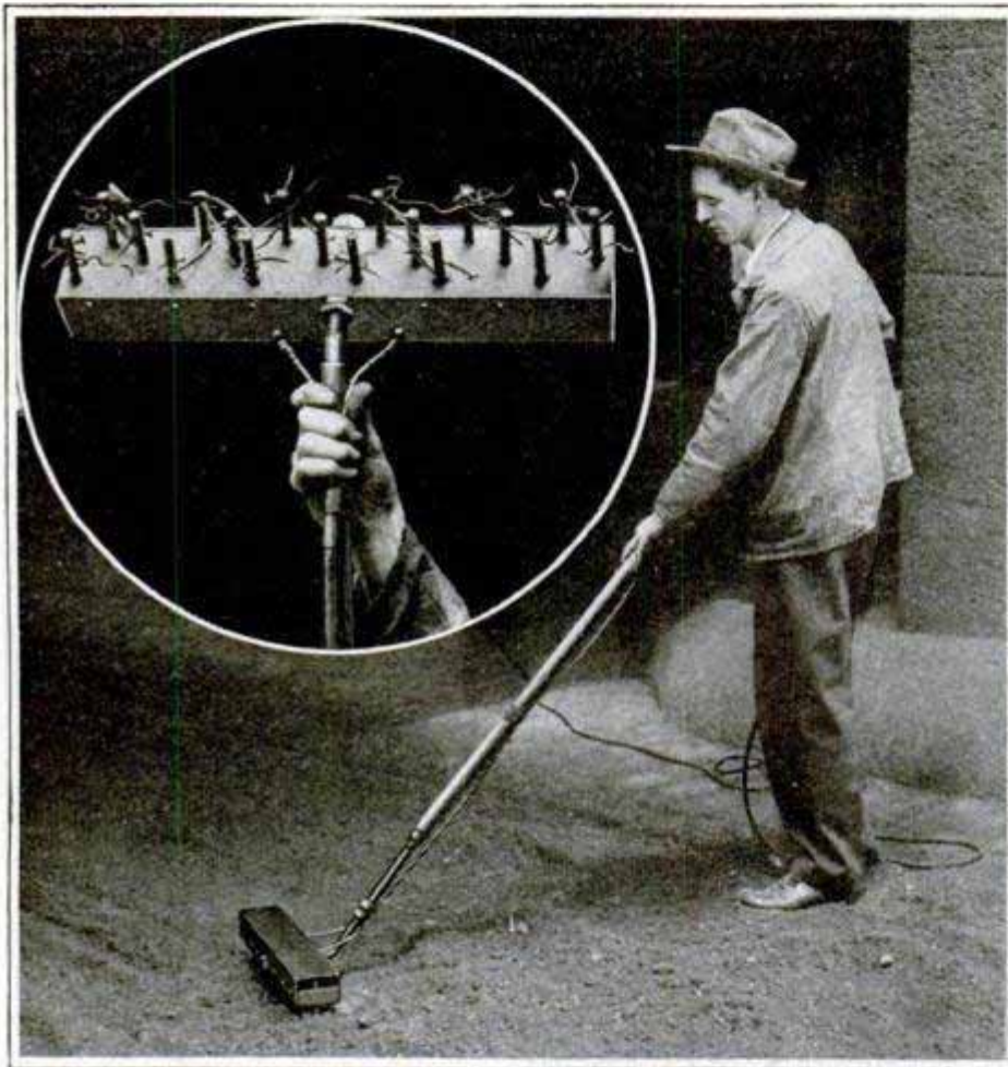
This Electromagnetic Rake Clears a Cinder Roadway of Loose Nails and Pieces of Wire
