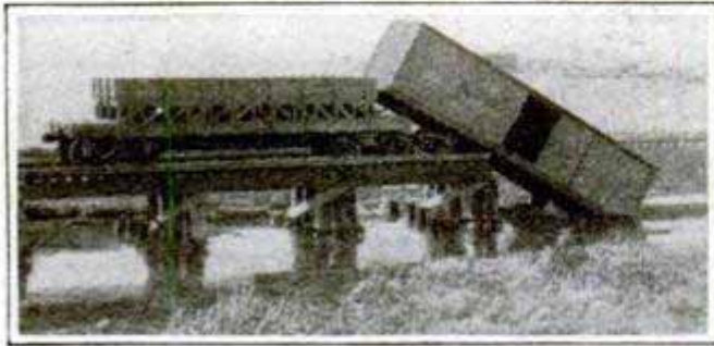
Box Car Blown from Trestle by Wind
