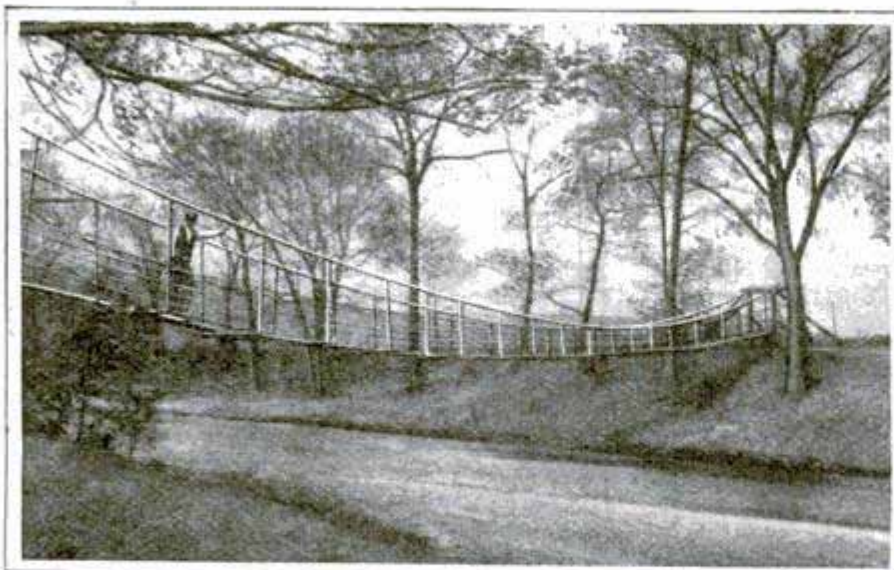
This Footbridge was Built Mainly of Old Wagon Tires and Woven-Wire Fencing, the Only New Material in It Being the Cables
