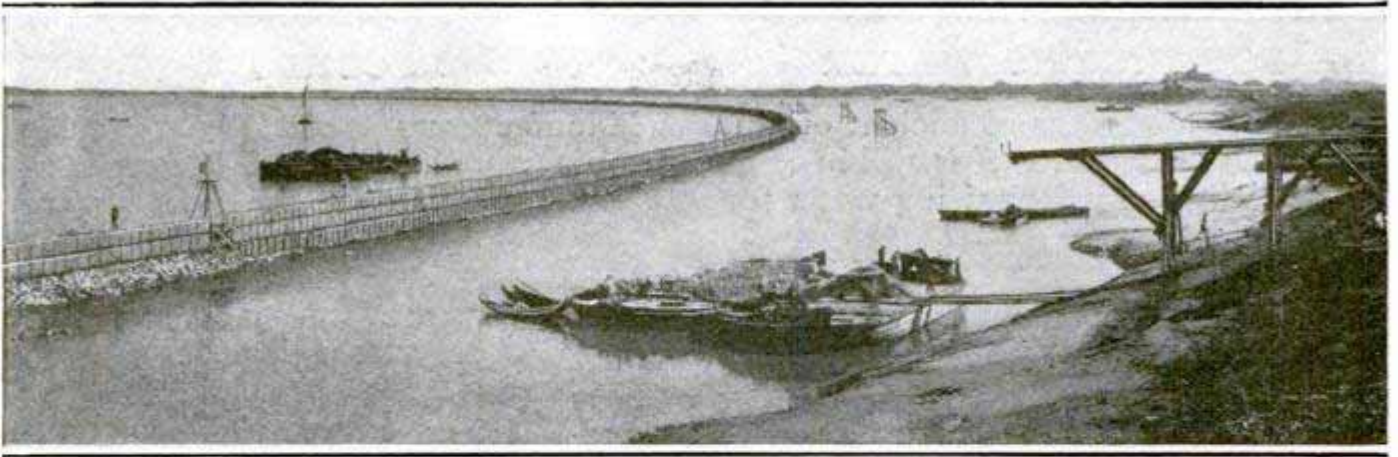
Burma: This Wall, Which Cost About $5,000,000, is About Two Miles Long and Rests Mattresses, Much of It being Built in Water Over 58 Feet Deep
