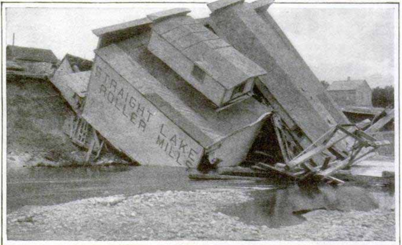
Big Minnesota Roller Mill That Topped into River When Foundations were Undermined by Rush of Water from Breaking Dam
