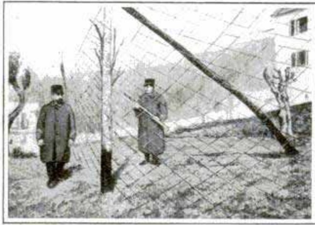
This Wire Fence is Built to Beat the Smugglers
