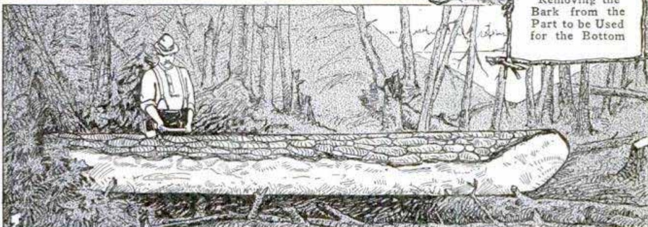
The Log is Lined and the Ends Left Partially Solid for Bulkheads
