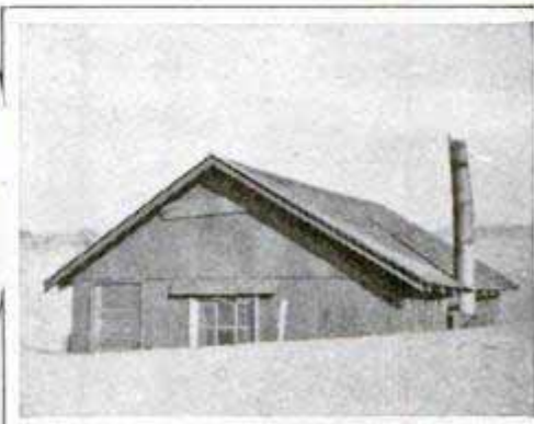
House Overwhelmed with Sand and Abandoned
