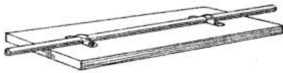
Two Pipe Straps Fastened to a Board over the Conduit Hold It Solidly While Cutting
