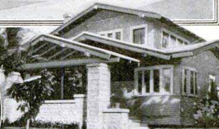
Pillars and Wall Built Up of Concrete Blocks
