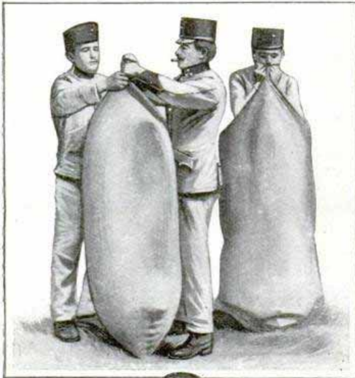
Austrian Soldiers Preparing Pneumatic Pontoons by Inflating Waterproof Bags
