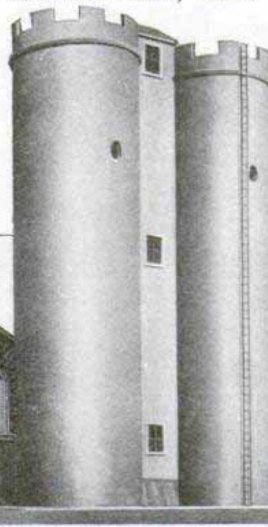
These Twin Silos are Built of Concrete and Stand 72 Ft. High
