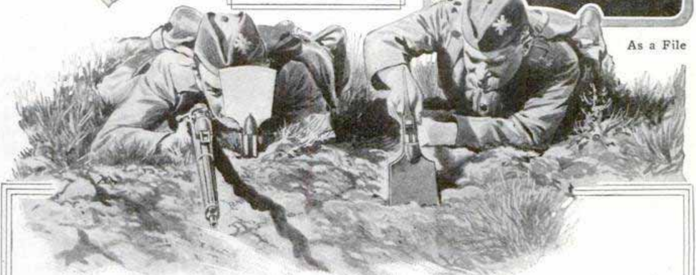
New English Combination Tool in Use as a Trench Digger and Shield
