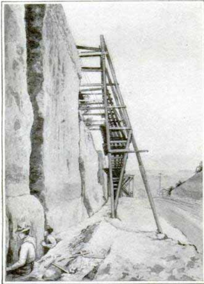
Ingenious Idea for Temporarily Bracing Retaining Wall
