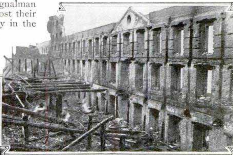
State of Dockyard after Fire
