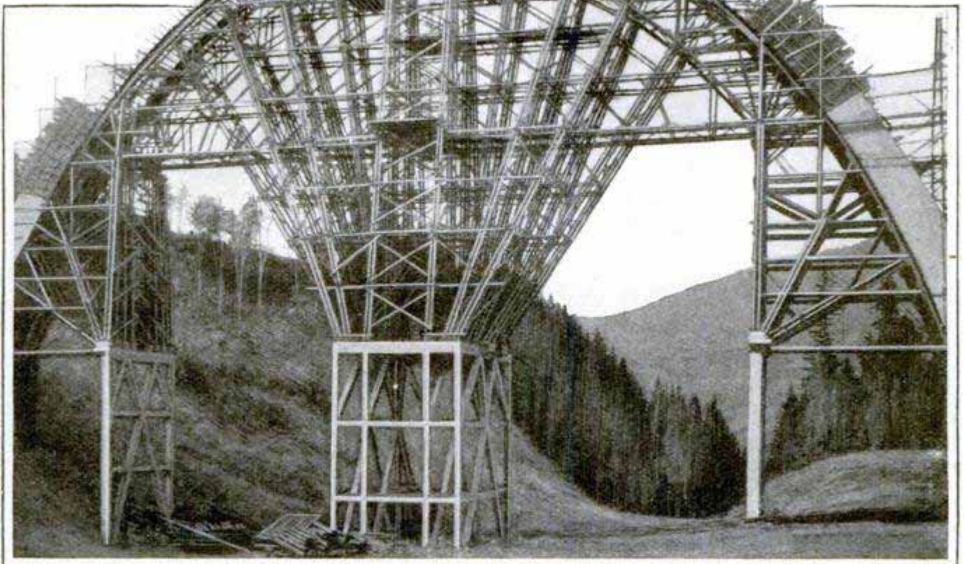
Archway for Viaduct at Langwies, Switzerland
