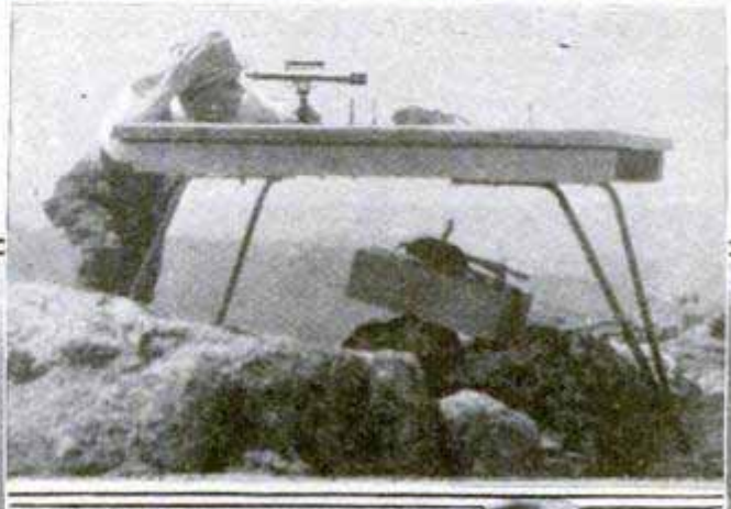
At Right: Lookout Station on Harney Peak, South Dakota. The Iron Legs of the Table are Fixed in Solid Rock
