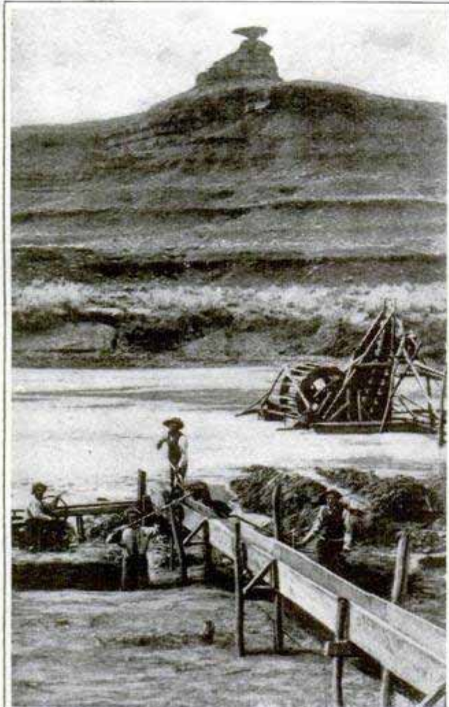
Placer Mining with Sluice; Rocker Operated by Wheel
