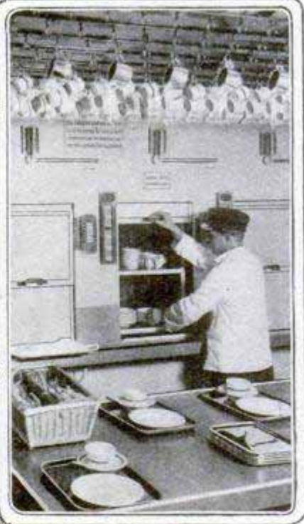
Electric Dumb Waiters Connect All Decks with the Kitchens
