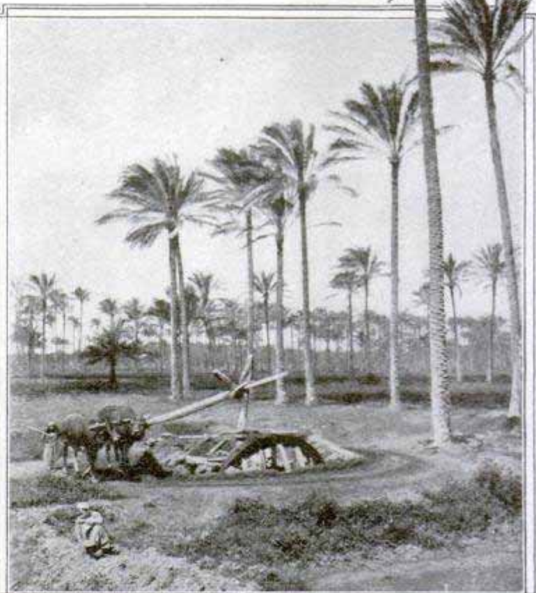
A Sakiya, or Geared Water Wheel of Primitive Type, Such as is Used in Egypt for Irrigating
