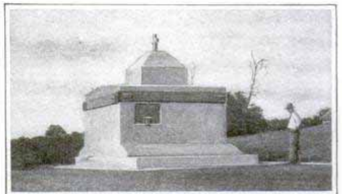
This Oil-Well Cap, of Solid Concrete, was Built in the Form of a Chapel for Protection against Mexican Revolutionists
