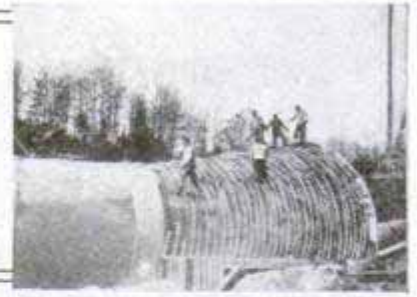
Building One of the Great Venturi Meters Which will Record the Flow of Water
