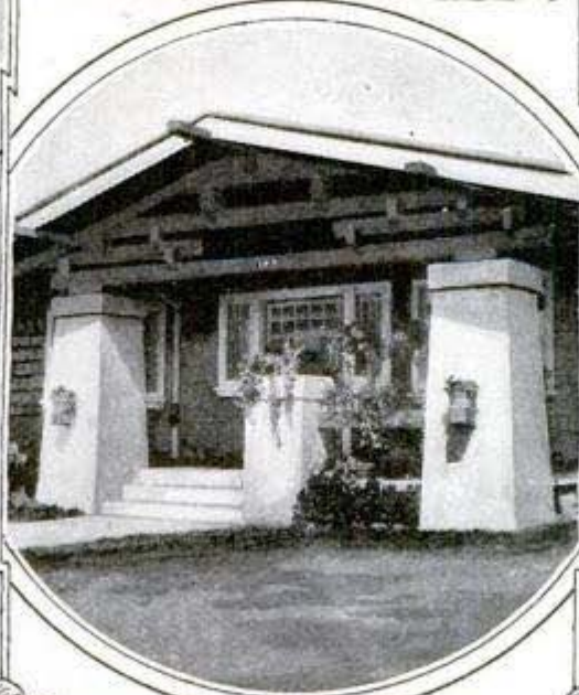
Use of Half-Pillar Relieves Heavy Corner Pillars
