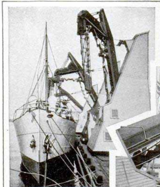
Electric Cranes Dropping Endless Belts into Hold of Steamer
