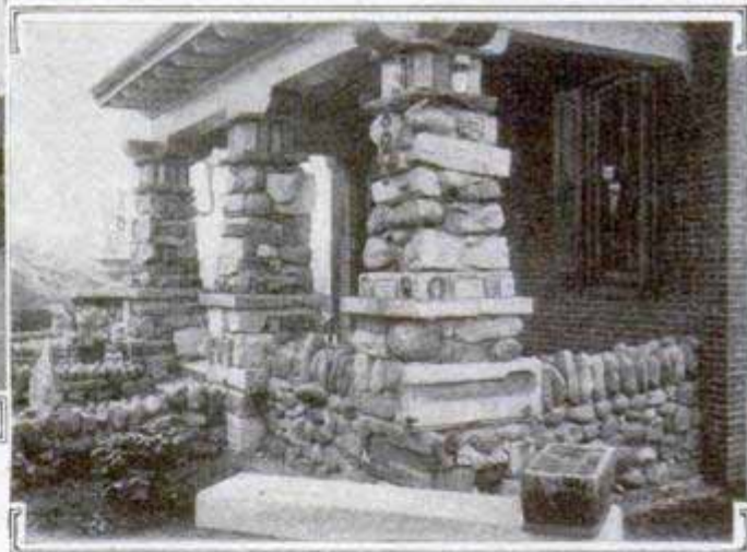
The Front Porch of the "Futurist" House in the Building of Which "Junk" from a Contractor's Yard was Used
