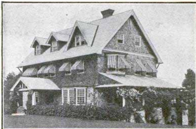
Residence of D. J. Dickson, Wayne, Pa. Covered with J-M Transite Asbestos Shingles. Francis Gogert, Architect, Wayne, Pa.
