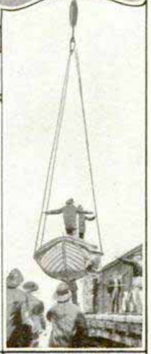
Launching Lifeboat from Railway Train
