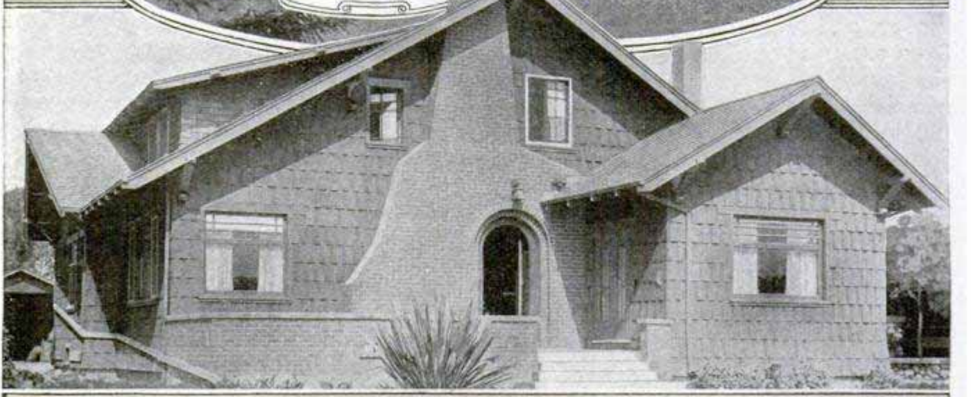
Brick Chimney with Front Doorway of Bungalow Passing through Base
