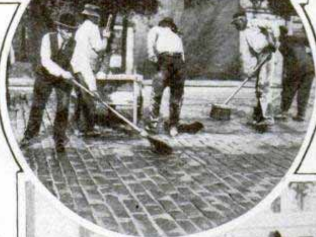
Washing Out the Crevices between Old Blocks
