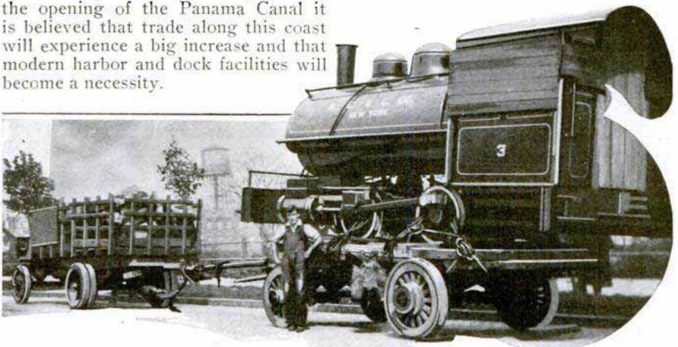
Hydraulic Truck Hauling a Steam Engine across Country, the Load Being 23 Tons beside the Ballast
