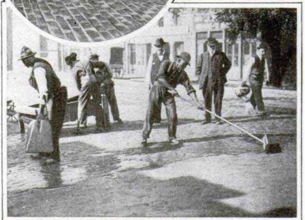
Putting on the Finishing Coat of Cement
