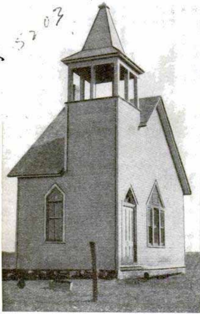
The Front End of a Church Left Standing to Satisfy the Law: The Rest of It was Sawed Off and Moved Away
