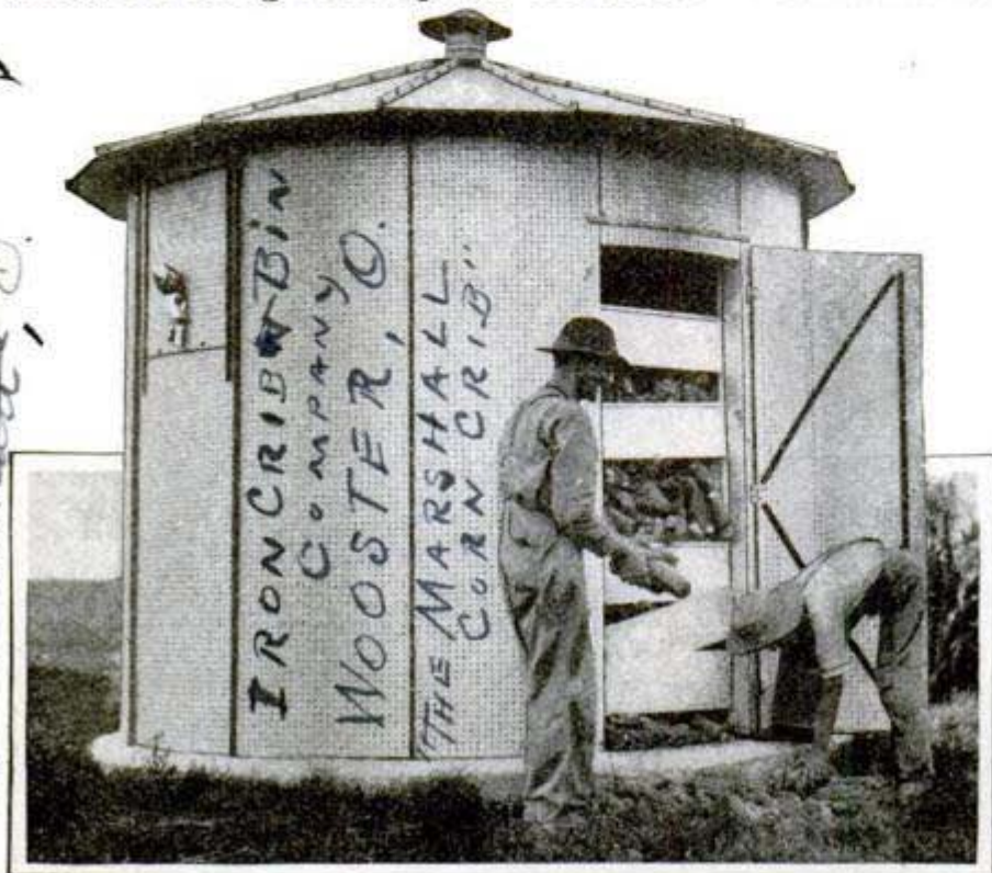
Latest Type of Corncrib Made of Cement and Galvanized Iron
