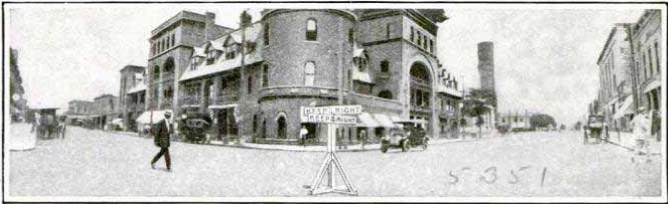
Crossing Sign Warns Drivers to "Keep to the Right"
