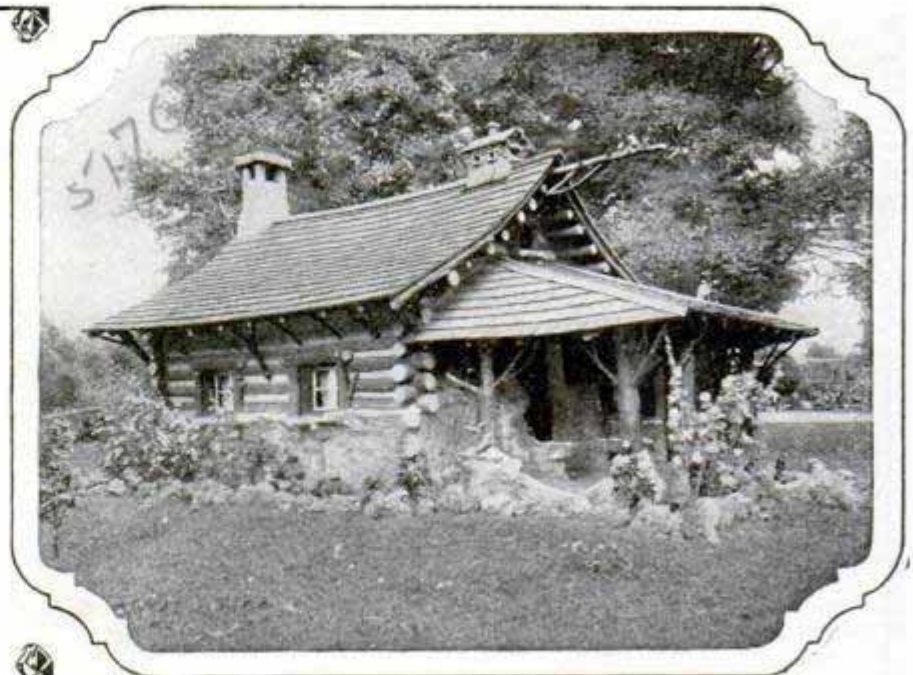
A Concrete Log Cabin in Which the Earliest Form of Home Building is Combined with the Most Modern
