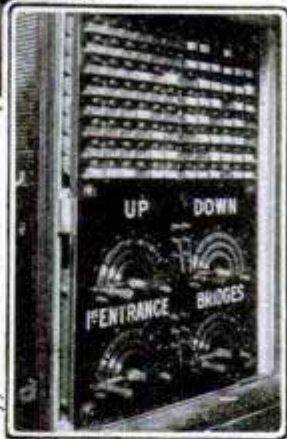
Switches and Cables That Raise and Lower Scenery
