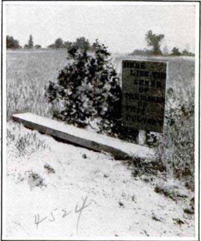
Sign Placed at End of Improperly Finished Culvert
