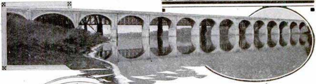
Double-Track Concrete Bridge, 1,445 Ft. Long, across the Delaware River at Yardley, Pa., Old Wrought-Iron Bridge behind It; Above, Top View of New Bridge Showing Concrete Shell Before It was Filled with Rock and Dirt and Old Iron Bridge beside It
