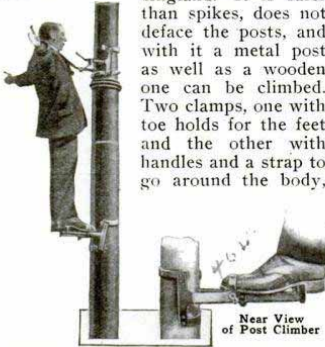
This Man is Standing on One of the New Post Climbers Clinging to an Iron Lamp-Post
