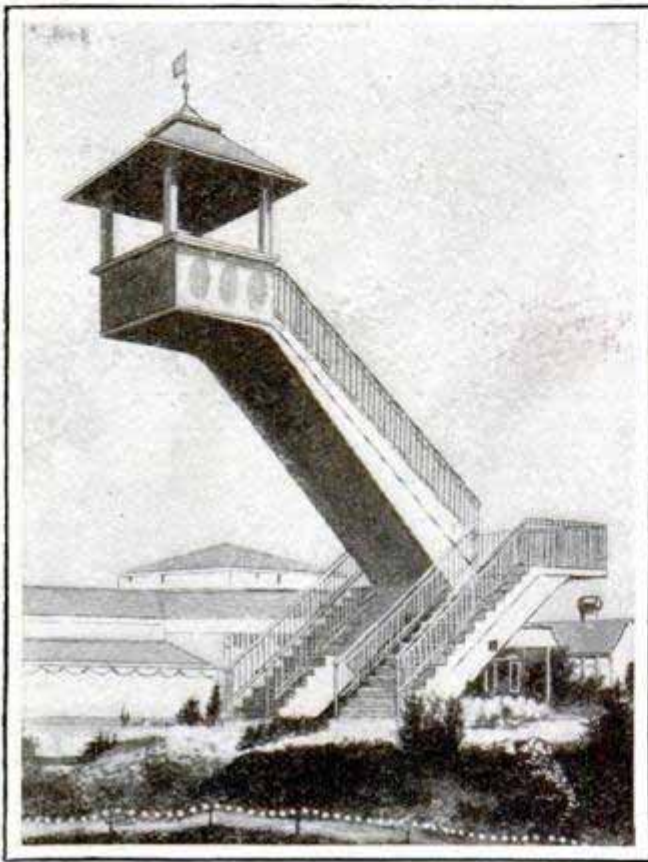
Cantilever Tower Built to Demonstrate Qualities of Reinforced Concrete
