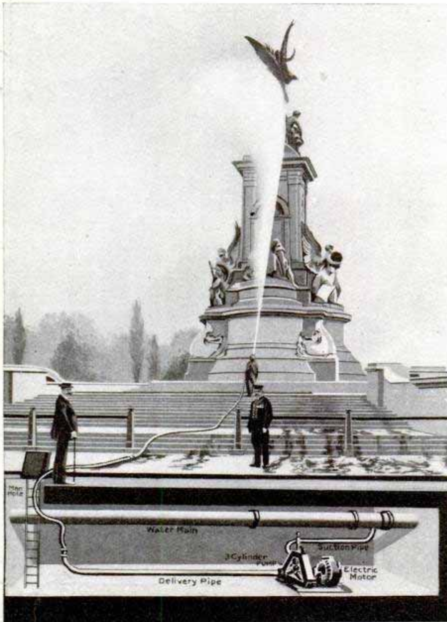
Apparatus That is Used to Clean the Victoria Memorial Monument, London
