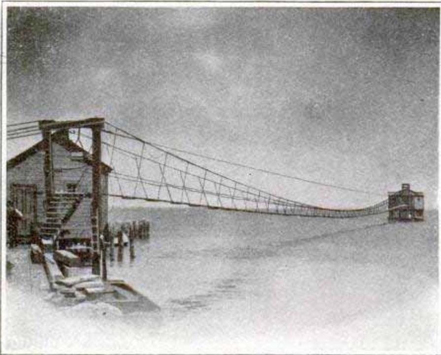
Storage House in Which Dynamite is Kept at Safe Distance Off Shore
