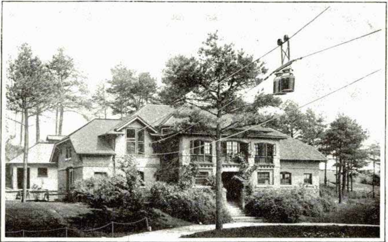
Aerial Cableway for Transporting Milk Cans on a Large Dairy Farm
