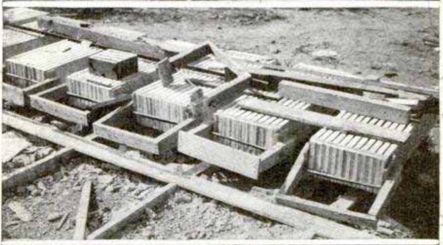
Top View: A Pile of Boards and Timbers Reproduced in Concrete; Center View: A Reinforced-Concrete House Put Together Just Like a Frame Structure Except That All Its Parts are Made of Concrete; Bottom View: Molds for Making Cement Clapboards
