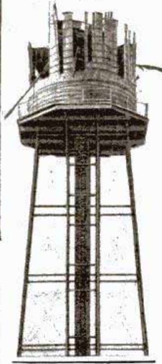
City Water Tank Which Burst Because of Rusted Hoops
