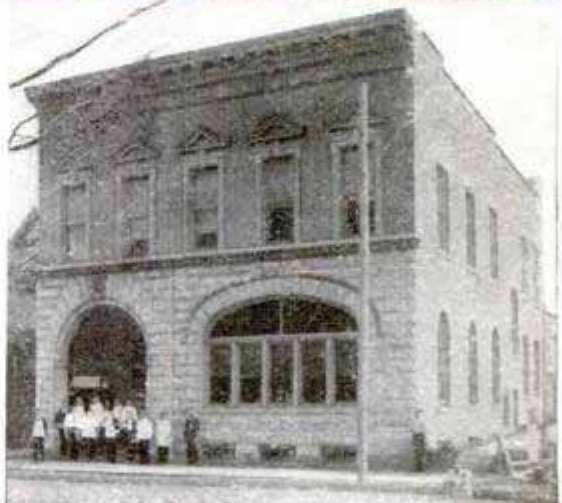
The Outside of Their Manual-Training Quarters
