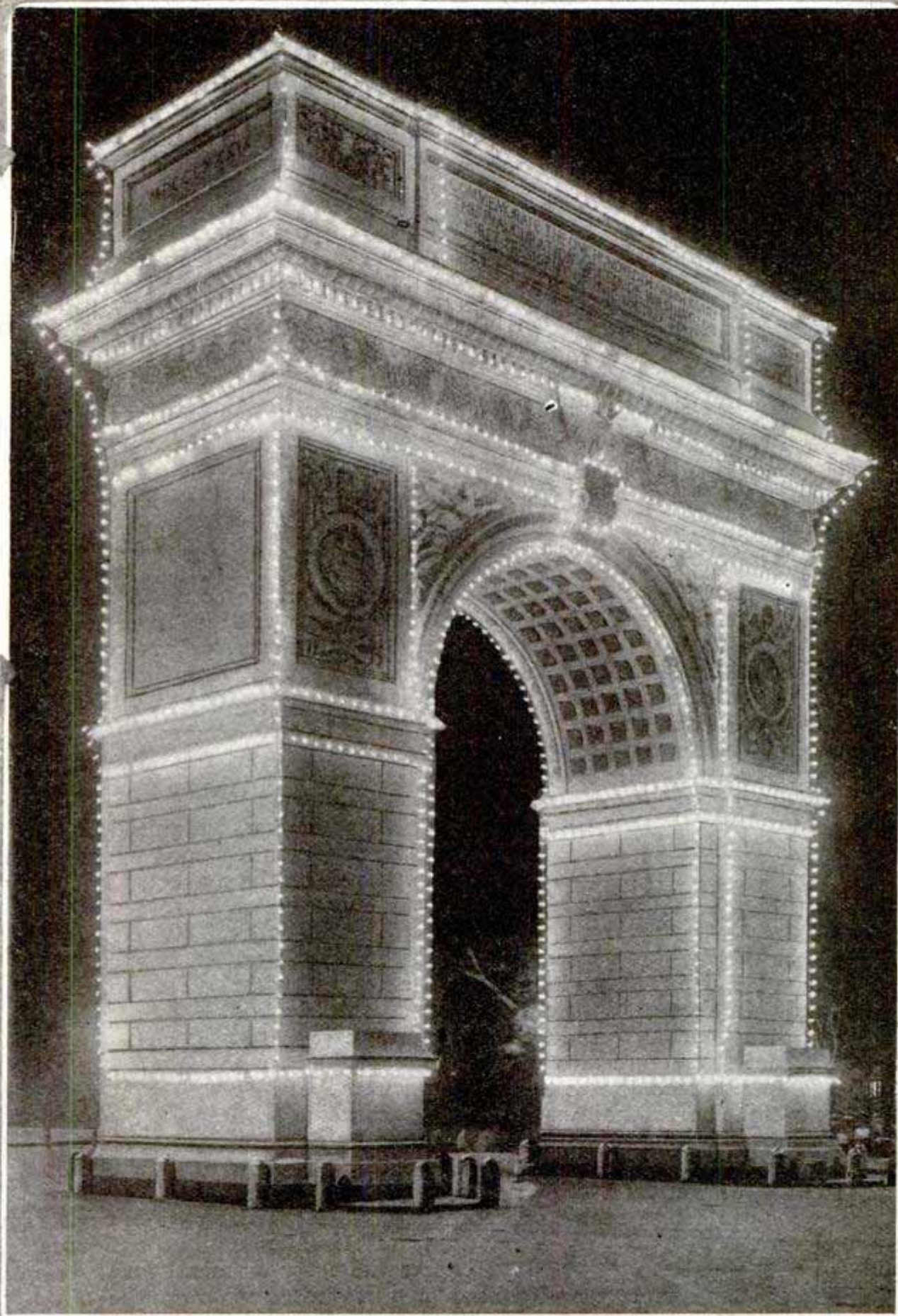
The Beautiful Effect Produced by Clusters and Strings of Electric Lights on Washington Arch, Which Guards the Fifth Avenue Entrance of Washington Square, New York City: Every Line of Light to the Top of the Entablature, Over 65 Ft. in the Air, Stands Out Clear-Cut in the Darkness
