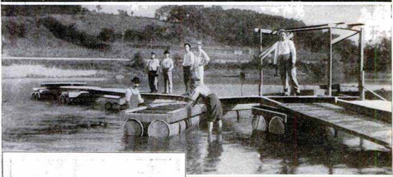
Swinging the Barrel Pontoons into Position
