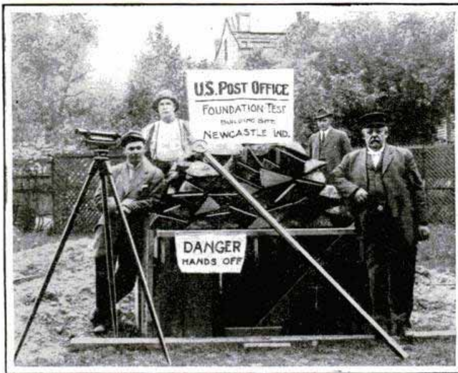
Getting the Bearing Power of the Clay Underlying a Foundation
