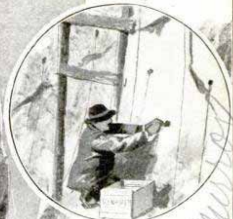
Placing the Dynamite Cartridges
