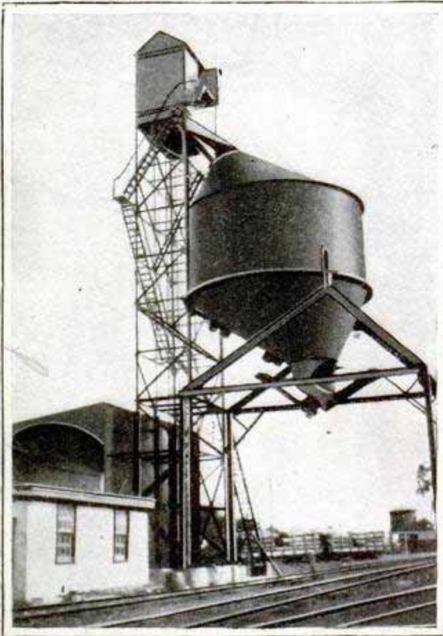
Modern Coaling Plant Hoists and Delivers Coal Automatically
