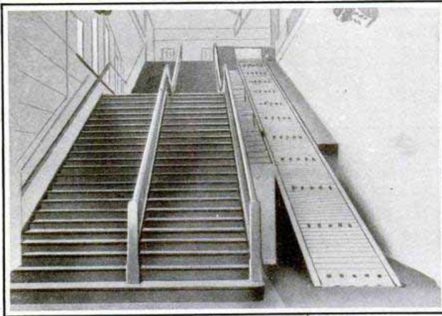
Baggage Conveyor and Stairways on One of the Transatlantic Piers
