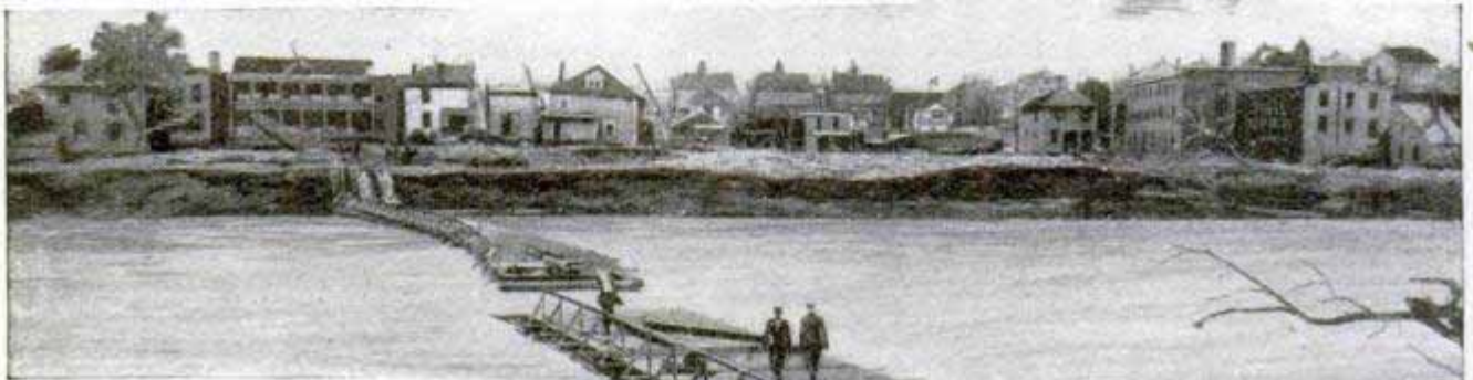
Troops of the Ohio National Guard Built a Pontoon Bridge at Hamilton to Enable Wagons with Food and Clothing to Enter the City
