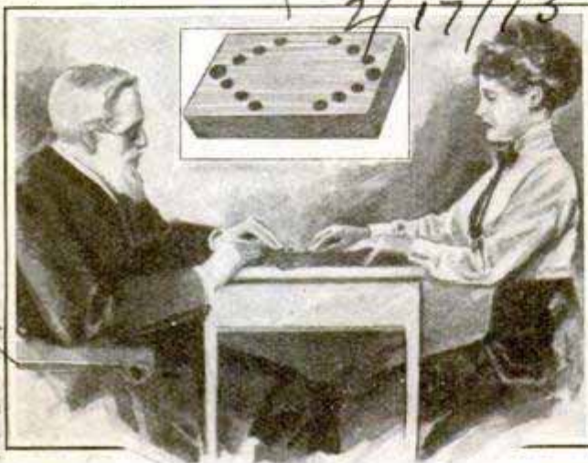
Simple, Practical Device by Means of Which Persons Both Blind and Deaf can Carry on a Conversation
