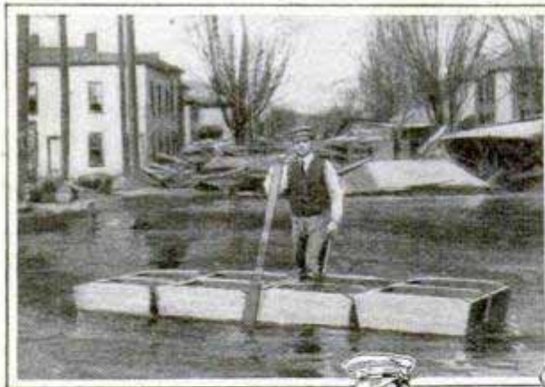
Rescue Boat Made of Four Washing Machines Nailed Together
