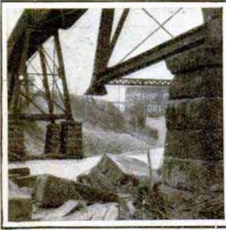
Bridge Pier Washed Out at Richmond, Ind.
