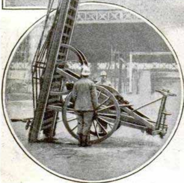
A 65-Ft. Ladder Ready to be Raised
