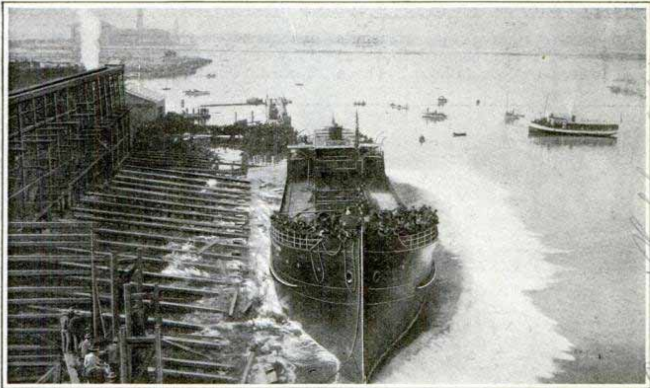
Dropping an Ocean Steamship into the Water Broadside
