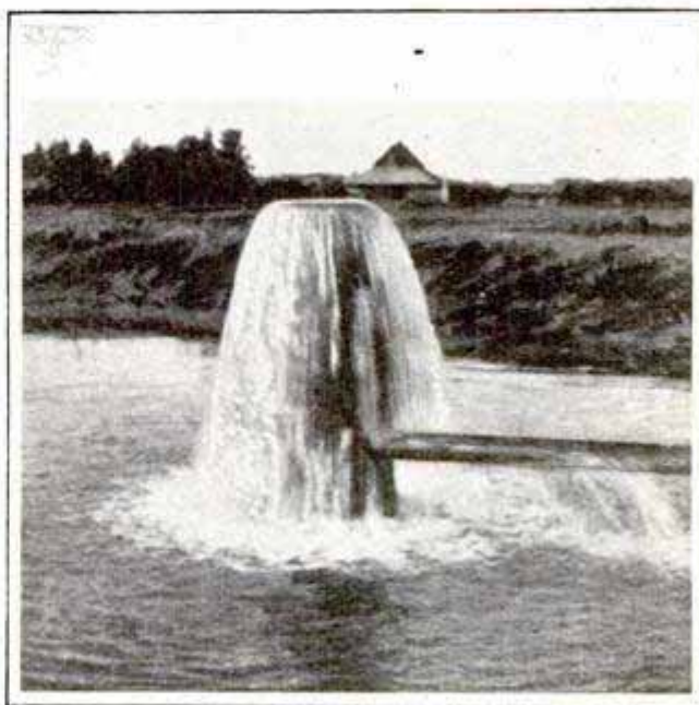
This Water Well Gives Off Sufficient Natural Gas to Run the Pumping Engine
