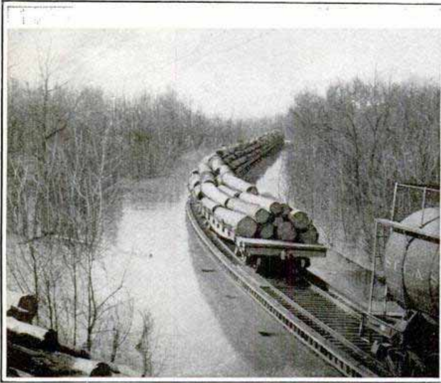
Long Train of Logs Prevents Track from being Carried Away by Floods
