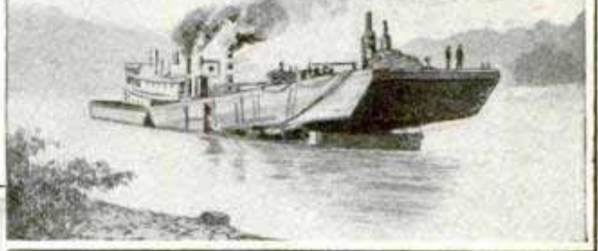
Manner in Which the Barge for the Monongahela Bridge had to be Floated to Get It through the Locks
