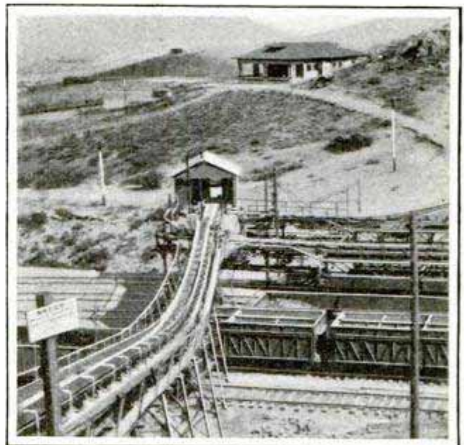
Ore Conveyor Which Automatically Makes Up Carload Mixture of Various Quality Ores
