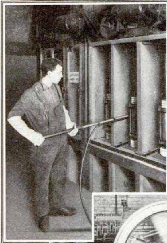
All Cables, Switches and the Like must be Discharged to Ground
