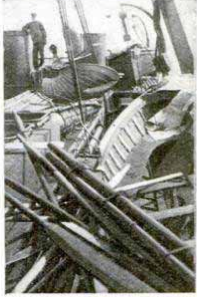
Wreckage on the Starboard Side of the Collier
