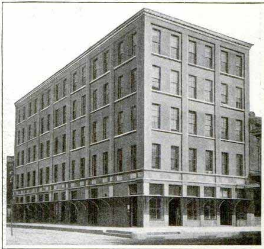
Large Galveston Office Building Constructed of Oyster-Shell Concrete
