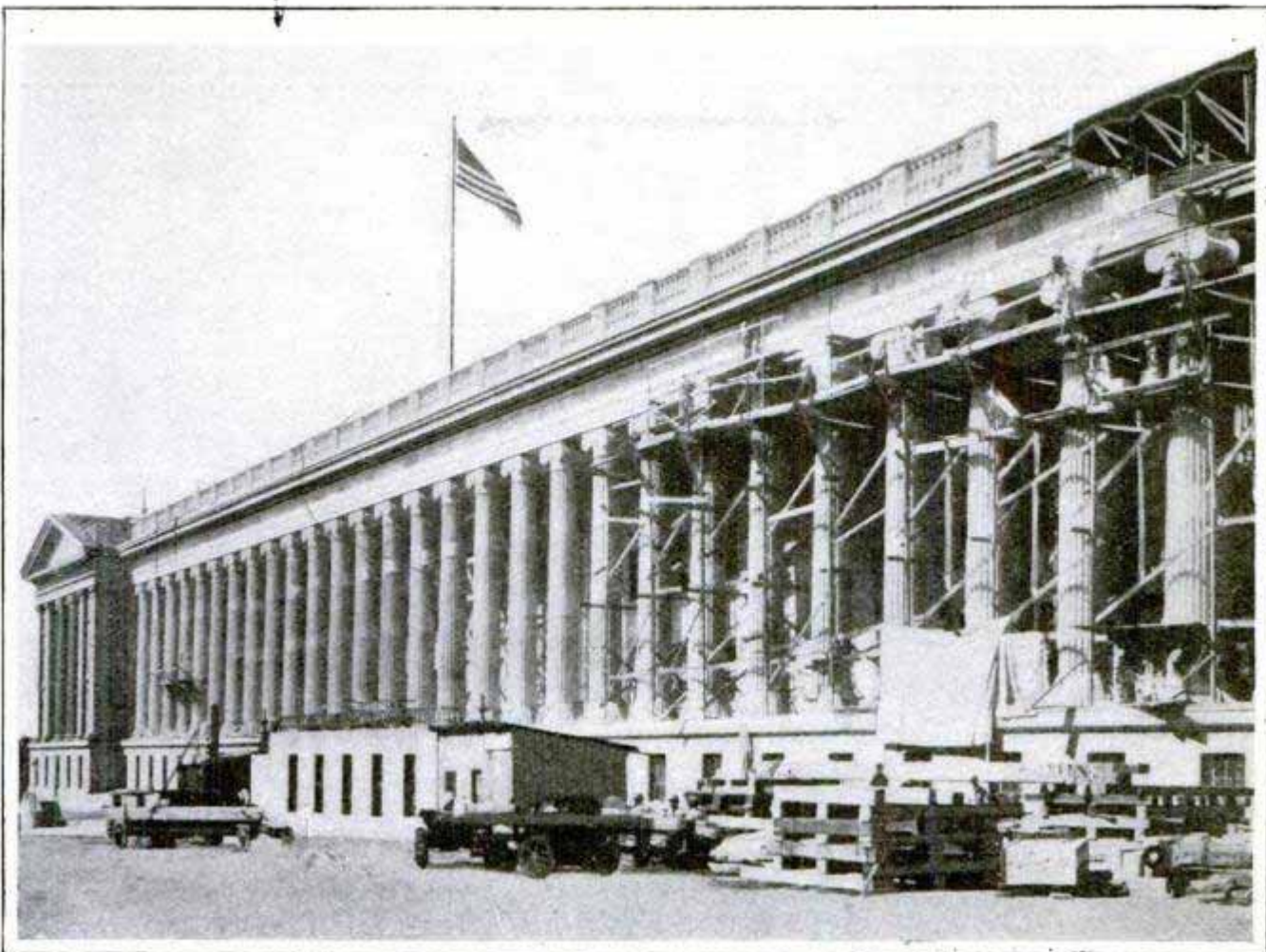
Replacing the Sandstone Columns of the U. S. Treasury with Granite That will Last 10,000 Years
