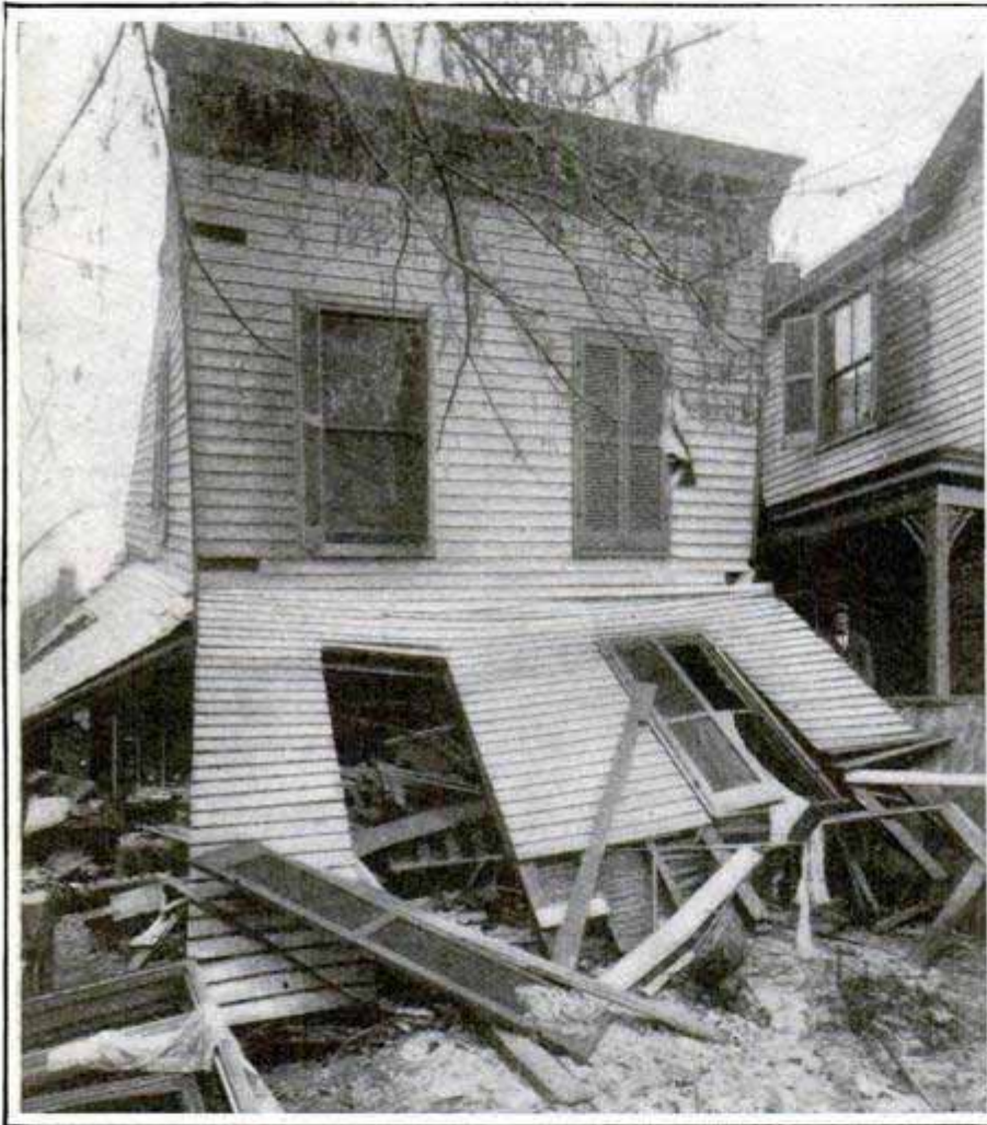
Natural-Gas Explosion Wrecked This Cincinnati House
