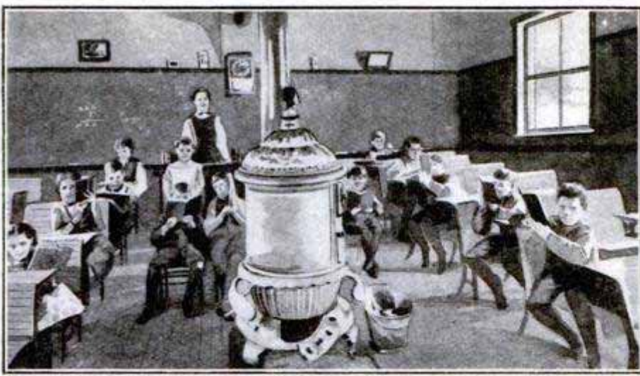
An Example of Faulty Heating. The Stove should be Jacketed, as Shown at the Right, and should be Placed in a Corner Instead of in the Center of the Room
