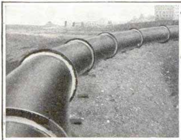
Curved Section of Boston's Electric Mail Tube
