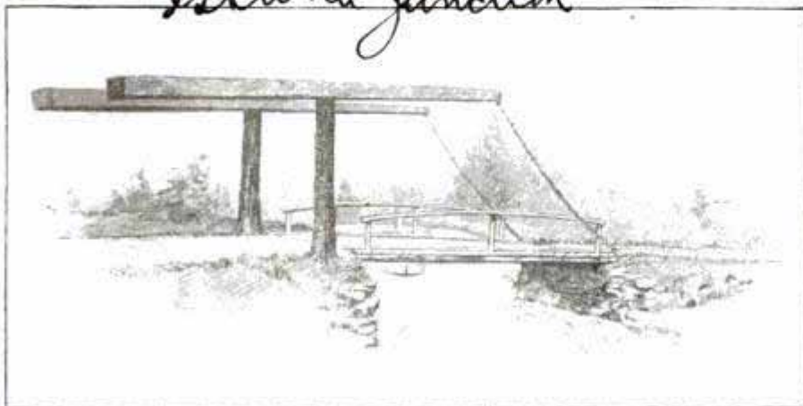
Balanced-Beam Drawbridge Which may be Lifted by Hand
