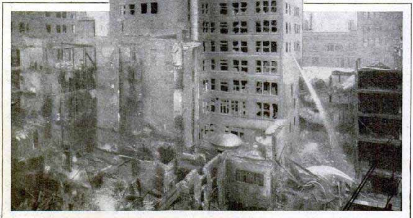
Cincinnati Skyscraper Claimed to be Fireproof, Guttled by Fire Which Started in Adjoining Hotel
