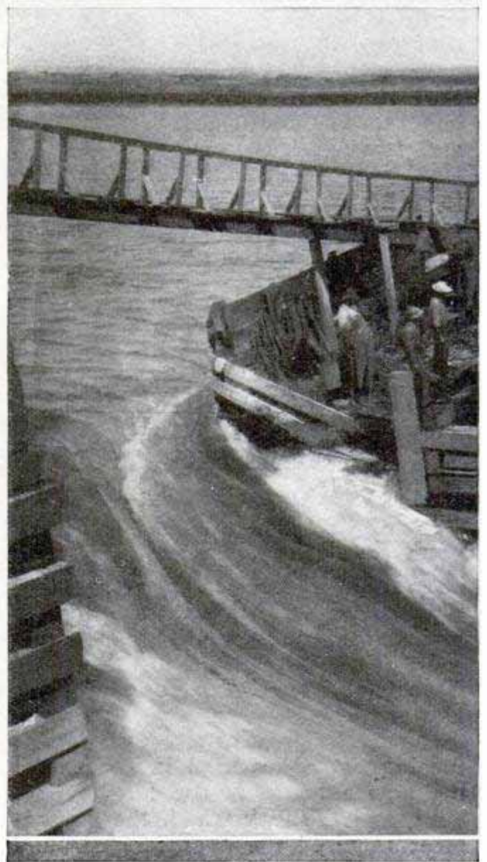
Upper Left-Hand View—Looking North through the Big Lock as It Appeared Last November. Lower Left—the Million-Pound Gates for the Lower End of the Lock. This Gate Contains Airtight Chambers, to Prevent Lower Right-Hand View—The Rush of Water through This Uncompleted Section of Cofferdam
