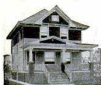
Design No. 50 $872 Eight Rooms and Bath, very attractive Exterior; Five Closets, Airy Balcony. Size 28 ft. by 28 ft.
