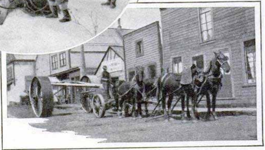
A "Spider" Used for Transporting Heavy Machinery in the Vicinity of Nome
