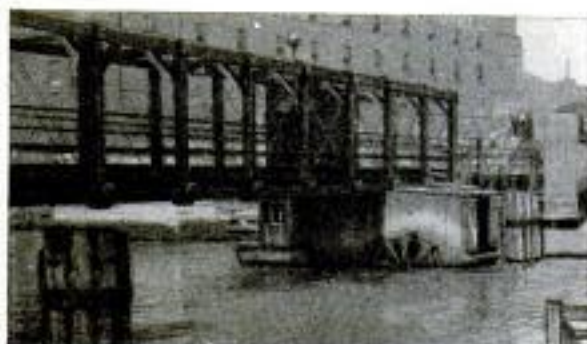
Views of the Curious Draw Bridge over the Chicago River. Showing the Bridge Closed, the Scow Which Turns the Draw, and the Method Followed in Opening It
