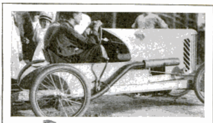
The "Gila Monster," Built for Racing with Minimum of Weight on the Rear Wheels
