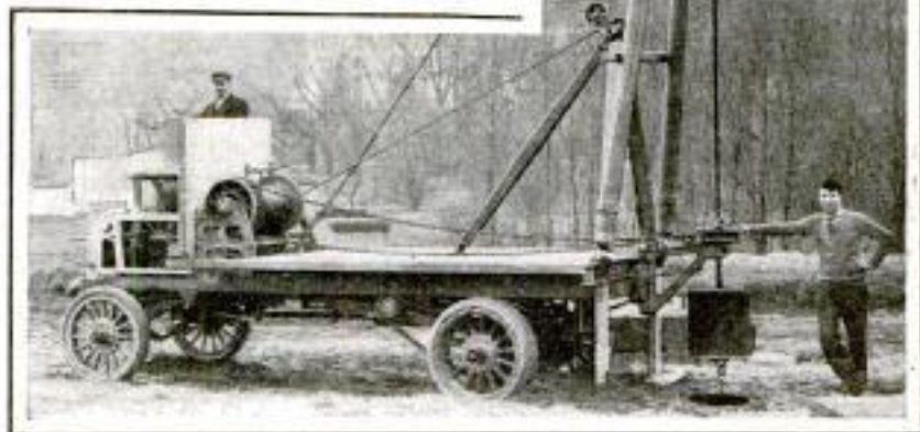
Apparatus Which Digs Post Holes and Lifts and Sets the Poles in Position
