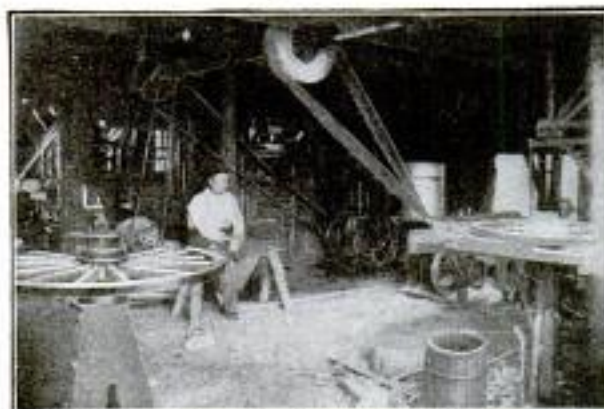
I H C Engine in Use in Blacksmith Shop
