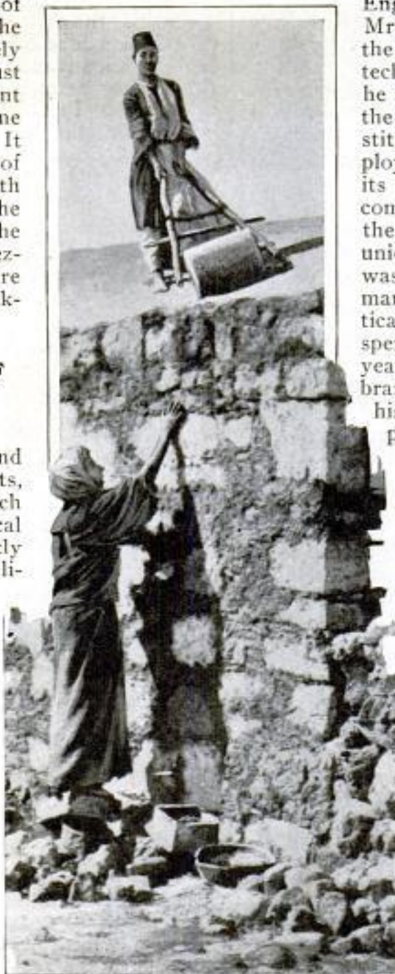
A Native of Palestine Rolling His Dirt Roof to Make It Rain-Proof
