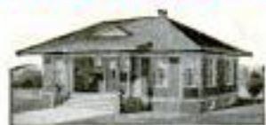
Design No. 117 $635 Six Rooms and Bath. A Modern Bungalow, Excellent Interior. Size, 39 feet, 6 inches by 27 feet.
