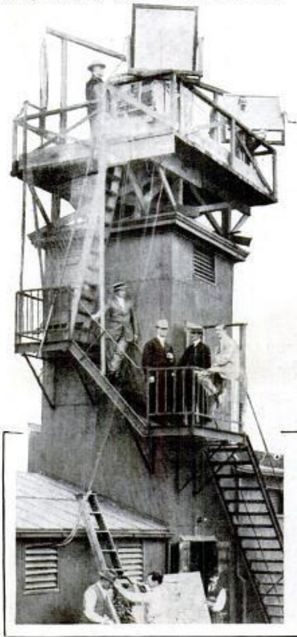
Searchlight Color-Flashing Apparatus on High Baltimore Building
