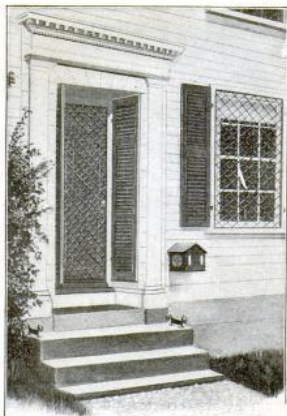
Flexible Wire Screen Placed Inside Window and Door Casings, so as to Obtain Protection while Windows and Doors are Open
