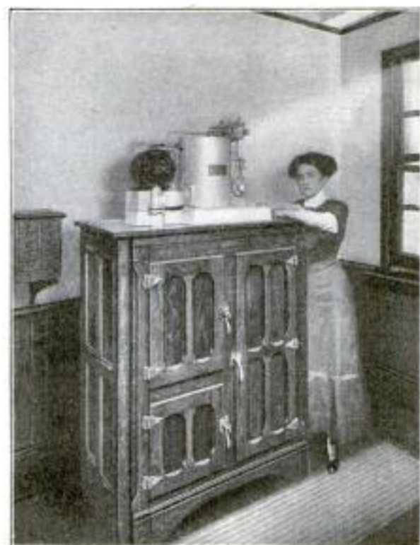
The Electric Ice-Making and Refrigerating Machine Mounted on the Top of the Ordinary House Refrigerator
