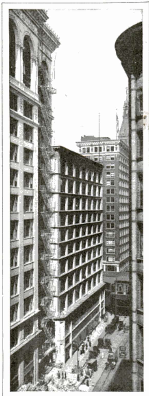
Recessed Fire Escape on the Face of Skyscraper Building; an Architectural Idea Which Eliminates Much of the Ugliness of Such Escapes
