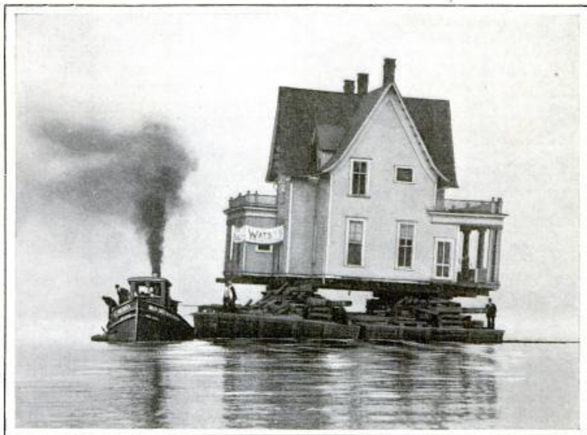
Large Two-Story House Moved on Scows Three Miles along the Shore of Lake Michigan
