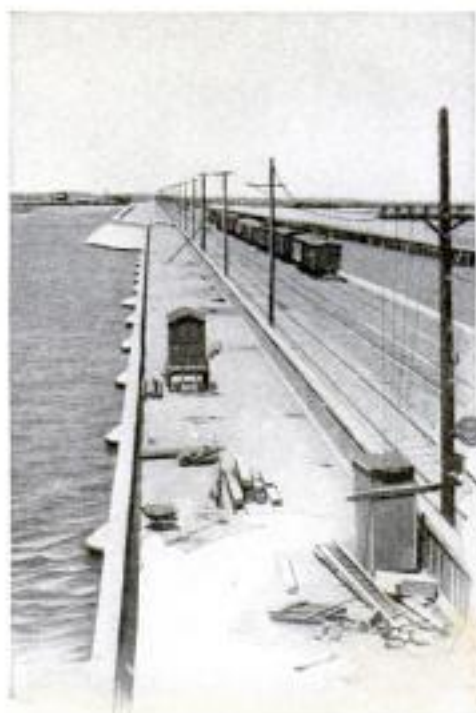
View of the Surface of the New $2,000,000 Causeway
