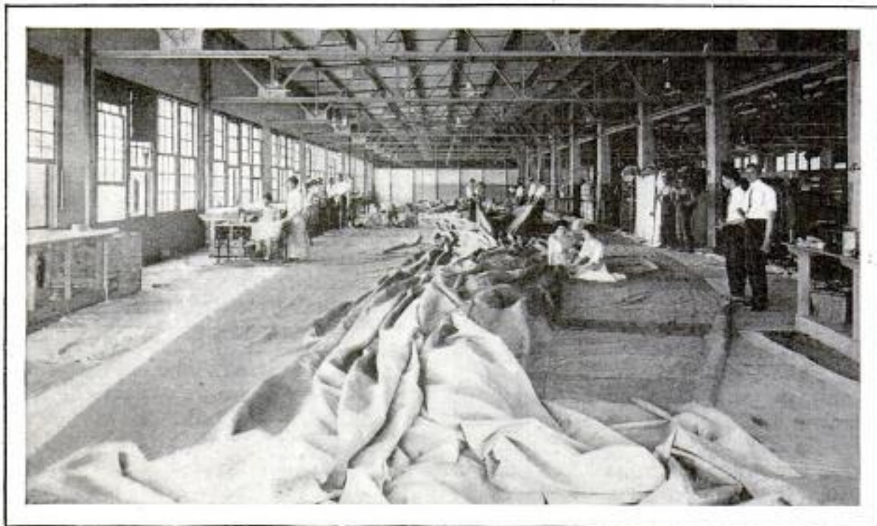
Constructing the Envelope of the Ill-Fated Airship in the Factory at Akron, Ohio. It was the Largest Ever Made in the United States
