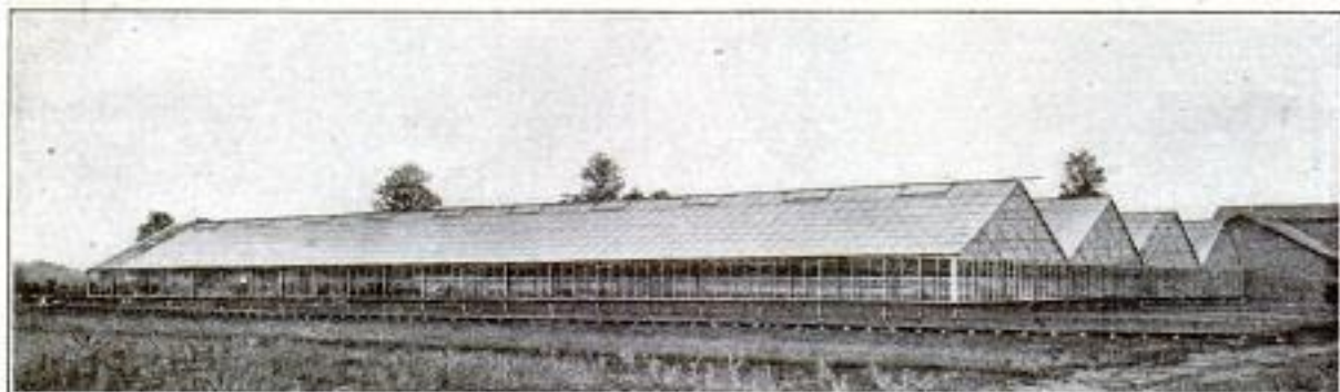
A Complete View of the Wheeled Greenhouse, Which Covers an Area of Almost 25,000 Square Feet
