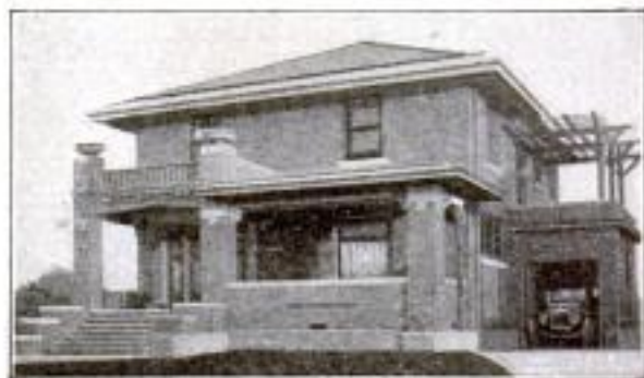
The Porte-Cochere Garage of a Dallas, Texas, Physician
