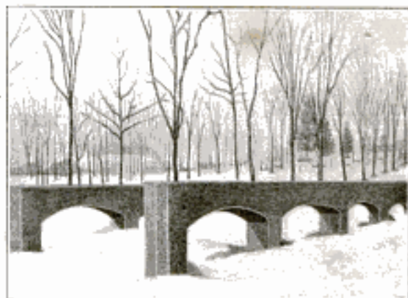
Rows of Concrete Arches Erected in Low Ground of an Old Cemetery at Portsmouth, N. H., as Grave-stone Foundations
