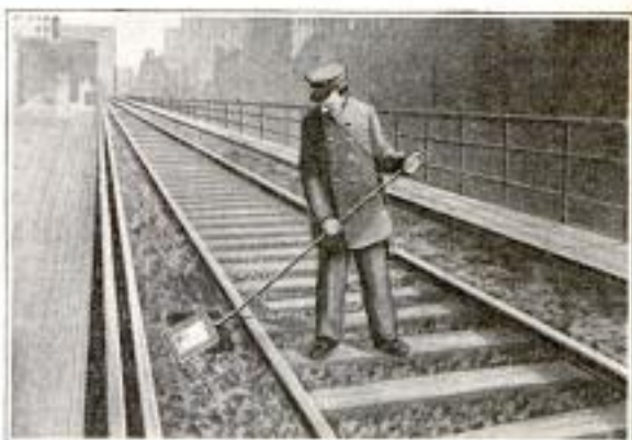
Examining the Cable of an Electric Railway in Germany by Means of a Looking Glass on a Stick
