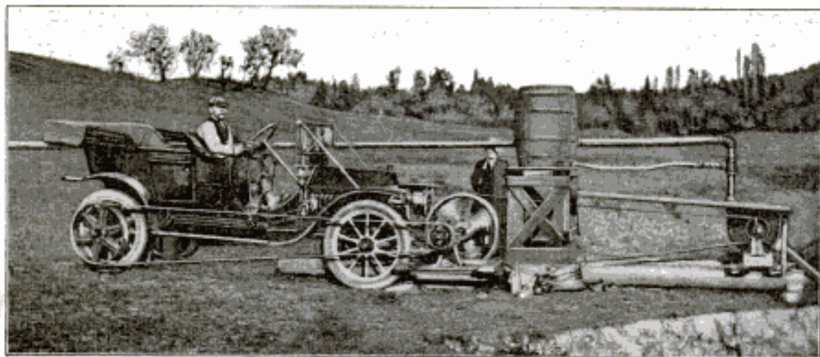
An Automobile-Driven Rotary Pump Used to Fill an Irrigation Reservoir on a California Ranch
