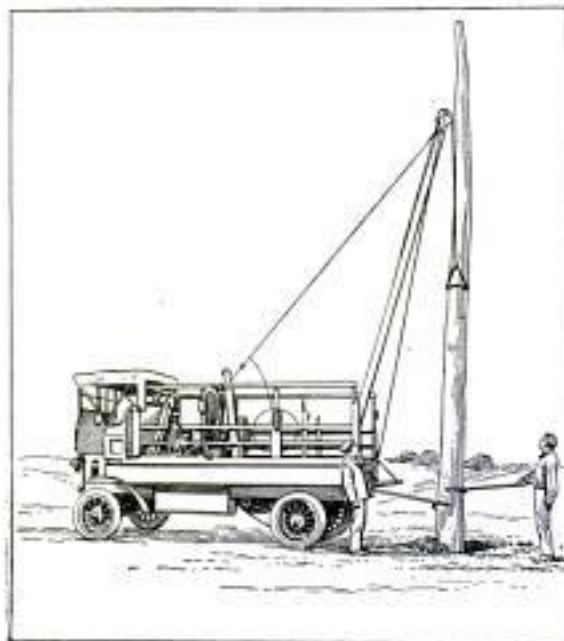
Courtesy the Motor World Setting a Telephone Pole in Place by Means of a Motor Truck
