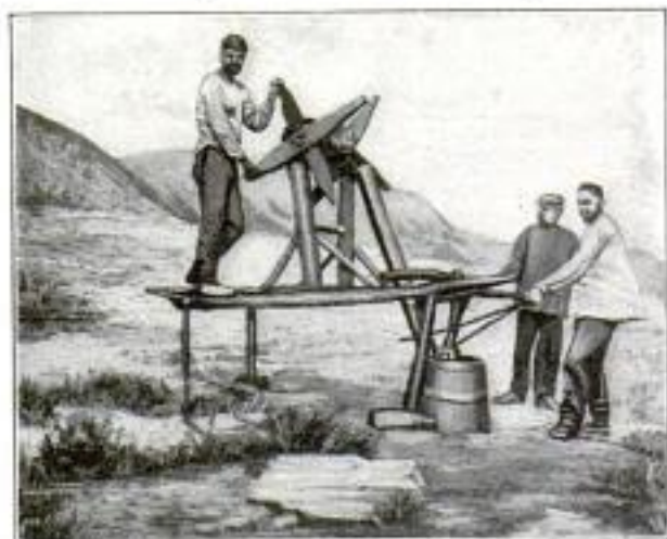
A Primitive Method of Extracting Oil Still in Use in Russia
