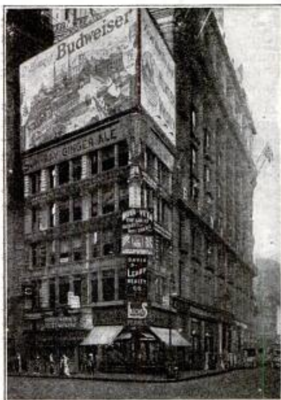
The Sign Privileges of This Building are Valued at $60,000 a Year, Which is $20,000 a Year More than the Building is Leased For
