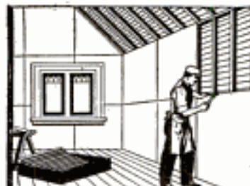
Applying Wall Board to Studding
