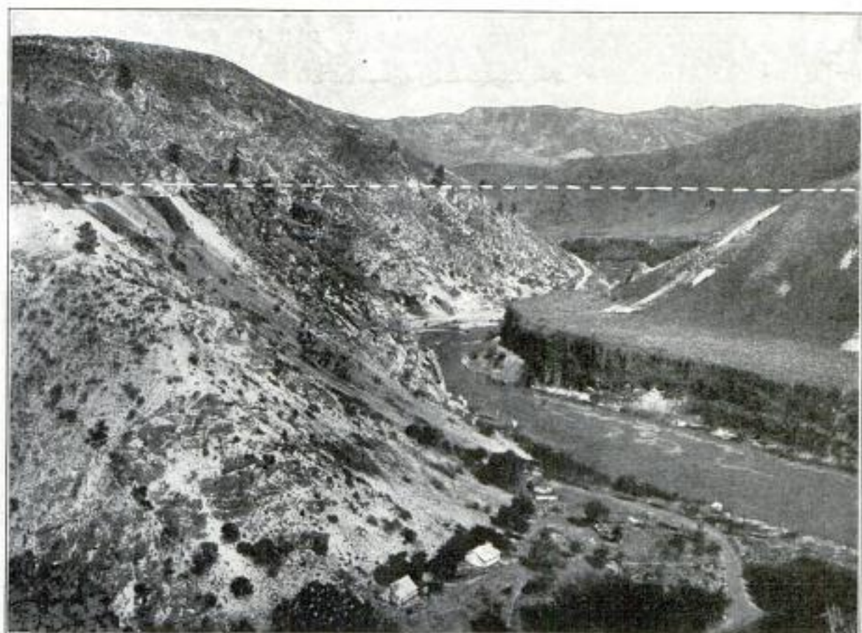
The Site of the Arrowrock-Boise Dam, to Be the Highest in the World. White Line Indicates Height of Dam, 351 Feet above the River
