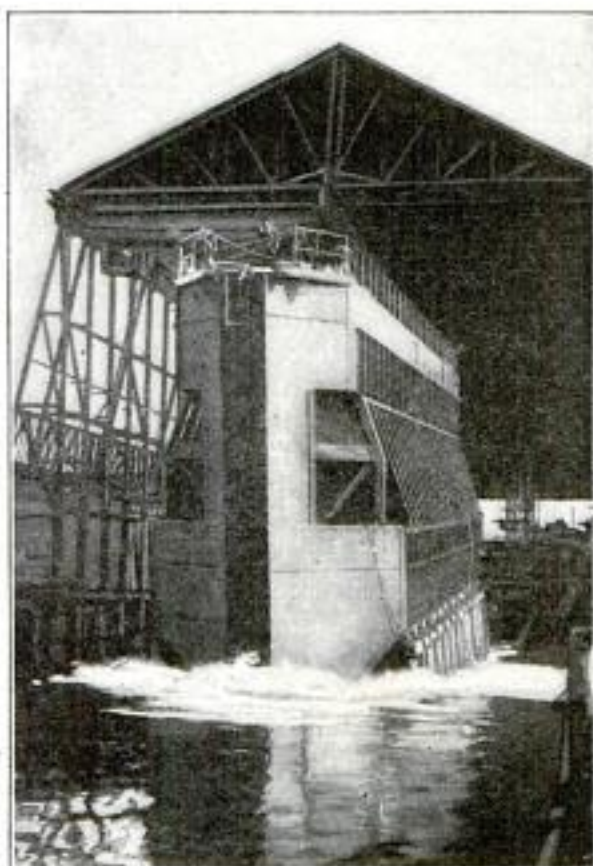
Launching of the 127-Ft. Gate for the New Drydock of the Bremerton Navy Yard
