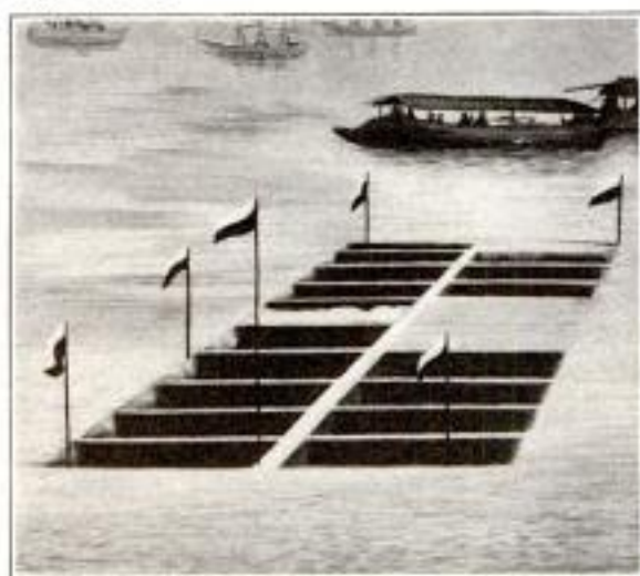
Sinking Reinforced-Concrete Caissons in Kobe Harbor, Japan
