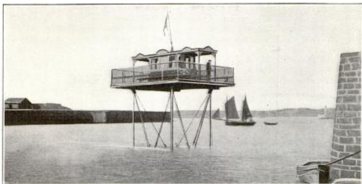
French Transporter Bridge Drawn Back and Forth on a Railway 22 Ft. under Water, the Drawing Power Being an Electric Motor
