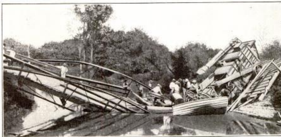
Bridge near North Platte, Neb., Which Collapsed with the Weight of a Threshing Machine and Engine
