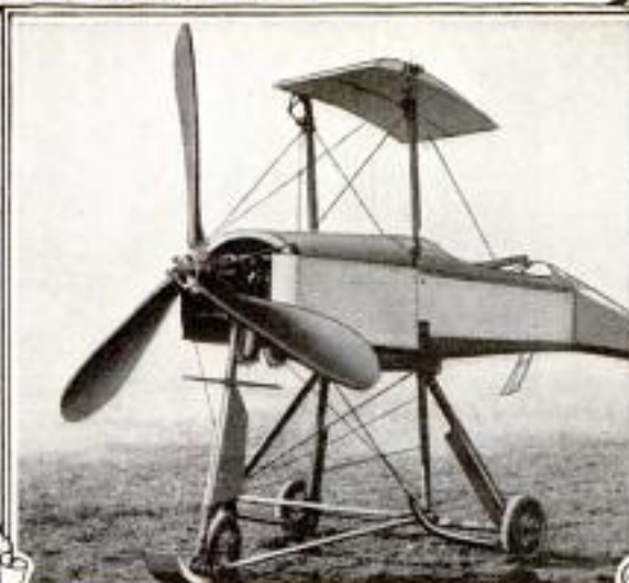
Three-Bladed Shock-Resisting Propeller on Frame of Breguet Aeroplane
