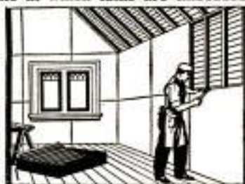
Applying Wall Board to Studling
