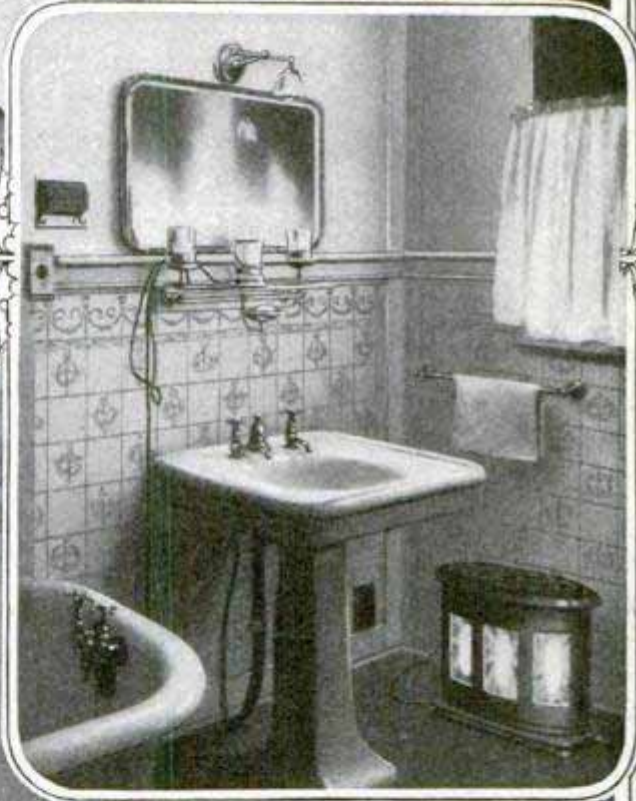
In Bathroom are the Luminous Radiator and Water Heater for Shaving
