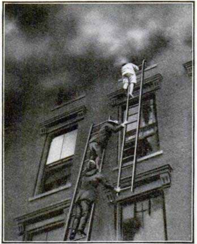
To Safety at Last by Means of a Light Scaling Ladder
