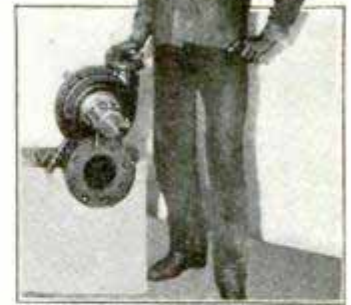
A Complete 110-Hp. Turbine
