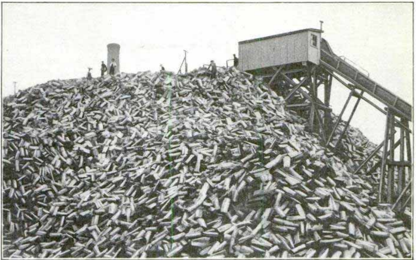
The Pile of Wood of Which This Illustration Shows a Section Will, Mixed with Soda Pulp, Make About 50,000,000 Lb. of Paper
