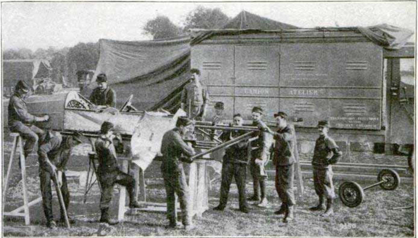
The French Aerial Corps' Traveling Machine Shop for Aeroplane-Construction Repair Work
