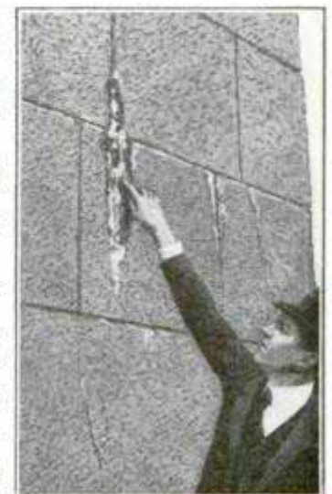
Deposit of Structural Material near Base
