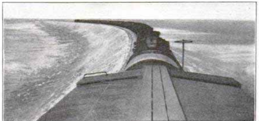
A tank train as it appears from the roof of the caboose at the tail end, is shown in the accompanying illustration. The tank cars contain water hauled from Willard, New Mexico, to Vaughn for railroad use.
