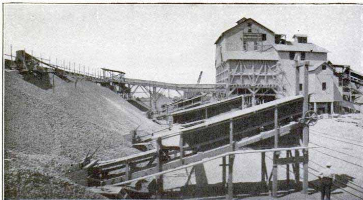
A Rock-Crushing Plant That Breaks Up the Stones after
