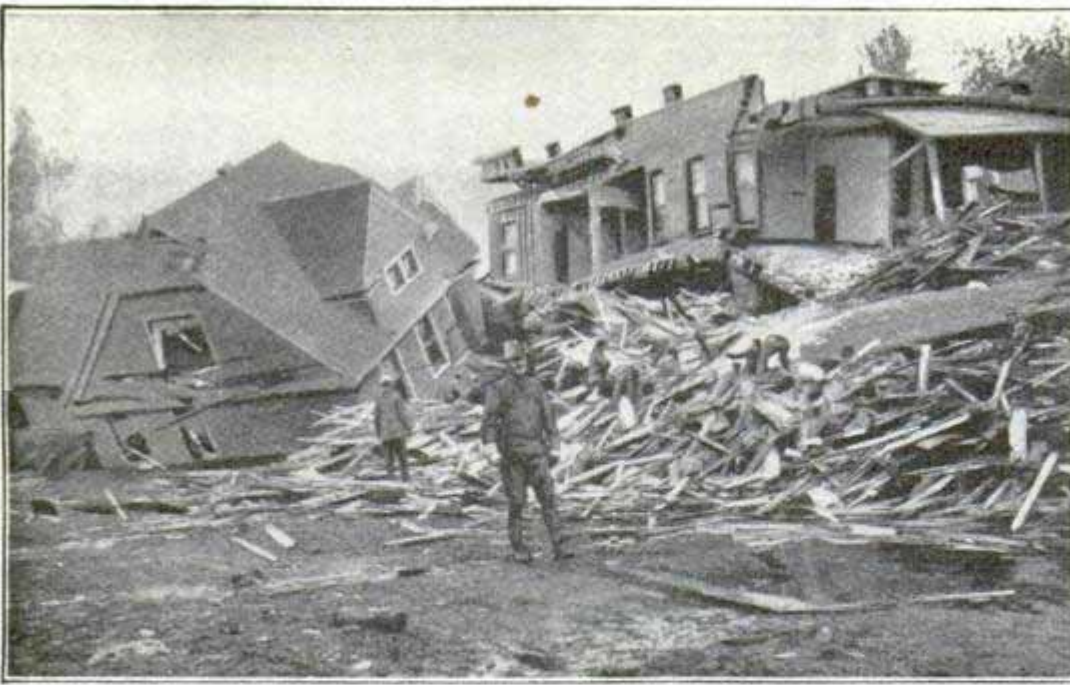
The Wrecks of Light Frame Buildings Were Piled against Brick and More Substantial Structures. Photo Copyright by Pictorial News Co.
