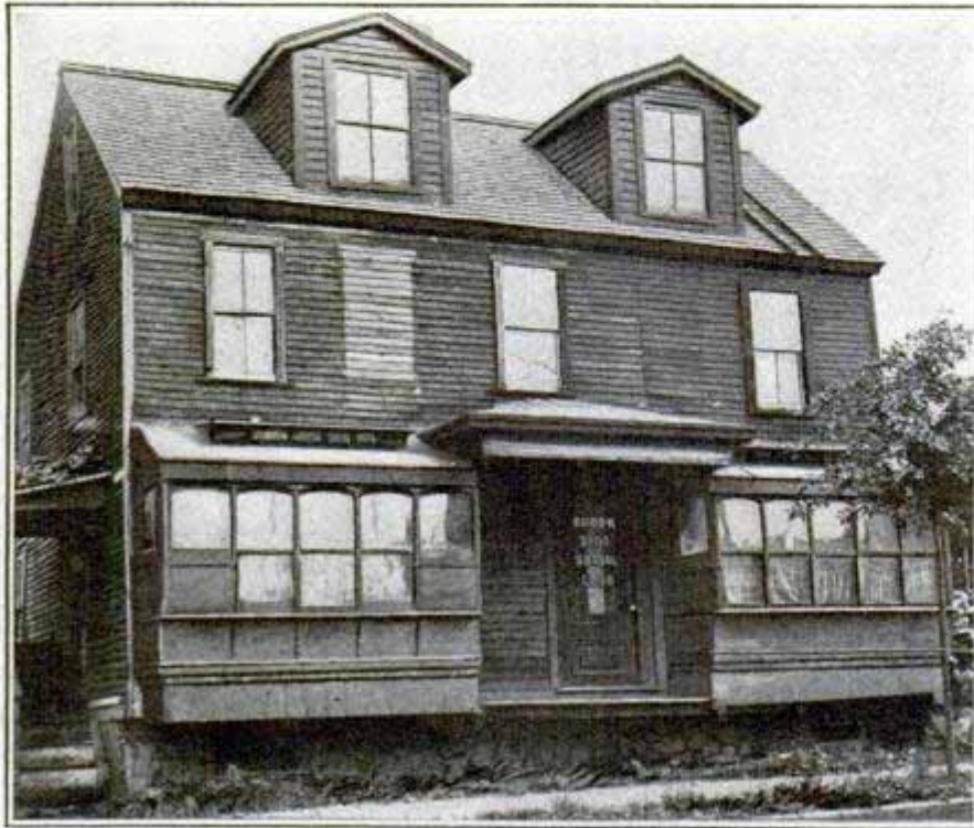
This Curious Architecture is the Result of Additions to a Street Car from Time to Time
