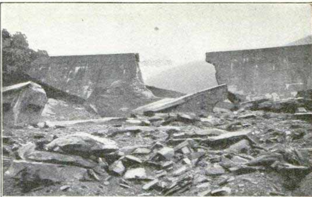
Where the Flood Started. View of the Wrecked Dam from the Side toward the Town. Photo Copyright by Pictorial News Co.
