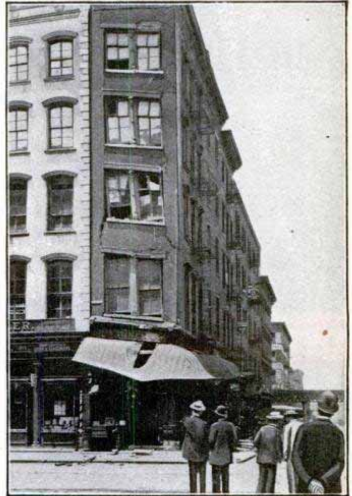
Partial Collapse Due to the Old Type of Supporting-Column Heads
