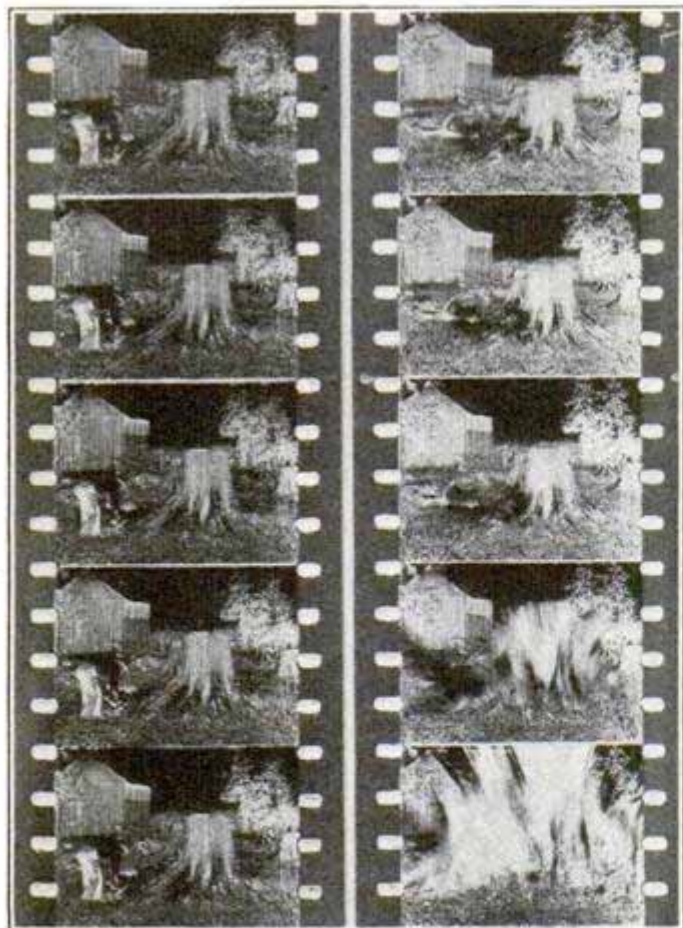
Sections of Film Showing Preparation of Charge and Blasting of Stump
