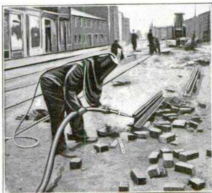
Strangely Garbed Operator of a Sand-Blast Nozzle at Work in a London Street
