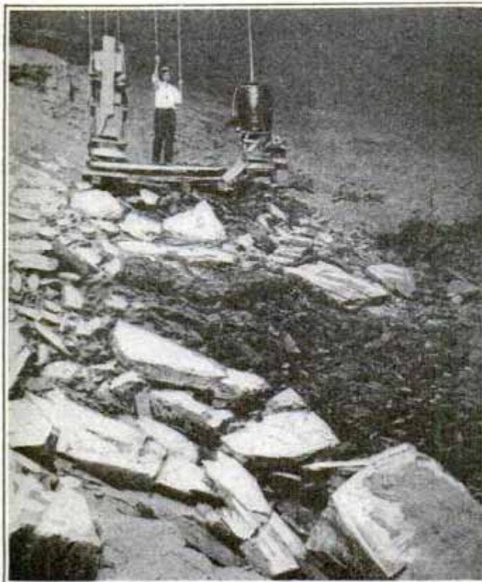
At the Bottom of the Shaft under the Ledge
