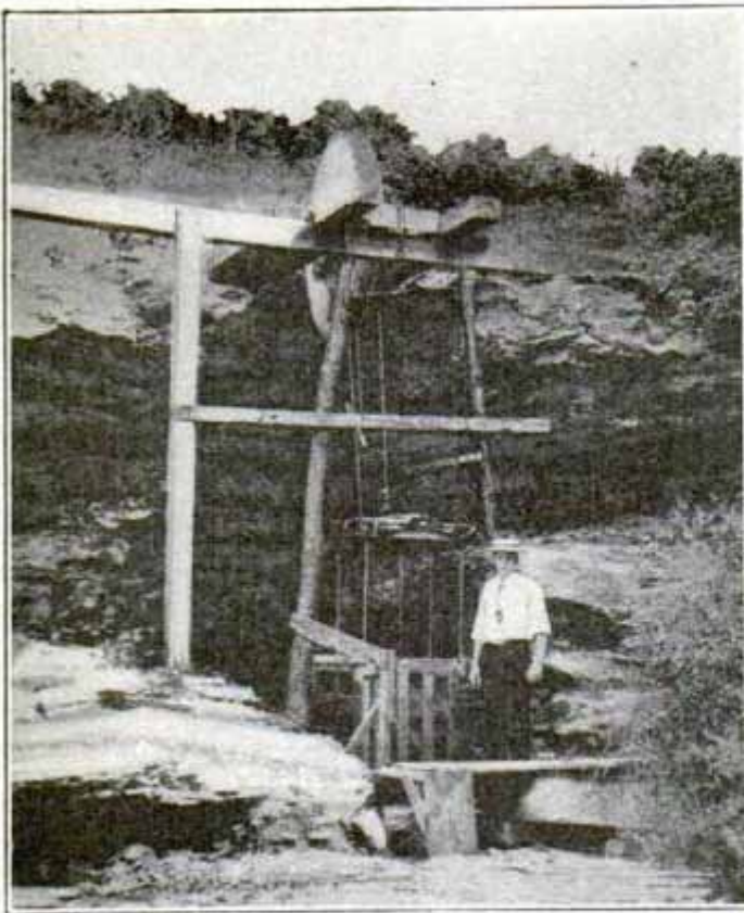
Preparing to Descend through Ledge in Unique Elevator
