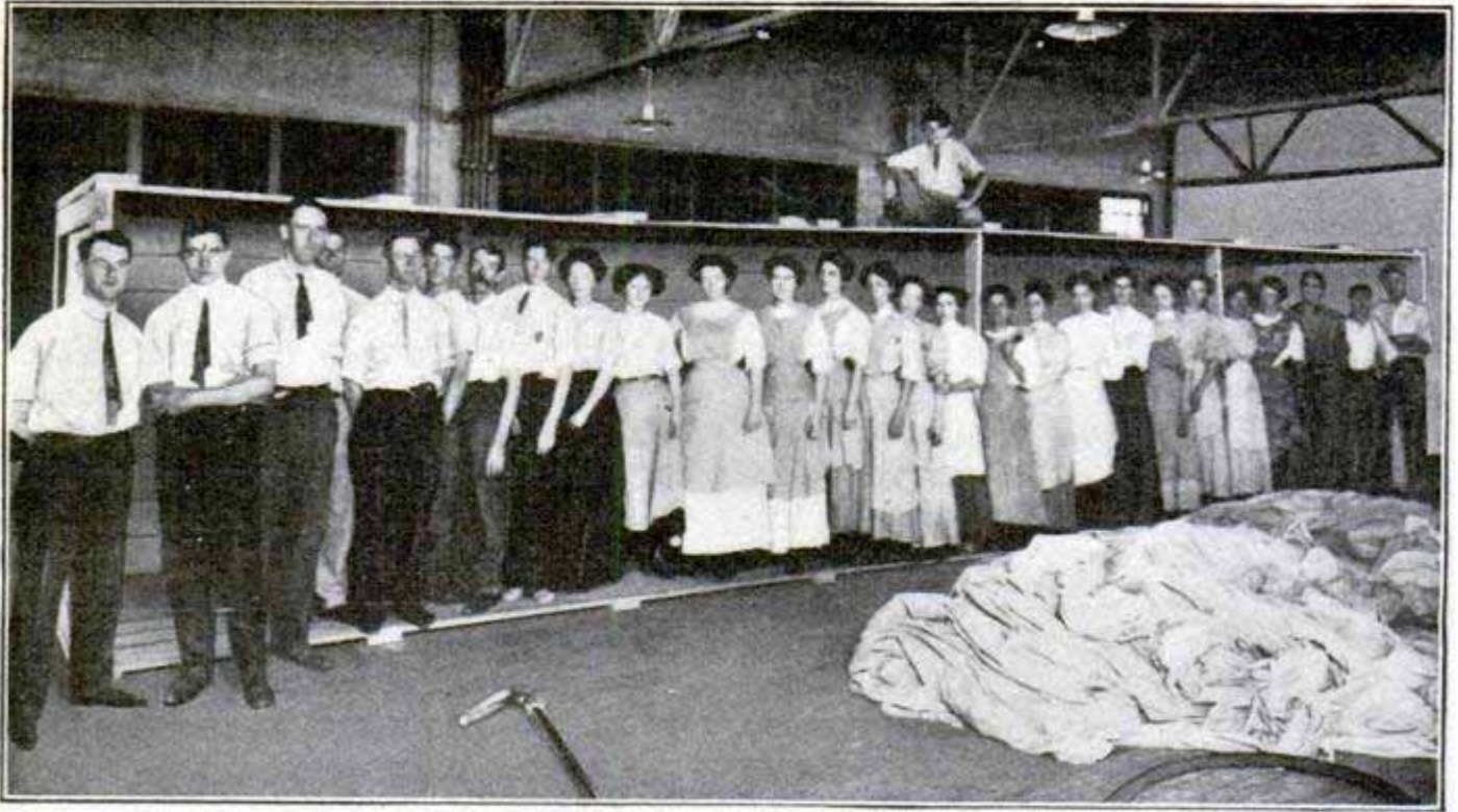
The Enormous Box in Which the Balloon Fabric was Shipped to Atlantic City—Section of Building Wall was Removed to Get the Box Out
