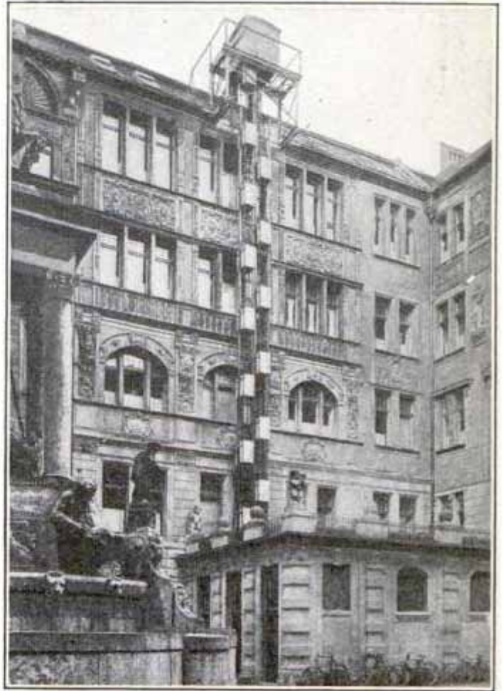
Exterior Freight Elevator on an Apartment House in Berlin
