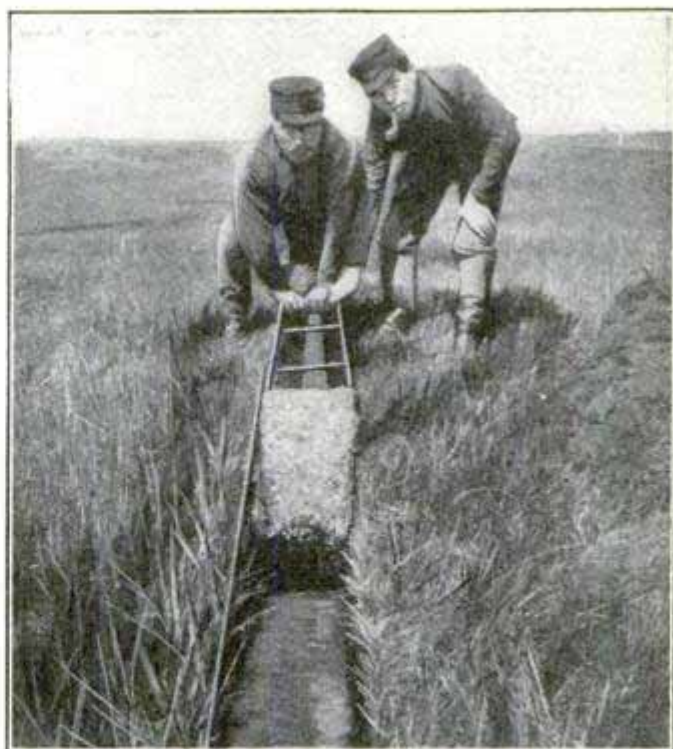
Another Spade at Work Cutting Ditches to Drain Mosquito Infested Sections. Two Men Can Dig about 600 Ft. a Day
