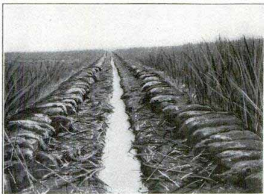
A Double-Width Main Ditch, Nearly a Mile Long, on Salt Marsh
