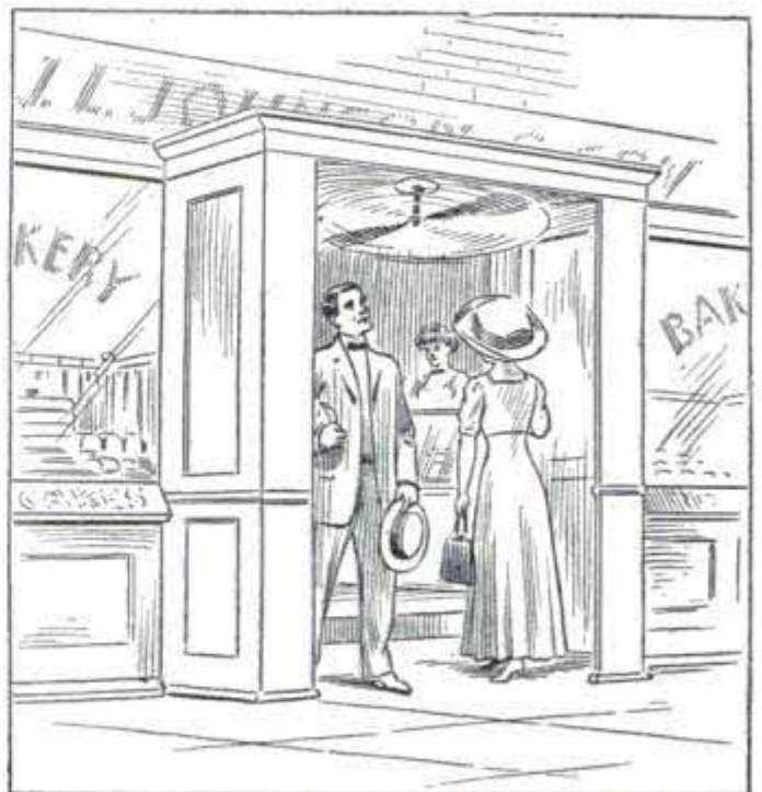
Fan above Door Makes Barrier of Air against Flies
