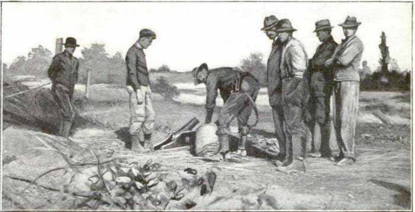
Stringing a Telephone Cable across a River with a Life-Saver's Outfit
