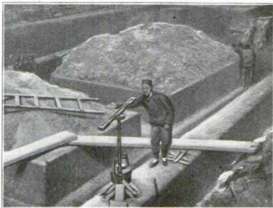
Chinese Contractor Using a Primitive but Effective Level
