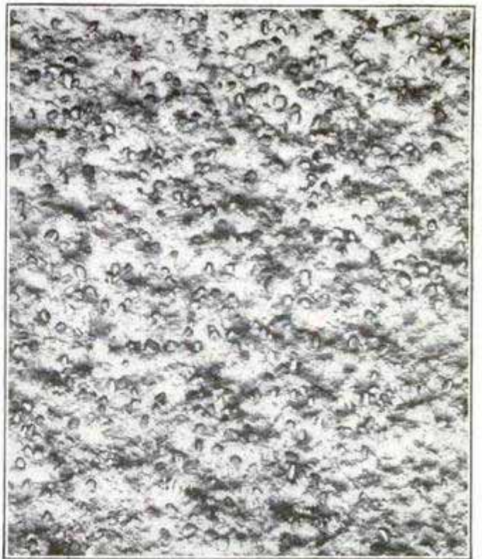
Rough Pebble-Dash Work as Done by the Roughcasting Machine.
