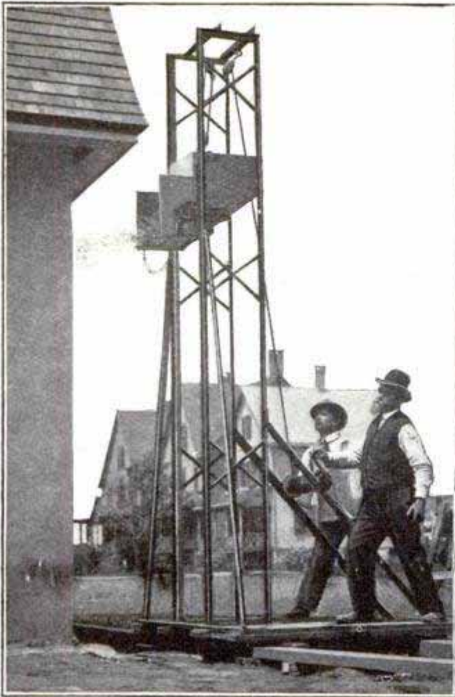
The Roughcasting Machine in Action, Throwing Material against Wall
