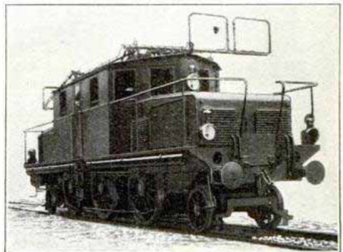
Electric Locomotive Used in Connection with the Work
