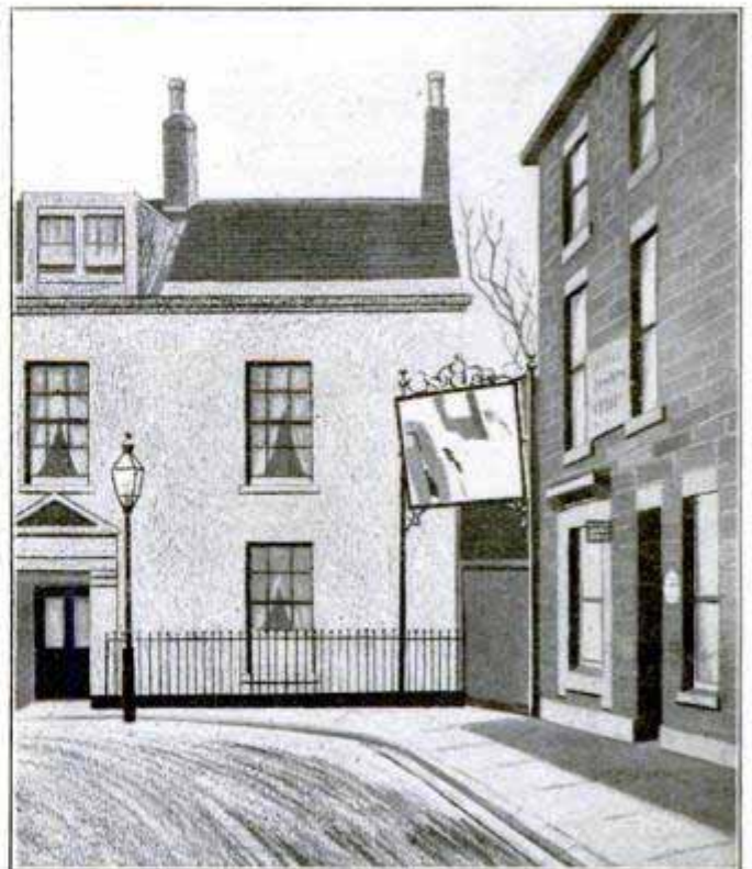
Exceptionally Large Looking Glass Mounted at Abrupt Turn in England
